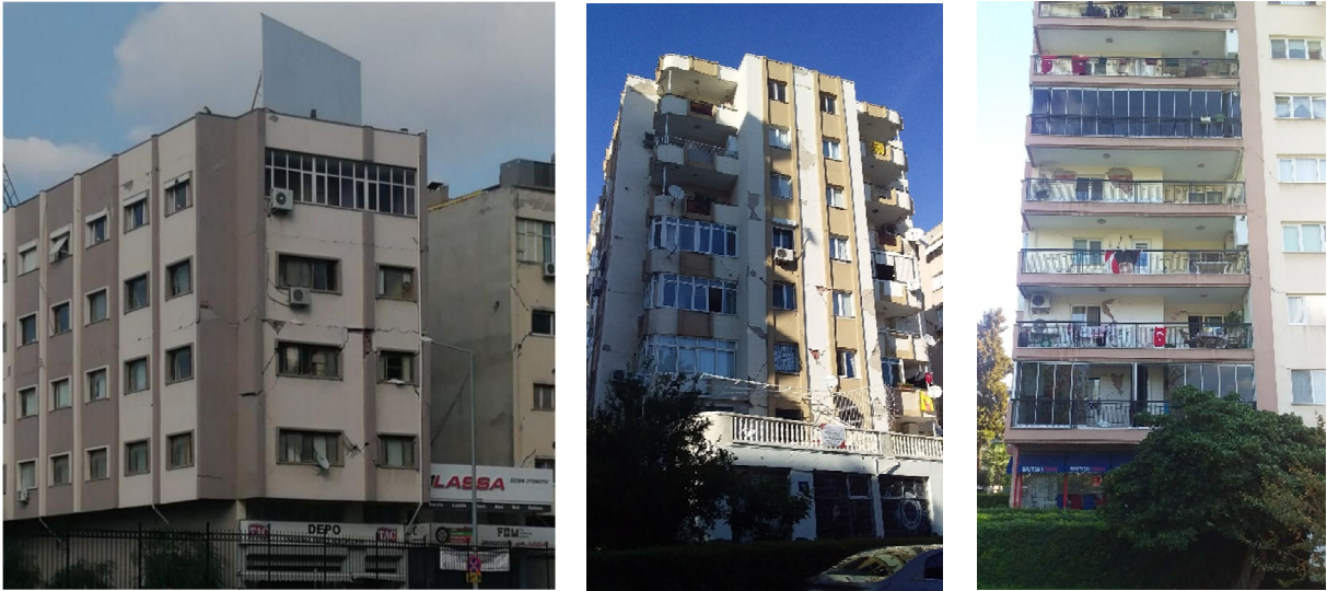
Figure 20. Damage in building façades (CNNTurk, 2020).
