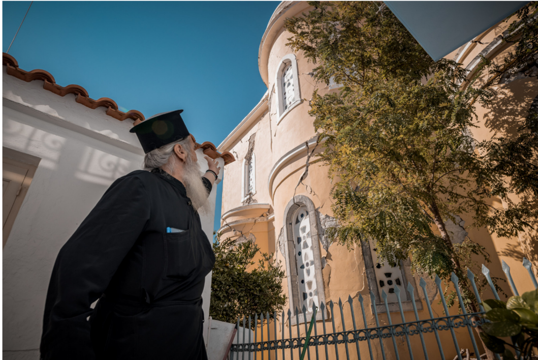
Figure 26. Damage to the Orthodox Church of Agios Nikolaos in Kokkari on the Greek island of Samos (MSN, 2020).
