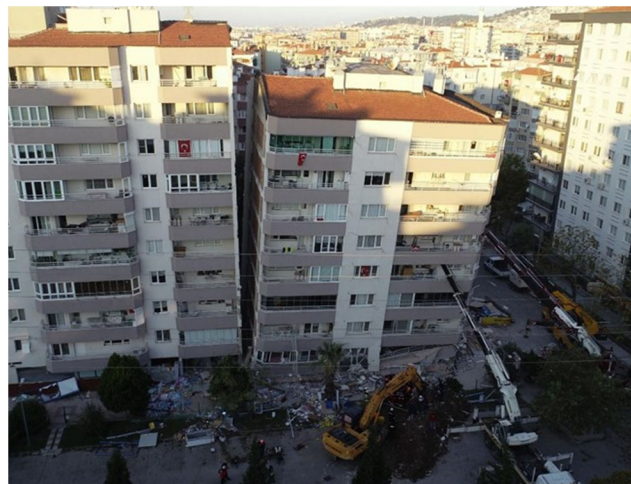
Figure 19. A partially collapsed building in Bayrakli district of Izmir, where first three floors above the ground collapsed (Twitter, 2020b; Haber7, 2020; Fanatik, 2020).
