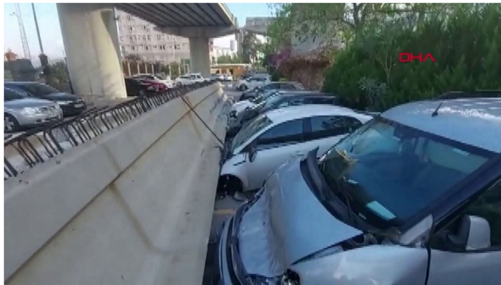
Figure 31. A collapsed girder of a bridge under construction fell to the ground and crushed parked cars in Alsancak district of Izmir, Turkey (HaberTurk, 2020).
