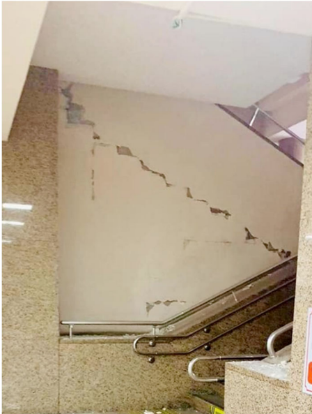
Figure 23. Nonstructural damage observed in windows, exterior and interior infill walls, and staircases of the Courthouse in Izmir (Yurt Gazetesi, 2020).
