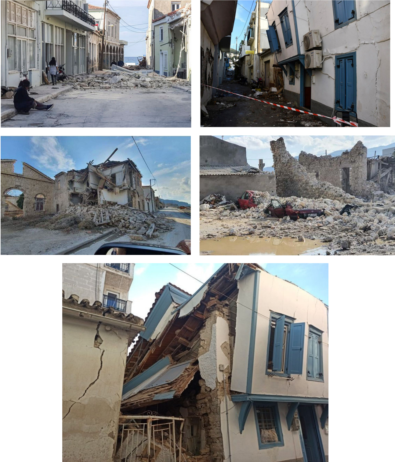
Figure 21. Damage to masonry and adobe houses on Samos island, Greece (CNN, 2020).
