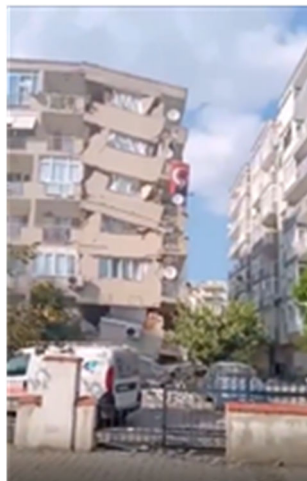
Figure 18. Partially collapsed Karagul building in Manavkuyu area, Bayrakli district, Izmir (Hurriyet, 2020).
