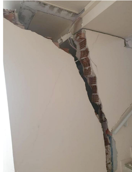
Figure 23. Nonstructural damage observed in windows, exterior and interior infill walls, and staircases of the Courthouse in Izmir (Yurt Gazetesi, 2020).
