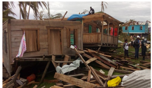
Figure 3.4. Damage to elevated wood-frame residential structures in the coastal community of Miskito, Nicaragua due to wind and storm surge impacts: (a-b) displaced boats and debris fields indicative of storm surge; (c-d) typical wind damage to CGI roofs; (e) houses unseated from foundation (Sources: Palmado via Twitter and Paul Cruz via Twitter ).
