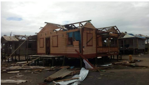
Figure 3.4. Damage to elevated wood-frame residential structures in the coastal community of Miskito, Nicaragua due to wind and storm surge impacts: (a-b) displaced boats and debris fields indicative of storm surge; (c-d) typical wind damage to CGI roofs; (e) houses unseated from foundation (Sources: Palmado via Twitter and Paul Cruz via Twitter ).
