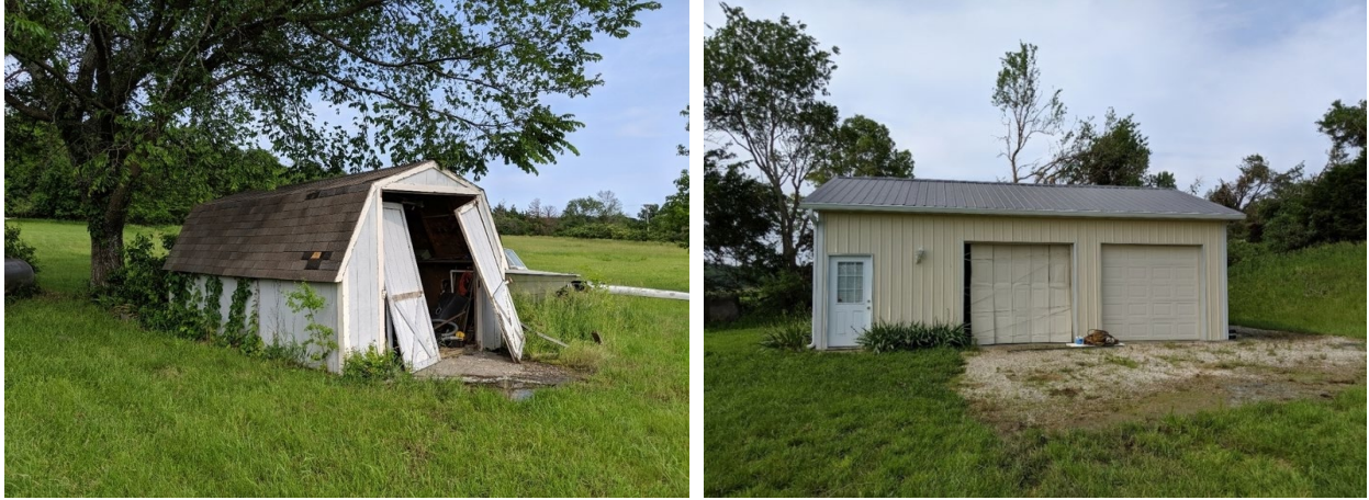
Figure 24. Damaged shed door (left) and garage door (right).
