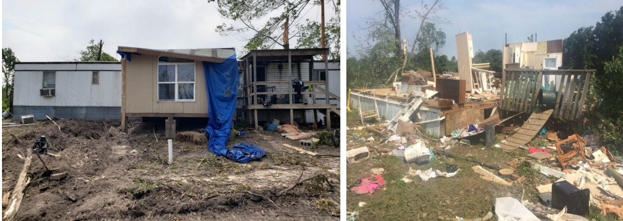
Figure 20. Severely damaged manufactured home (left) and completed destroyed manufactured home (right).
