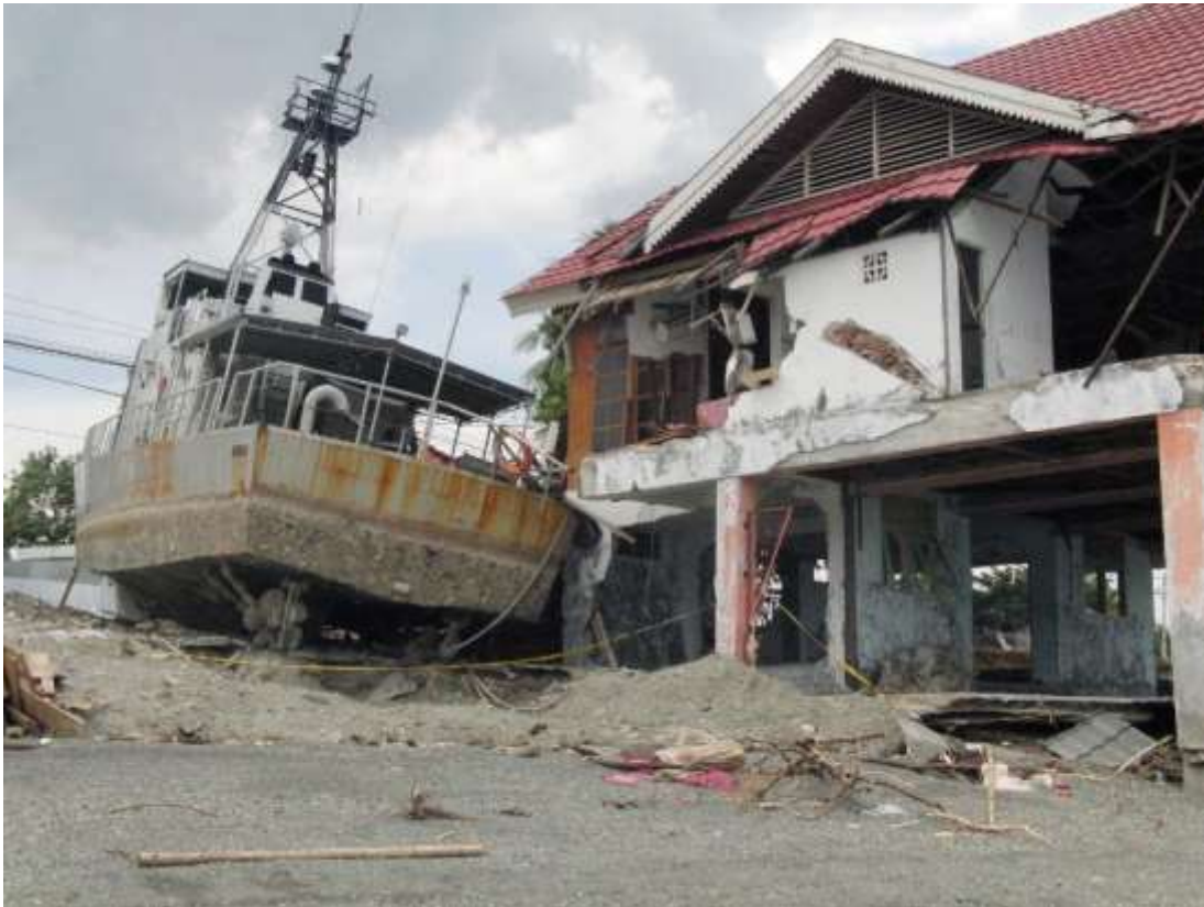
Figure 71: Naval ship adjacent to building with evidence of impact damage.
