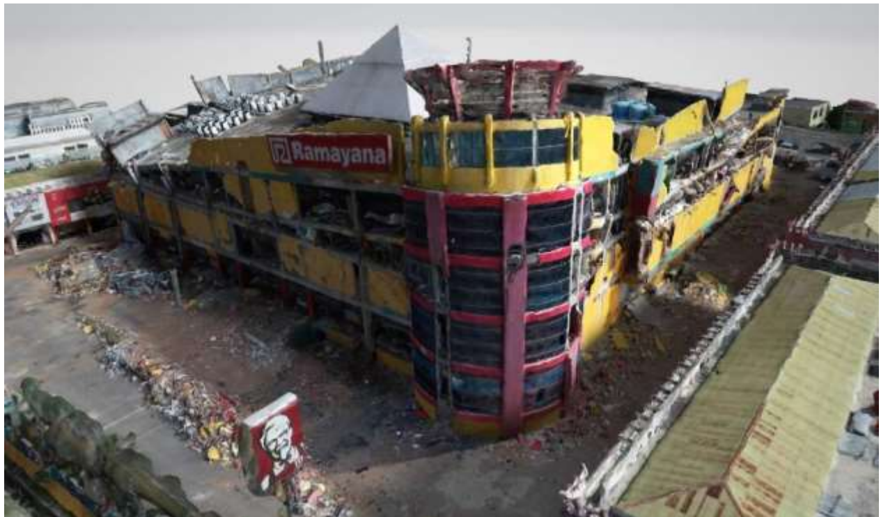
Figure 47: 3D image of Tatura Shopping Mall generated from 1500 drone images using “Structure-from-Motion”
