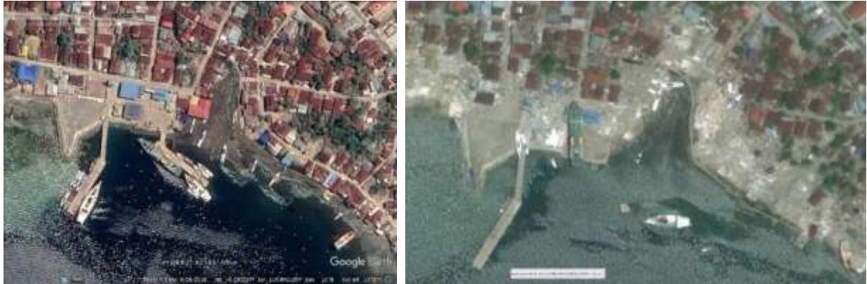
Figure 74: Google Earth images of Wani Port before (left) and after (right) earthquake and tsunami.
