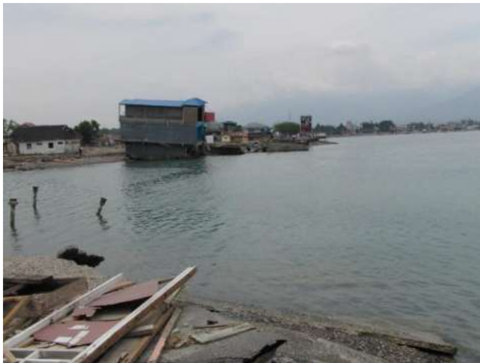
Figure 22: View along original alignment of coastal highway (See Figure 21) that is suspected to have been part of landslide 11 in Talise.
