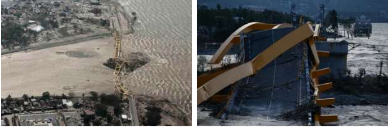
Figure 64: Palu Bridge IV after the earthquake and tsunami.
