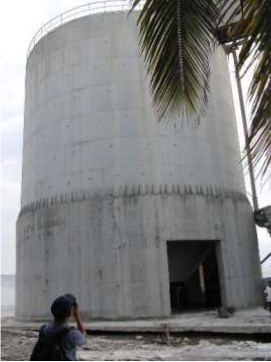
Figure 79: Leaning cement silo (left) and scour under surrounding concrete apron (right).
