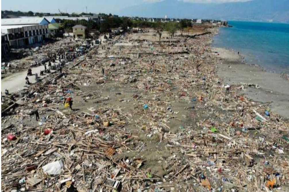
Figure 33: Debris from light framed timber structures along the Palu shoreline (Credit: Jewel Samad/AFP).
