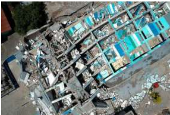
Figure 43: Google Earth Streetview images of Roa-Roa Hotel before the earthquake (top) and collapsed Roa-Roa Hotel after the earthquake (bottom).
