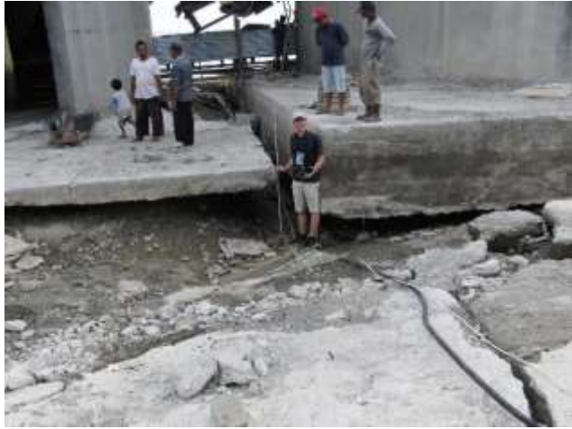
Figure 79: Leaning cement silo (left) and scour under surrounding concrete apron (right).
