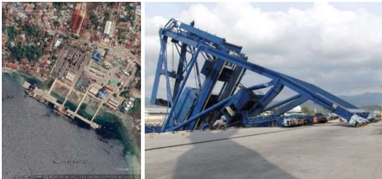
Figure 73: Google Earth image of the Port of Pantoloan before the earthquake and tsunami (left) and the collapsed gantry crane after the earthquake (right).
