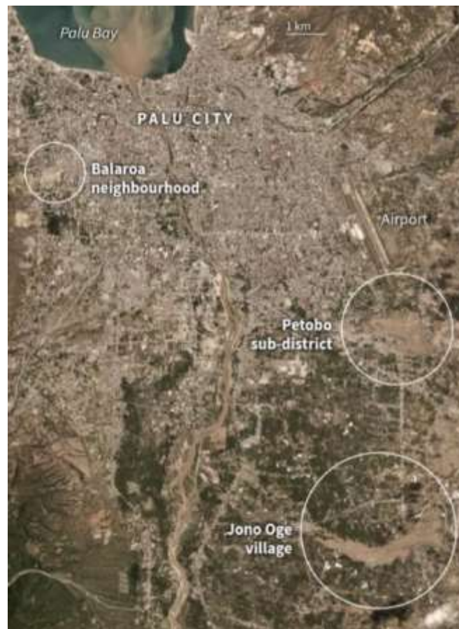
Figure 35: Areas of significant liquefaction induced lateral spreading in and around Palu City.
