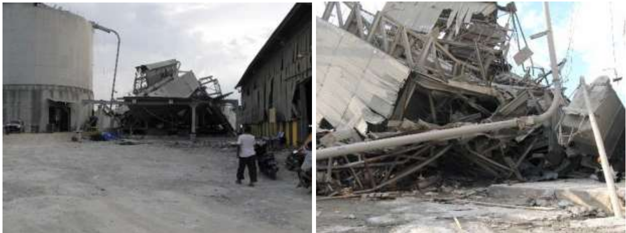
Figure 78: Collapse of steel-framed cement packaging building during earthquake.
