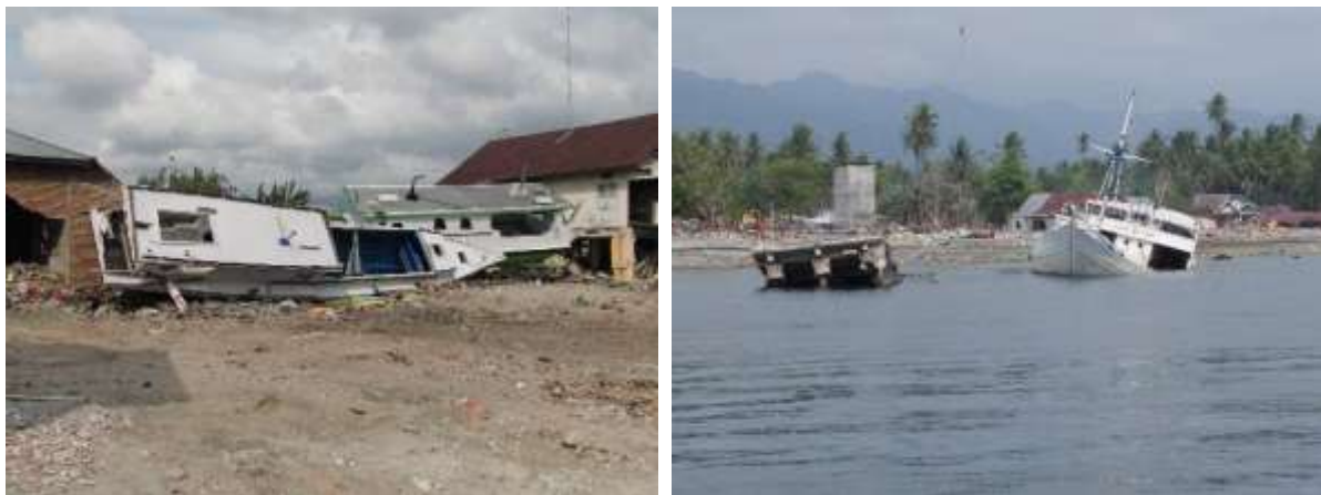
Figure 76: Ship impact with buildings (left) and broken pier and sunken ship (right) at Wani Port.
