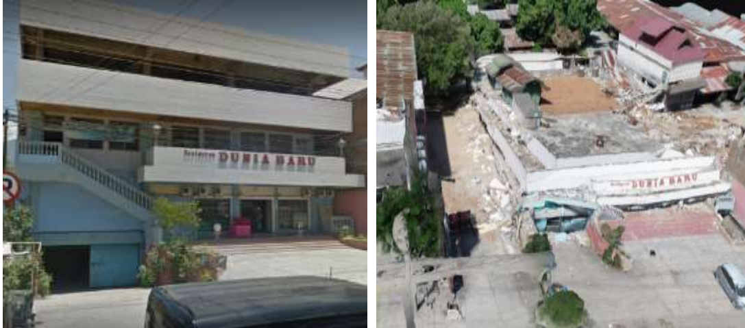
Figure 52: Dunia Baru Restaurant before the earthquake and after the earthquake
