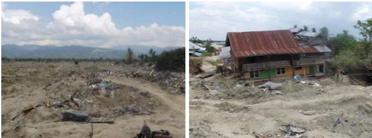
Figure 41: View looking up the Petobo Sub-district slide (left) and a typical timber framed home that traveled with the surface soil during the slide (right).
