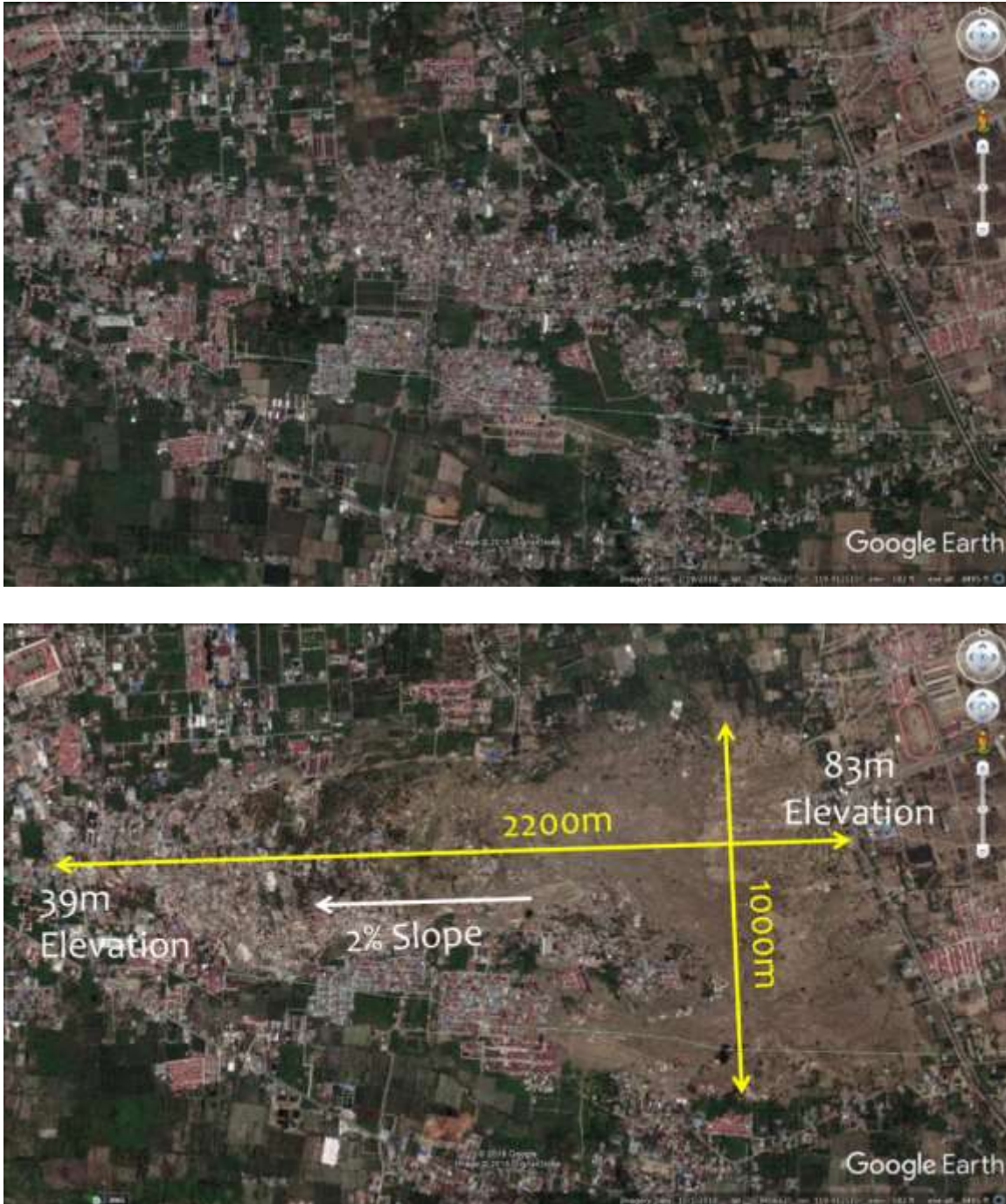
Figure 39: Google Earth image of Petobo Sub-district before earthquake (top) and after earthquake (bottom) showing extent of lateral spreading due to liquefaction.
