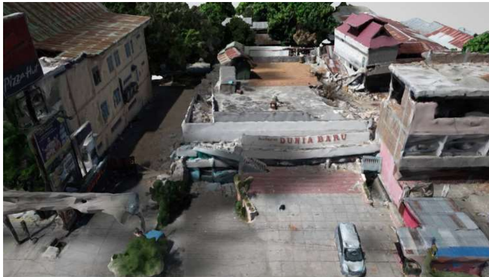
Figure 53: 3D image of Dunia Baru Restaurant generated from 577 drone images using “Structure-from-Motion”
