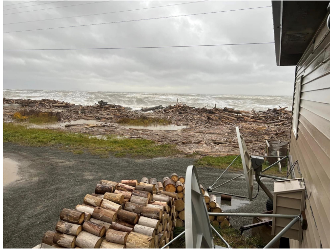
Figure 6.7: Remnants of the Shaktoolik berm (source: Bering Strait School District, Alaska DHS & EM 2022b )
