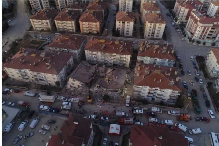
Figure 7. Collapsed reinforced concrete building in Sursuru neighborhood of Elazig with similar intact buildings around (NTV, 2020).
