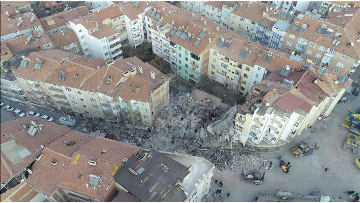
Figure 6. Collapsed reinforced concrete building among a block of buildings in Mustafa Pasa neighborhood of Elazig (Anadolu Agency, 2020).
