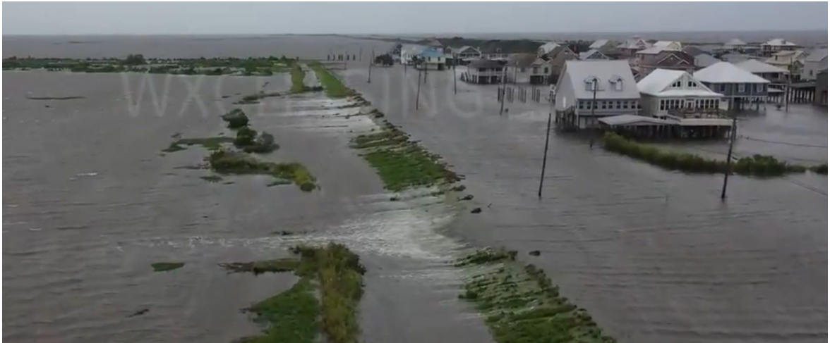
Figure 5. Levee overtopping in Plaquemines Parish near Myrtle Grove. Still shot taken from video by WXChasing .
