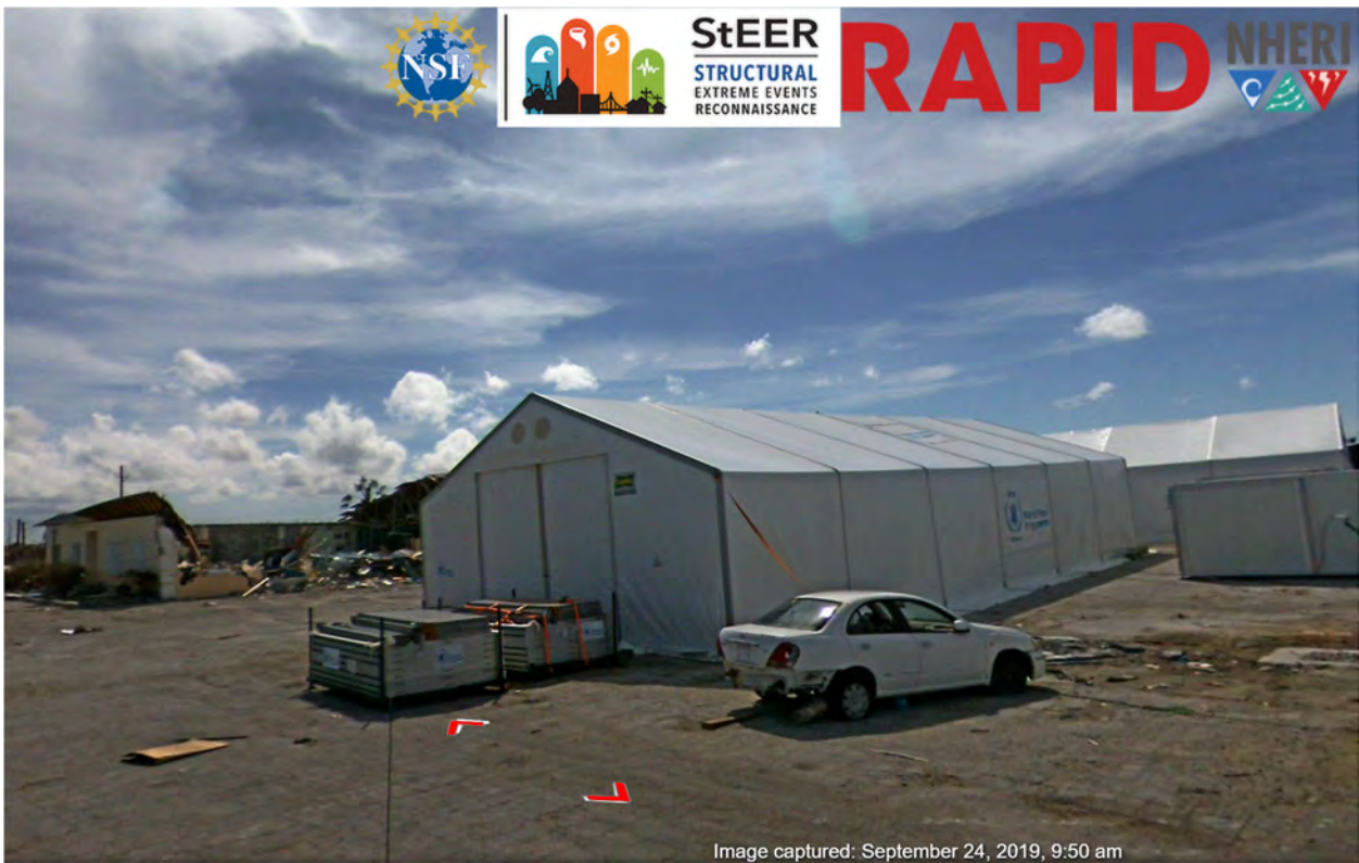
Figure 7.7. StreetView imagery of the temporary structures set up at the port facility, with view of the destroyed Administration building in the background.
