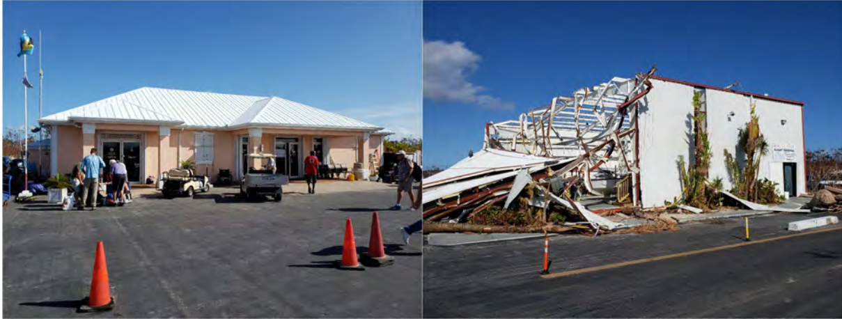
Figure 7.3. Examples of structures assessed by the D2D team at the Leonard Thompson International Airport: (a) Flight Base of Operations (FBO) Jet Center, assessed as “Undamaged” [26.51362, -77.08426]; (b) Cherokee Aviation hangar building, assessed as “Severe” damage [26.51353,-77.08483].
