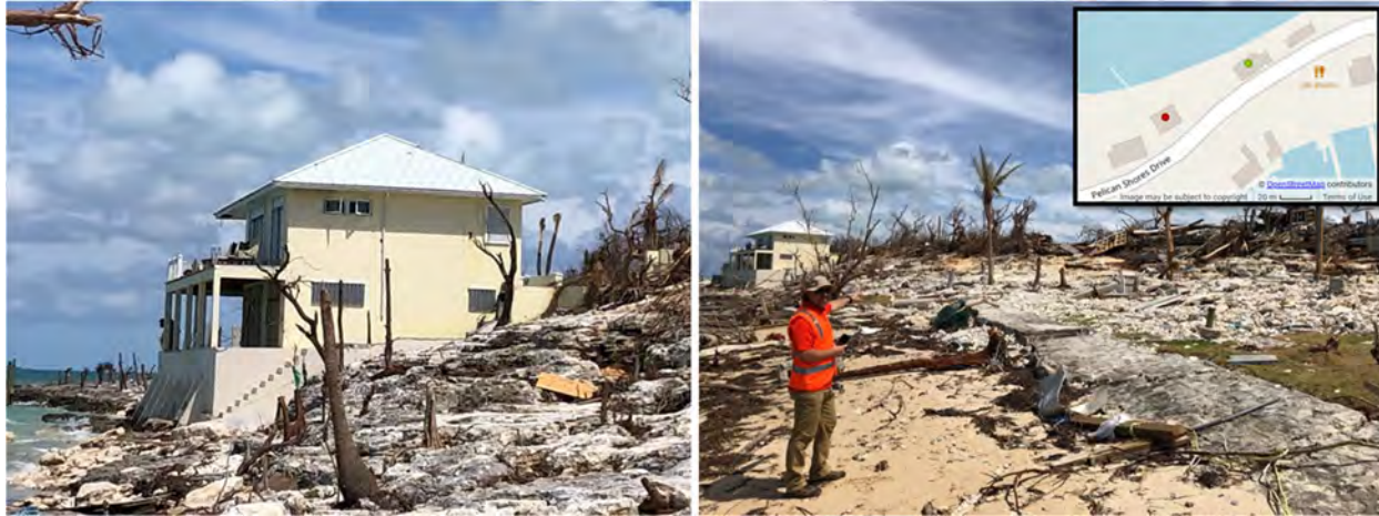
Figure 6.1. Contrast between the performance of two homes located along Pelican Shores Drive exposed to the worst of Dorian's wind, storm surge and waves. The home on the left is located at [26.552164, -77.055065], and the home on the right at [26.551852, -77.055599].
