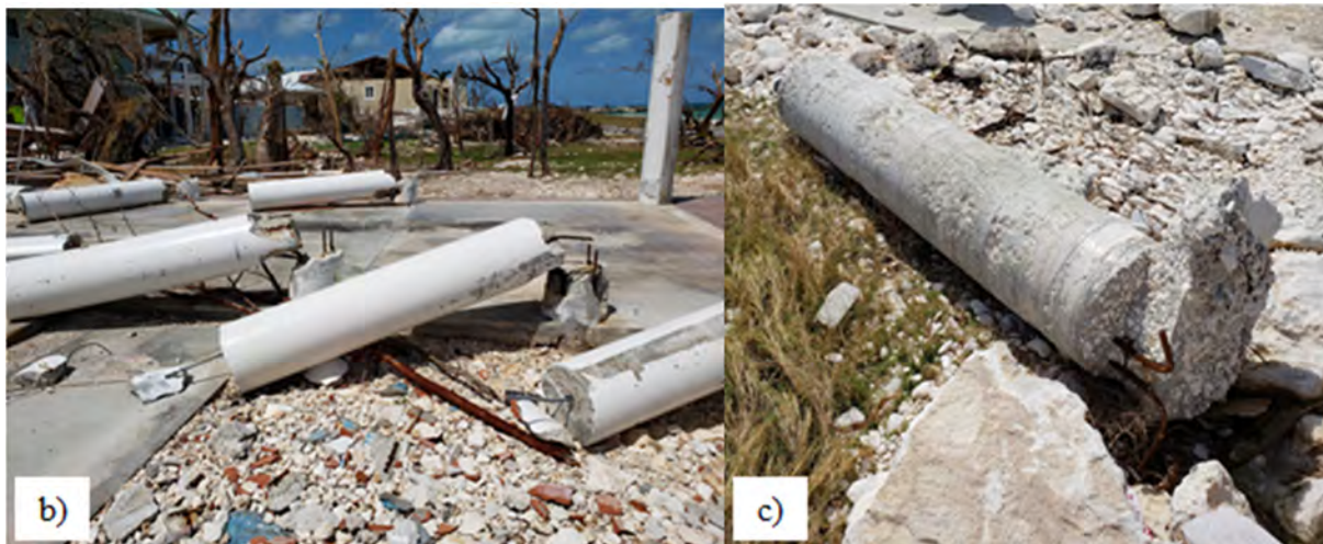
Figure 6.2. (a) Google Earth map indicating structures that collapsed due to wind and surge along the coast. The structure on the far left with a red marker is located at [26.55363, -77.06072]. (b) Topped concrete columns showing minimal corroded reinforcement and a single anchor bolt to attach to the supported structure located at [26.44297, -77.05980]. (c) Topped concrete column showing minimal reinforcing and anchorage into a footing located at [26.55174, -77.05588].
