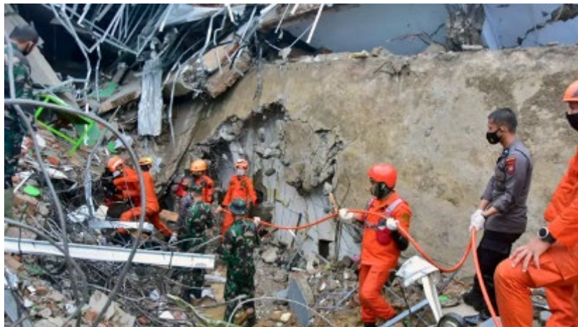
Figure 3.7 A collapsed government building in Mamuju (Source: AP Photo/Daus Thobelulu).
