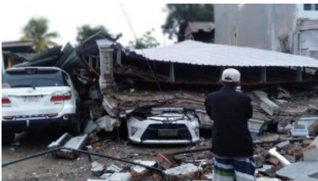
Figure 3.2 Images of collapsed RC residential buildings and one with a failed exterior wall (lower right) located in Mamuju (Sources: CNN 2021b, GettyImages 2021, AP 2021, AP Photo/Rudy Akdyaksyah, Kumparan, 2021, https://pbs.twimg.com/media/Er1PSQuU0AIPcnw.jpg ).
