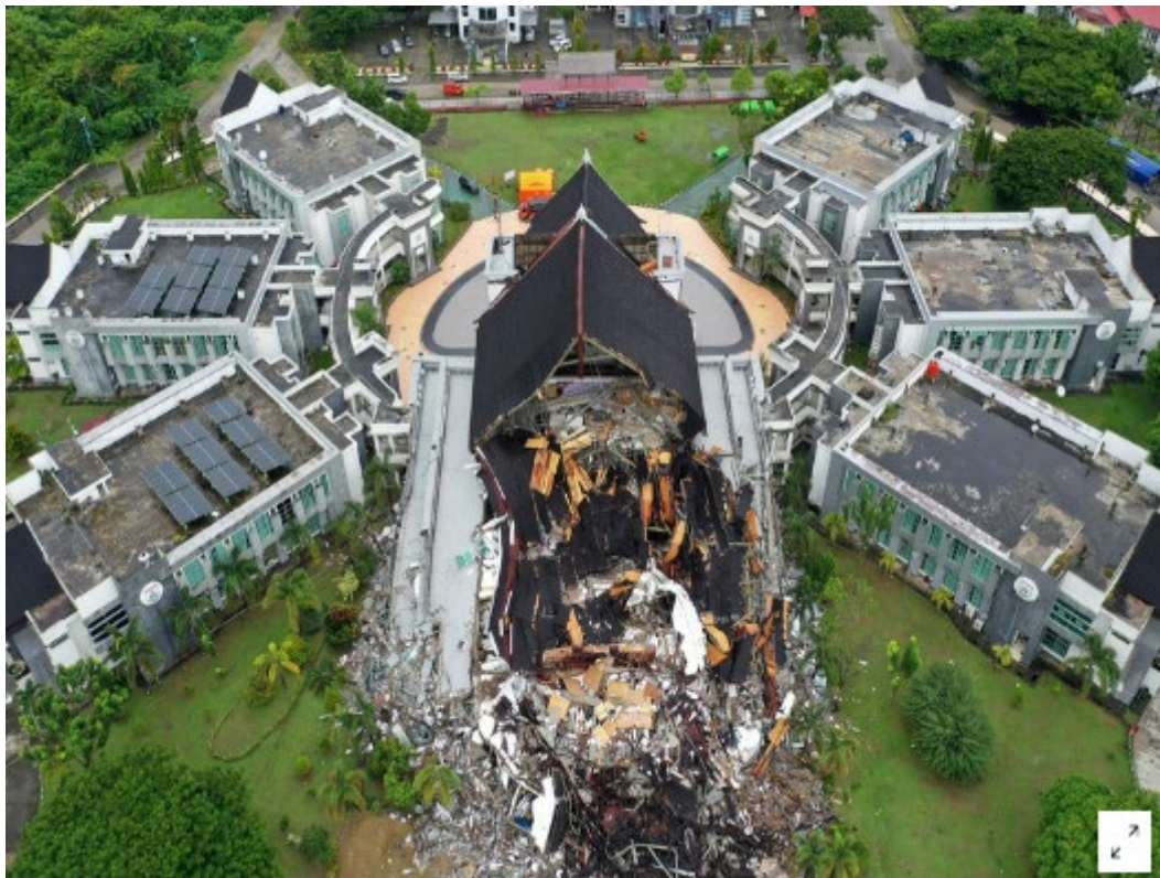
Partially collapsed West Sulawesi Governor's office in Mamuju, Sulawesi, Indonesia
