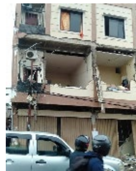
Figure 3.2 Images of collapsed RC residential buildings and one with a failed exterior wall (lower right) located in Mamuju (Sources: CNN 2021b, GettyImages 2021, AP 2021, AP Photo/Rudy Akdyaksyah, Kumparan, 2021, https://pbs.twimg.com/media/Er1PSQuU0AIPcnw.jpg ).
