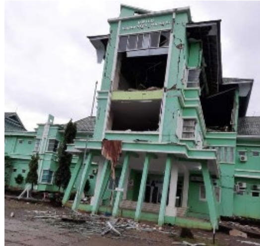
Figure 3.5 Glass façade and unreinforced masonry walls of a district hospital in Mamuju (2.685S, 118.889E) intact before the earthquake (left) and broken after the earthquake (right) (Sources: Left: Google Street view; Right: https://suryakepri.com/2021/01/16/update-jumlah-korban-gempa-majene-bertambah-jadi-42-orang-meninggal-dunia/ ).
