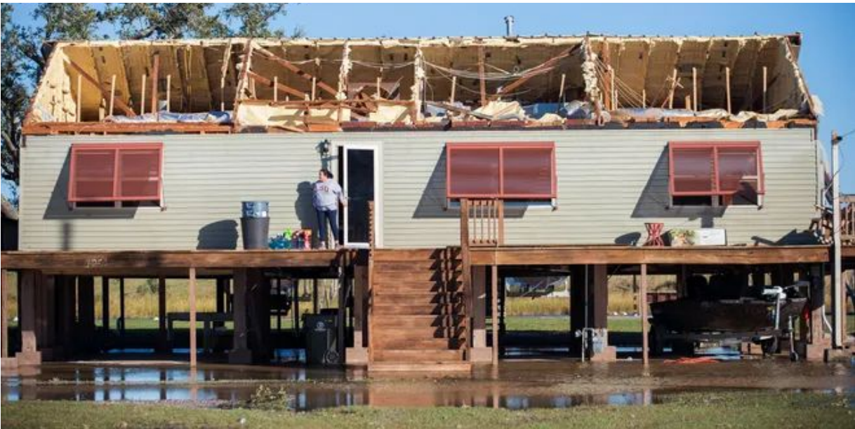
Figure 3.1.1. Roof damages in Louisiana: (a) loss of metal roof cover on a commercial building (upper left background) and roof sheathing loss and damage to wood roof trusses in elevated homes (foreground) in Grand Isle, LA (Source: BRproud.com ); (b) complete detachment of roof section in gable roof home in Chauvin, LA (Source: Chris Granger, AP via USA Today )
