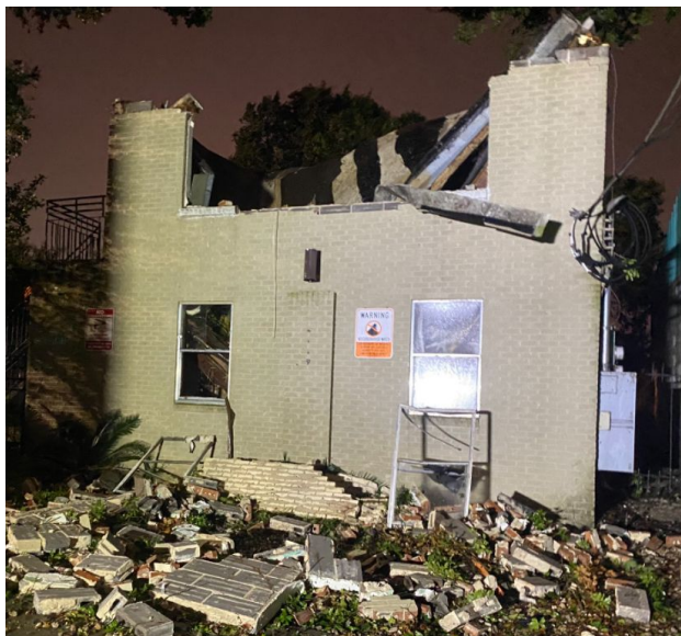
Figure 3.1.3. Masonry failures in Hurricane Zeta: roof failure propagating to the collapse of second-story unreinforced masonry walls (a) of a commercial building in Golden Meadow, LA (Source: Twitter ) and (b) in an apartment in New Orleans, LA (Source: NYtimes ); (c) loss of brick veneer at apartment building in New Orleans suburb of Terrytown (Image credit: Jefferson Parish ).
