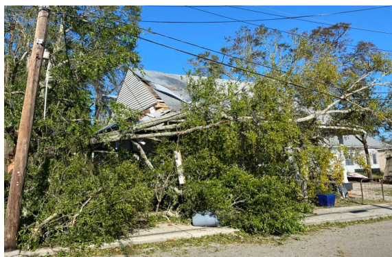
Figure 3.1.6. Examples of roof damage to homes in Waveland, MS, ranging from (a-b) loss of cover and sheathing to (c) additional loss of framing (Source: Twitter ); (d) tree falls were also a driver of damage to roofs in areas like Bay St. Louis, MS (Source: Twitter )
