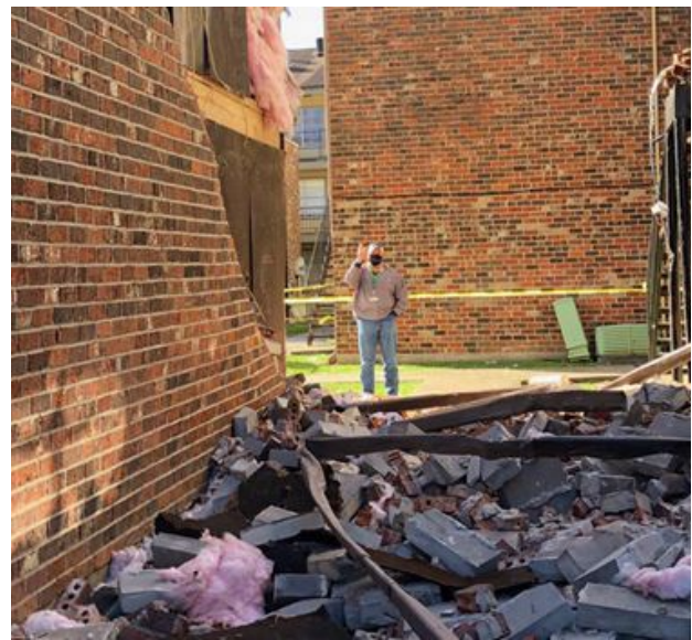
Figure 3.1.3. Masonry failures in Hurricane Zeta: roof failure propagating to the collapse of second-story unreinforced masonry walls (a) of a commercial building in Golden Meadow, LA (Source: Twitter ) and (b) in an apartment in New Orleans, LA (Source: NYtimes ); (c) loss of brick veneer at apartment building in New Orleans suburb of Terrytown (Image credit: Jefferson Parish ).
