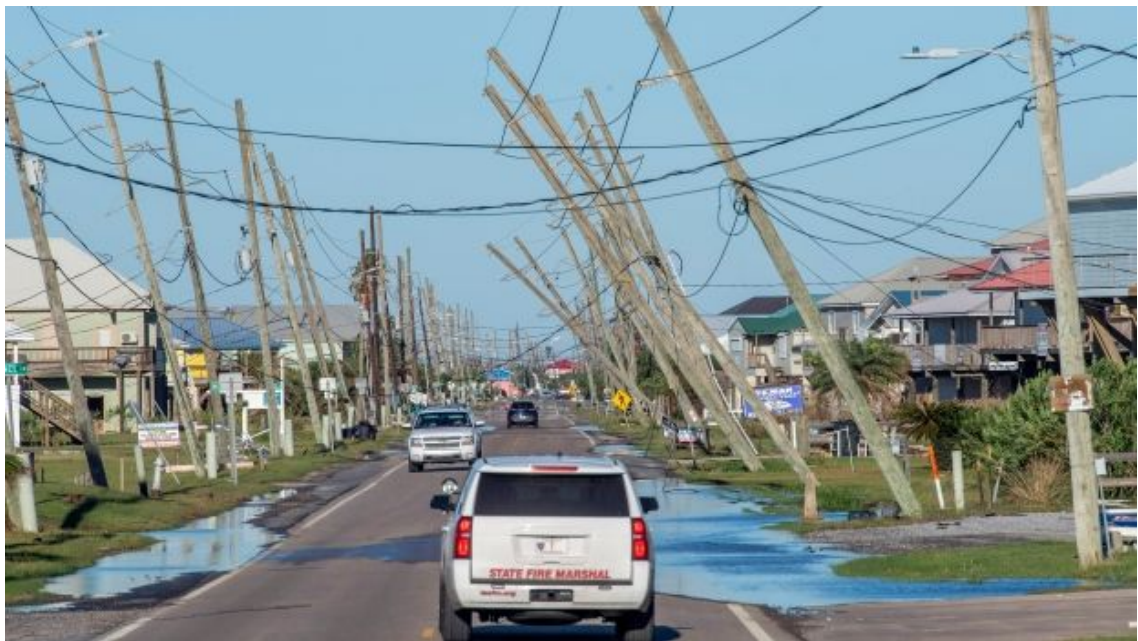
Figure 3.2.2. Power poles leaning or snapped due to Hurricane Zeta in: (a)-(b) Yucatan Peninsula (Source: Riviera-Maya-News ) and (b) Grand Isle, LA (Source: CP24 )
