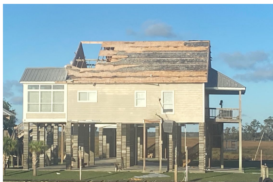
Figure 3.1.6. Examples of roof damage to homes in Waveland, MS, ranging from (a-b) loss of cover and sheathing to (c) additional loss of framing (Source: Twitter ); (d) tree falls were also a driver of damage to roofs in areas like Bay St. Louis, MS (Source: Twitter )
