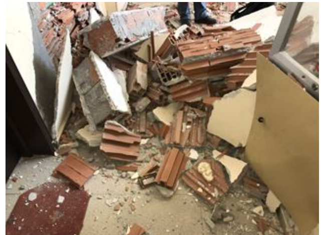
Figure 5. Heavily damaged multicell clay blocks in masonry buildings and infill walls in RC buildings (Twitter, 2019)
