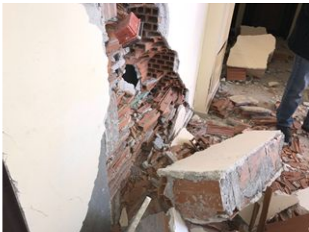
Figure 5. Heavily damaged multicell clay blocks in masonry buildings and infill walls in RC buildings (Twitter, 2019)
