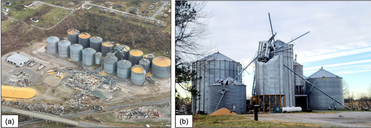
Figure 7.3.1. (a) Aerial view of damage to grain silos ( NAPSG Crowdsourcing ) (Lat: 36.7339, Long: -88.6477) and (b) damage caused by grain elevator collapse ( NAPSG Crowdsourcing ) in Fulton County.
