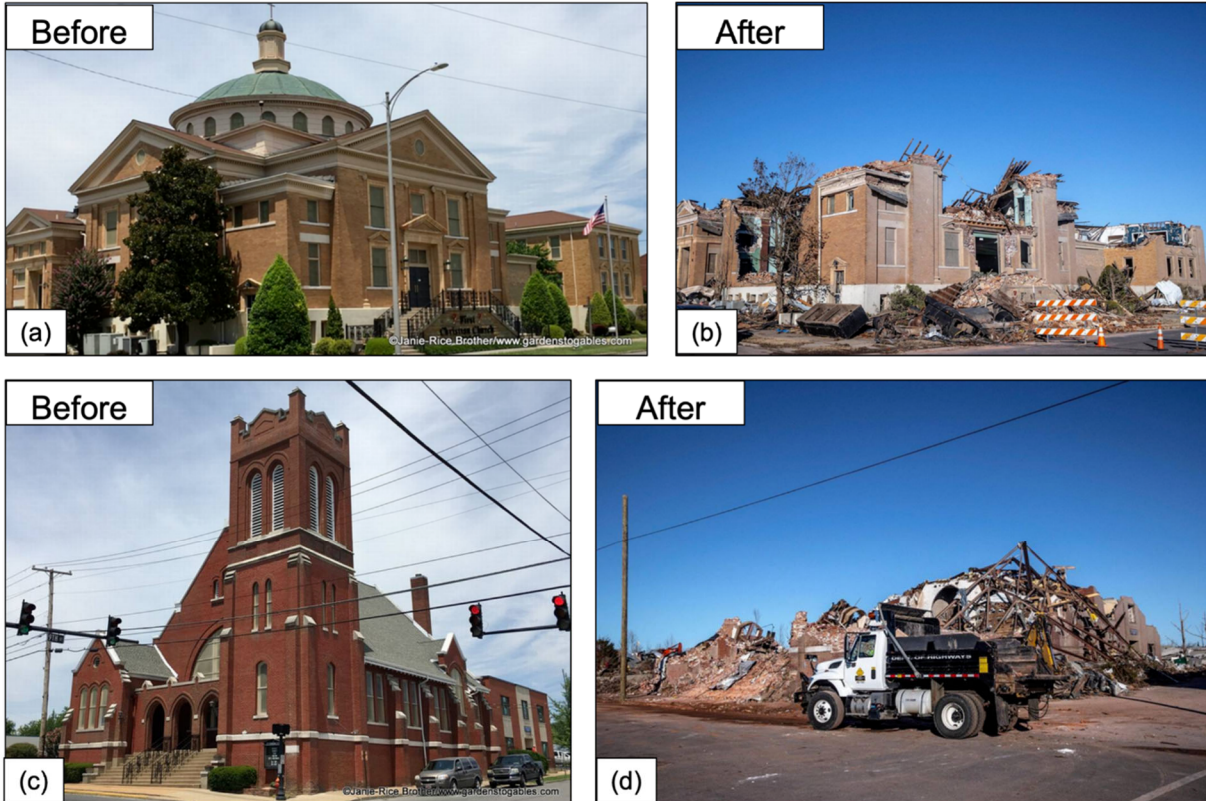
Figure 6.5.1. Damage to churches in Mayfield: (a) First Christian Church on South 9th Street (Lat: 36.74086, Long: -88.6389) before and (b) after tornado, and (c) historic First Presbyterian Church (Lat: 36.7420, Long: -88.6389) on West Broadway before and (d) after tornado (source: Kentucky.com ).
