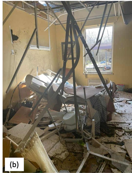
Figure 6.4.7. A closer view of damage to the Mayfield Health and Rehabilitation Center: (a) loss of roof and exterior CMU wall with brick cladding, and (b) falling roof ceiling panels and other debris. (Sources: (a) acquired by the FAST, (b) from Mayfield Health and Rehabilitation Center Facebook page ).
