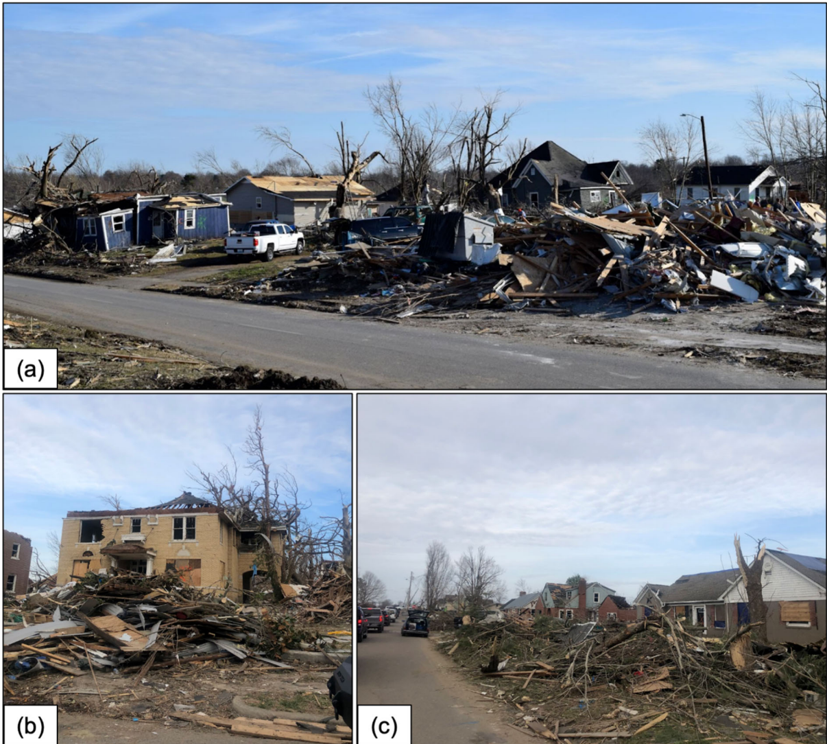
Figure 6.1.3. Representative residential damage and debris found in Mayfield, KY, including (a) varying damage levels, from no visible damage to complete collapse, evident in a cluster of wood-frame homes in close proximity to each other; (b) loss of the roof structure and windows blown out in a two-story home with a large pile of debris in front of it; and (c) debris piles in front a row of homes that suffered primarily building envelope damage. (Images acquired by the FAST).
