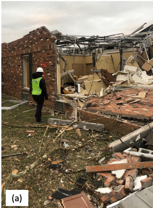
Figure 6.4.7. A closer view of damage to the Mayfield Health and Rehabilitation Center: (a) loss of roof and exterior CMU wall with brick cladding, and (b) falling roof ceiling panels and other debris. (Sources: (a) acquired by the FAST, (b) from Mayfield Health and Rehabilitation Center Facebook page ).
