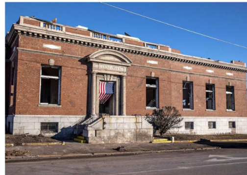
Figure 6.3.2. Before and after images of the Post Office (Lat: 36.741, Long: -88.6383) on West Broadway in Mayfield (source: Lexington Herald Leader ). Note complete loss of all visible fenestration.
