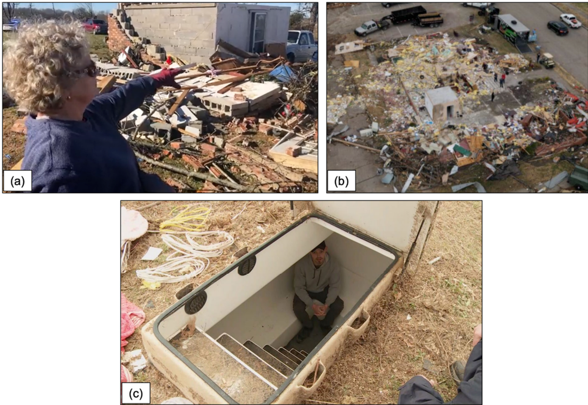
Figure 6.6.1. (a) Homeowner shows surviving home-built “safe room” at 44 Perry Lane, Bremen, KY (Lat: 37.3729, Long: -87.2200) after the 10 December Tornado outbreak. This safe room was constructed after a tornado destroyed this same home in 1988 (source: Twitter ), (b) a safe room in Hargrove & Foster, an attorneys’ office building at Mayfield, KY (Lat: 36.7429, -88.6347) (source: FAST UAV ), and (c) a pre-fab underground shelter, which safely housed 8 people and 2 dogs during the tornado at Berman, KY (exact location unknown) (source: WHAS11 News ).
