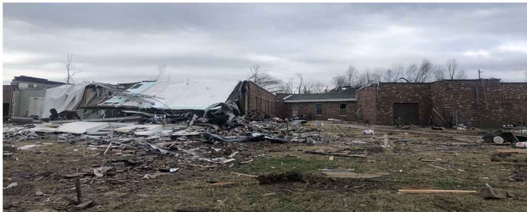
Figure 6.4.6. Damage to one wing of the Mayfield Health and Rehabilitation Center (Image acquired by the FAST).
