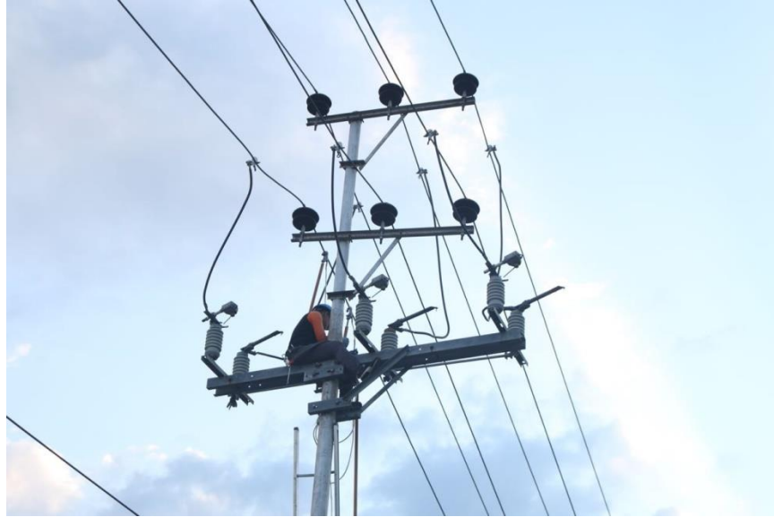
Figure 38: Repair of high-voltage transmission lines within days after the earthquake.
