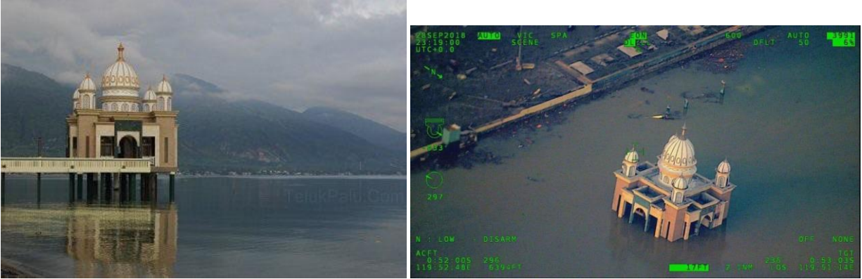
Figure 19: Apung Palu Mosque before (left) and after (right) the earthquake and tsunami. Exact cause of damage not yet established but could be due to earthquake shaking prior to the tsunami, or possibly a combination of both events.
