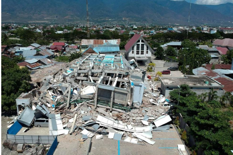
Collapsed Roa-Roa Hotel in Palu
