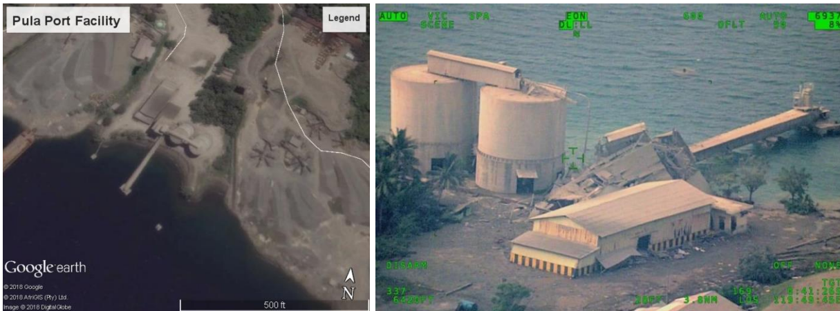
Figure 28: Damage to port facility (0.690718 S, 119.82923 E)
