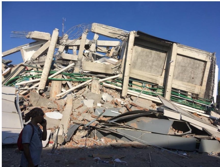
Figure 14: Lower levels of Roa-Roa Hotel after collapse due to earthquake
