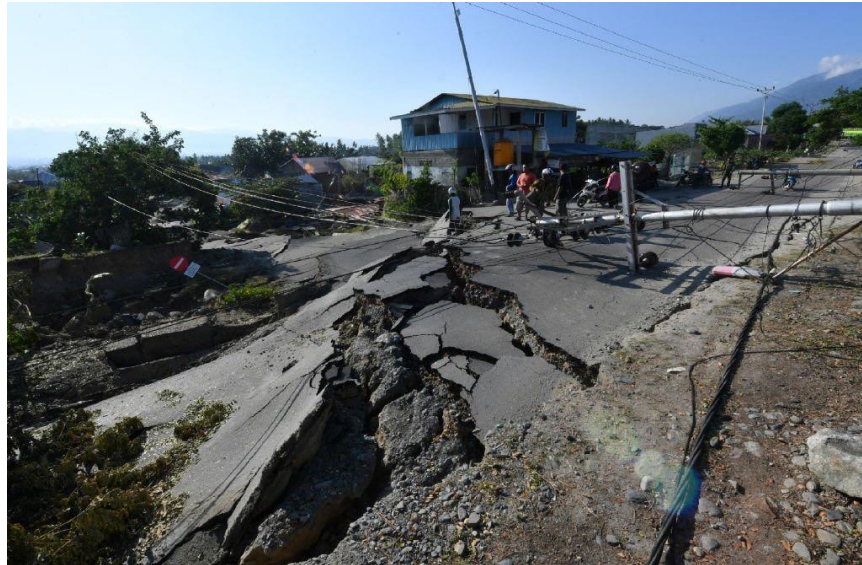
Figure 29: Significant damage to roadways due to fault rupture and liquefaction.
