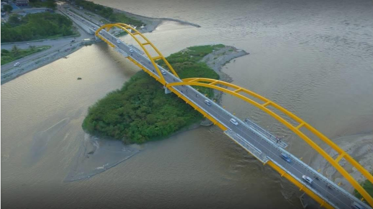
Figure 23: Palu Bridge IV prior to earthquake (Tofan Rozianto) (0.885423 S, 119.85883 E)
