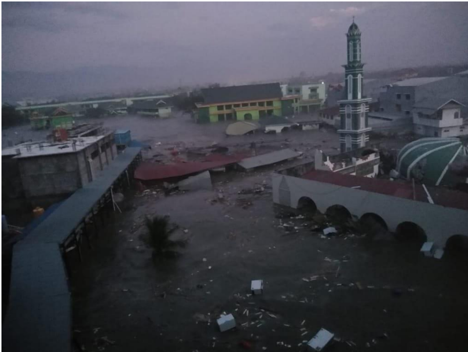
Figure 18: Baiturrahman Mosque during tsunami inundation
