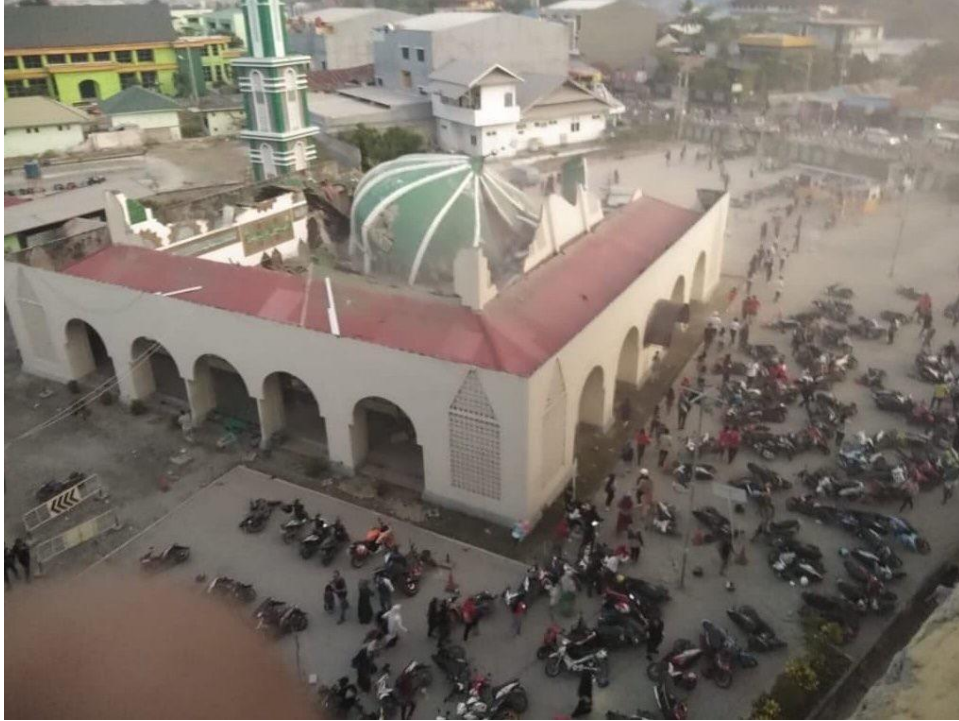
Figure 17: Damage to Baiturrahman Mosque
