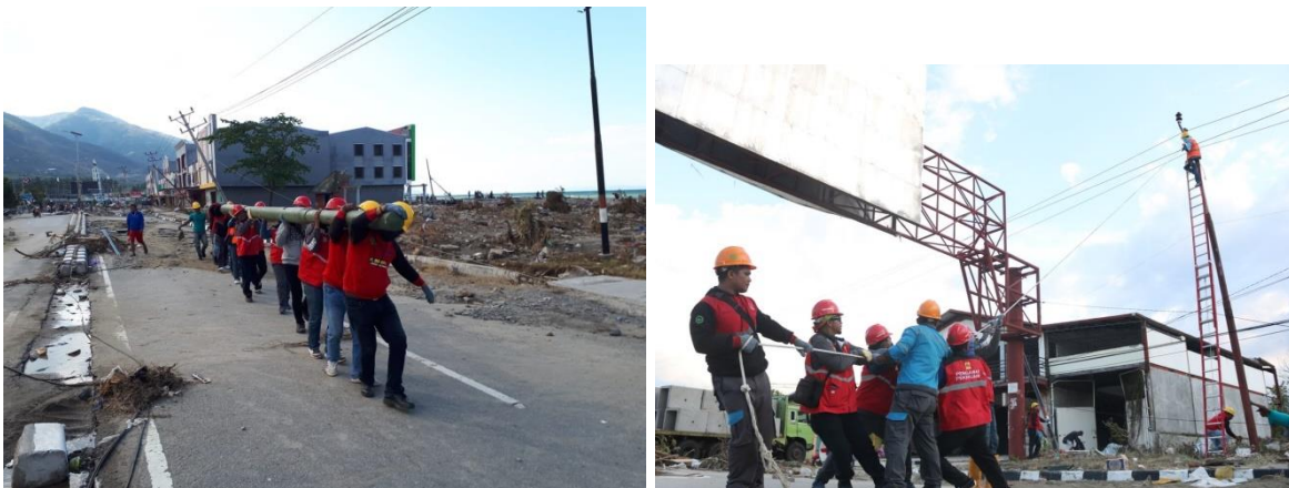
Figure 37: Installation of new power distribution poles within days of the earthquake.
