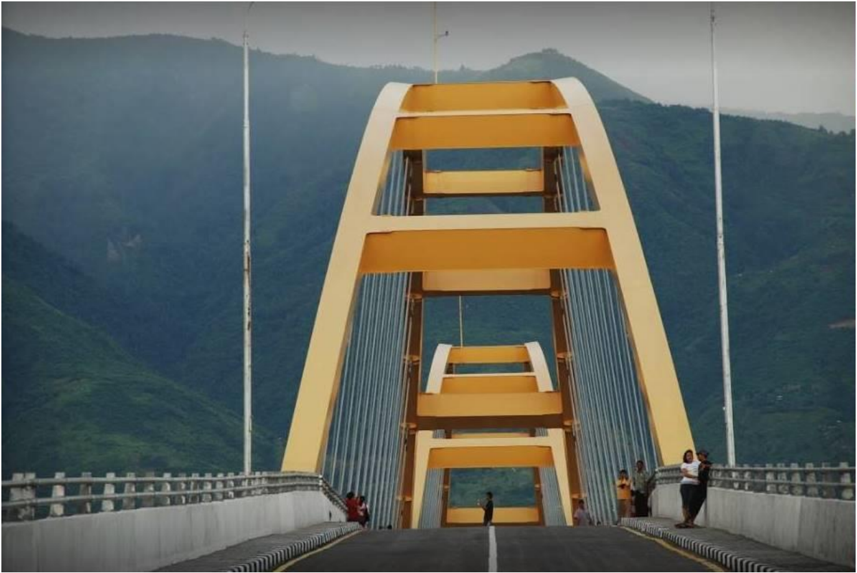
Figure 24: Palu Bridge IV before earthquake (Mohamad Affan)
