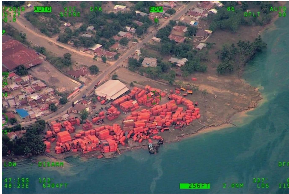
Figure 36: Shipping container yard after tsunami (0.76477 S, 119.7905 E)
