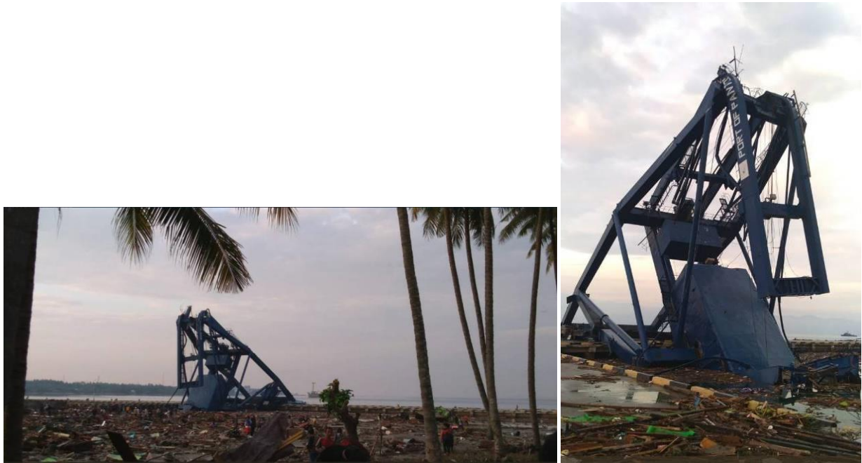
Figure 27: Failure of gantry crane (possibly at 0.710899 S, 119.85577 E)
