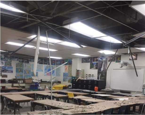
(b) Damaged suspended ceilings and Light fittings at Bartlett High School 23
