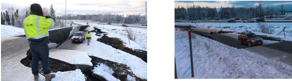
(c) Collapsed northbound onramp for International Airport Rd. at Minnesota Blvd with stranded vehicle 29 .
