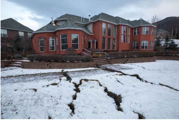
Figure 18: Home in Eagle River with significant structural damage due to geotechnical failure 14
