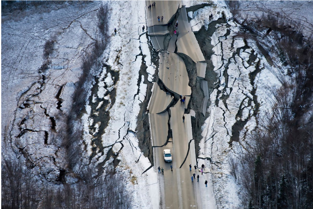
Earthquake damage on Vine Road, near Wasilla, Alaska, on Nov. 30, 2018. (Source: Time Magazine, Image Credit: Marc Lester - Anchorage Daily News/AP )
