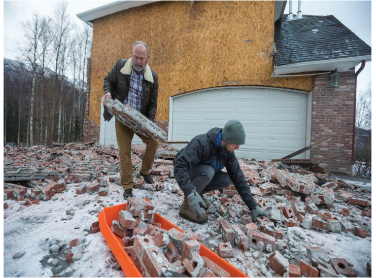
Collapsed Masonry Walls in Eagle River, Alaska
