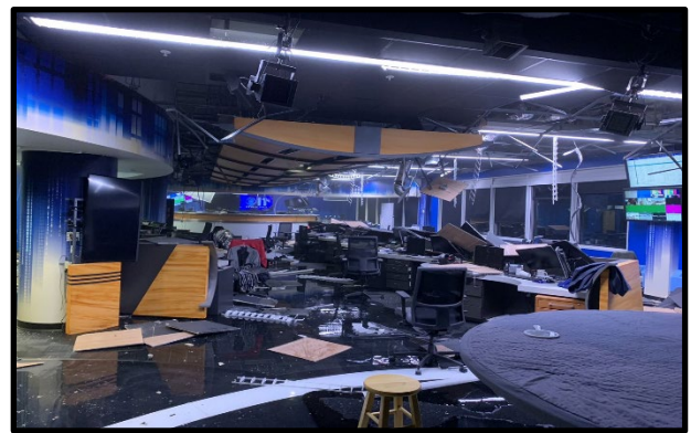
Figure 11: Window and ceiling damage at the CNN affiliate KTVA's offices 9
