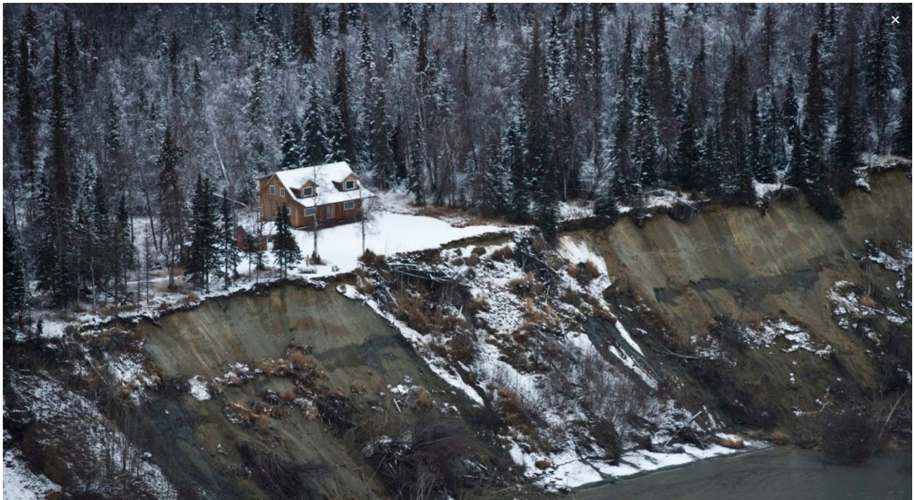
Figure 32: Landslide occurred after the earthquake, on the northwest side of Knik Arm in the Anchorage area 37
