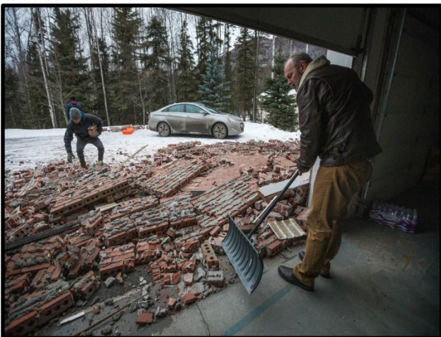
Figure 17: Brick veneer damage at residence in Eagle River 13
