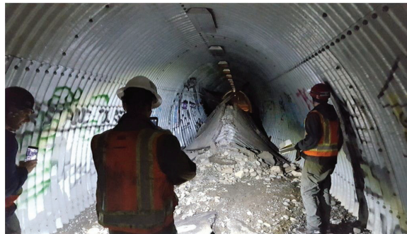
Water main that failed under the pedestrian tunnel just to the north of Briggs Bridge over Eagle River Source1 , Source2
