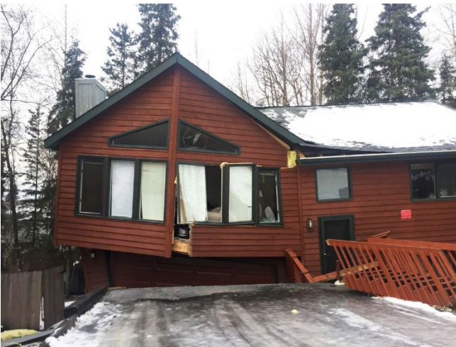
Figure 18: Home in Eagle River with significant structural damage due to geotechnical failure 14
