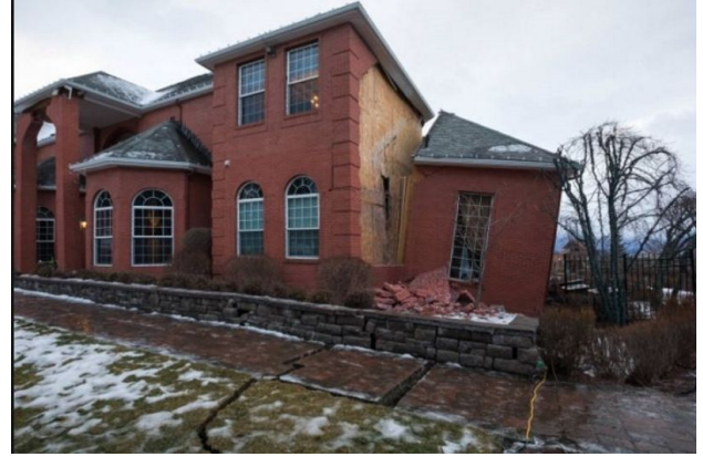
Figure 18: Home in Eagle River with significant structural damage due to geotechnical failure 14
