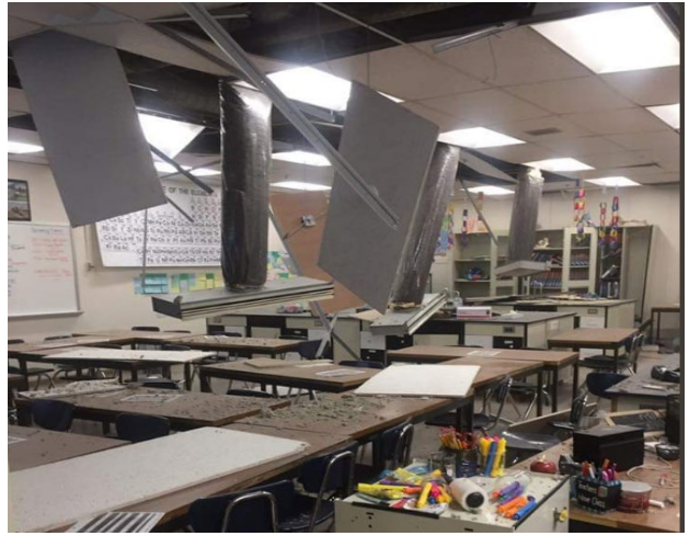
(b) Damaged suspended ceilings and Light fittings at Bartlett High School 23
