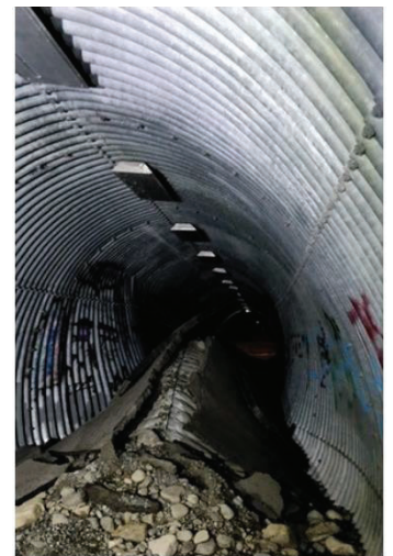
Water main that failed under the pedestrian tunnel just to the north of Briggs Bridge over Eagle River Source1 , Source2
