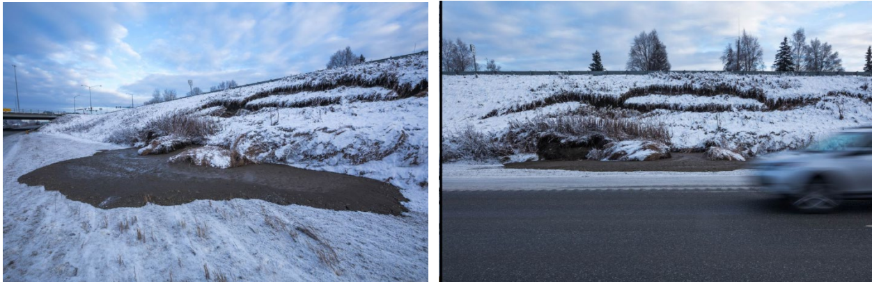
Figure 36: Mudslide along Minnesota Blvd. near Diamond 41
