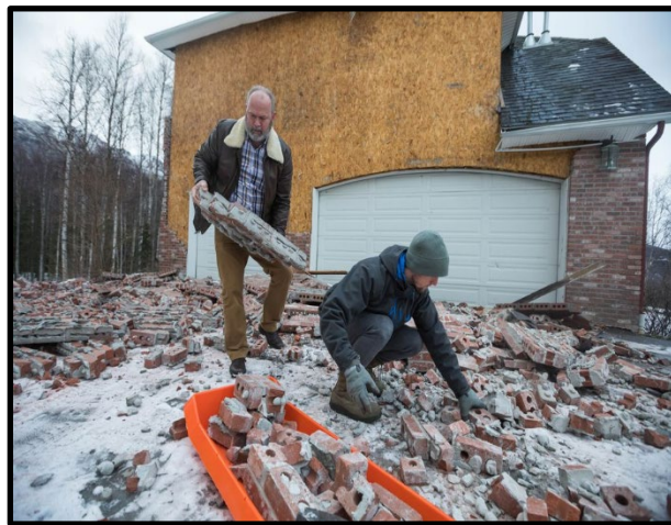
Figure 17: Brick veneer damage at residence in Eagle River 13
