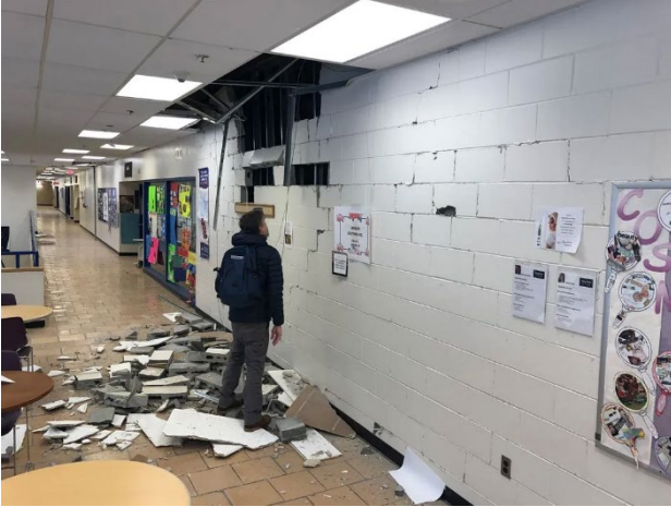
(a) Damage to masonry infill wall at King Tech High School 22
