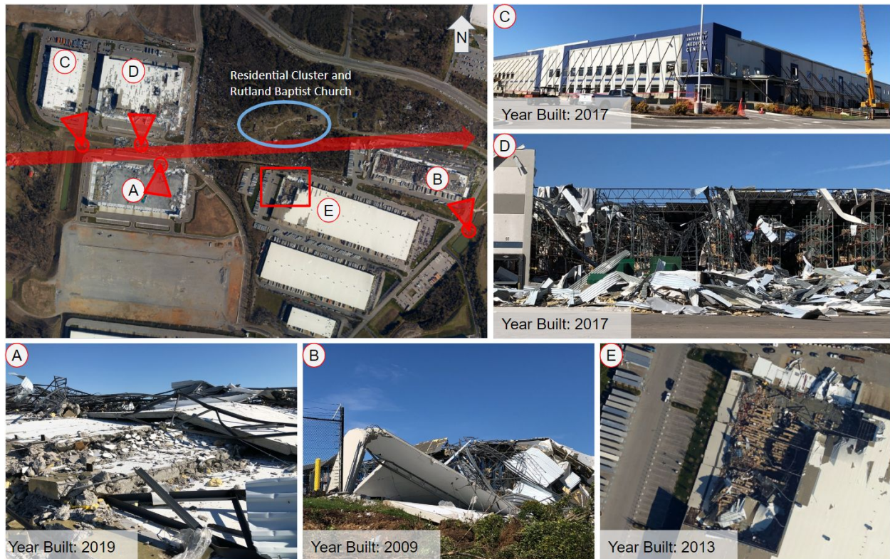
Figure 6.4.5. Damage to a cluster of modern industrial buildings between Mt. Juliet and Lebanon. All buildings were tilt-up precast concrete construction with steel roof joists and joist girders. FAST captured aerial imagery via UAV of this cluster to develop densified point clouds to facilitate measurements and further analysis. A residential cluster in the same area experienced a mixture of failures, from complete destruction of a mobile/manufactured home, removal of the roof structure of a single-family home built in 1936, minor damage to a single-family home built in 1949, and moderate damage to Rutland Baptist Church.
