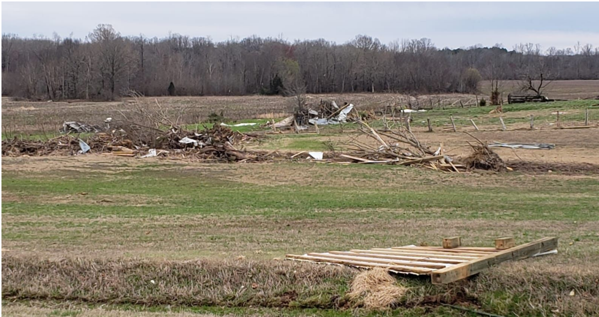
Figure 6.9.3. Debris field in rural/agricultural areas (36.087824, -88.340024) including corrugated steel from failed silos.
