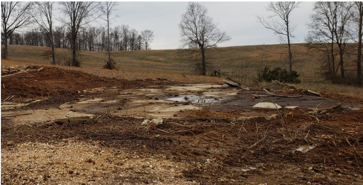
Figure 6.9.4. Steel silo failure (36.091628, -88.372416). Failure due to grouted or epoxy connection at base.
