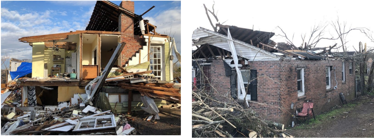
Figure 6.1.1. (left) 2-story hollow CMU residential structure with horizontal 1X wood planks for roof sheathing in Lockeland Springs; (right) single-story wood-frame home (constructed in 1945) in the Osage/North Fisk neighborhood in north Nashville with wood rafters and plywood sheathing.
