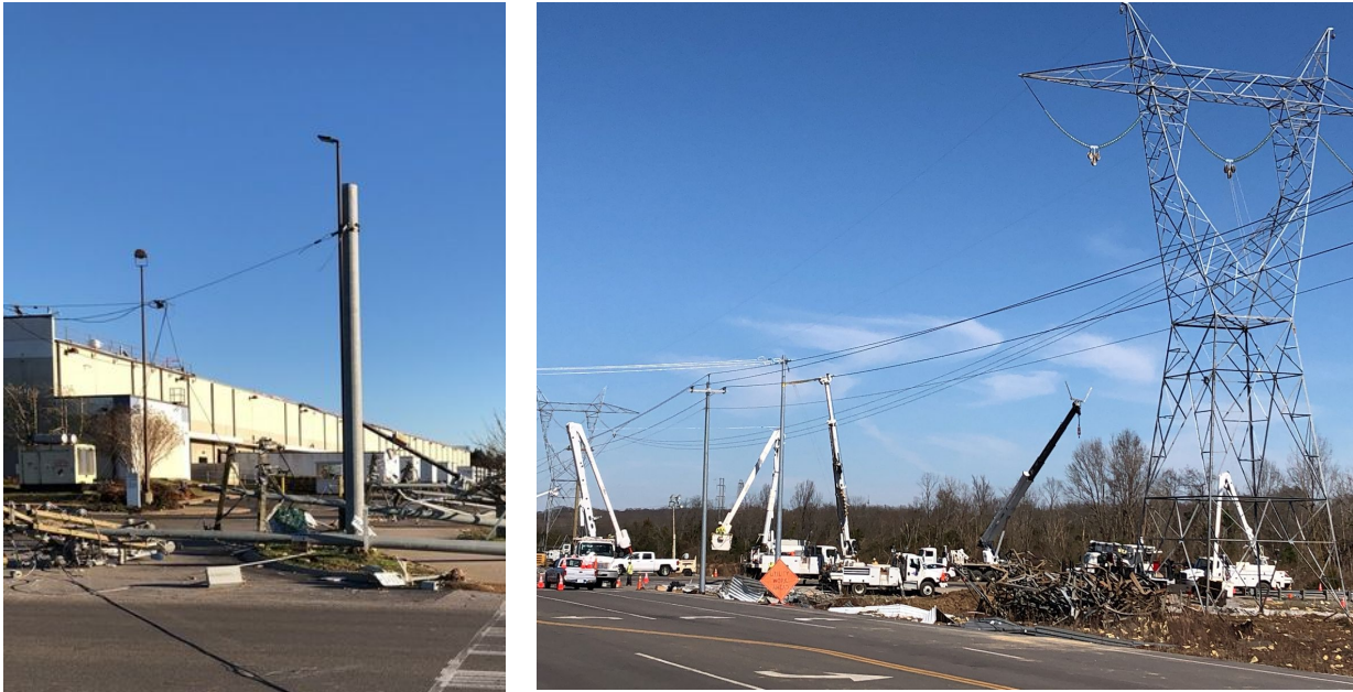
Figure 7.1.1. Illustrative damage to power infrastructure observed by FAST: (left) damage to power poles and traffic signal structure in Mt. Juliet (36.186894, -86.41586); (right) lattice towers in Mt. Juliet (Location: 36.184661, -86.464333) supporting 500 kV high-voltage transmission lines replaced after being damaged in the tornado, per the TVA .
