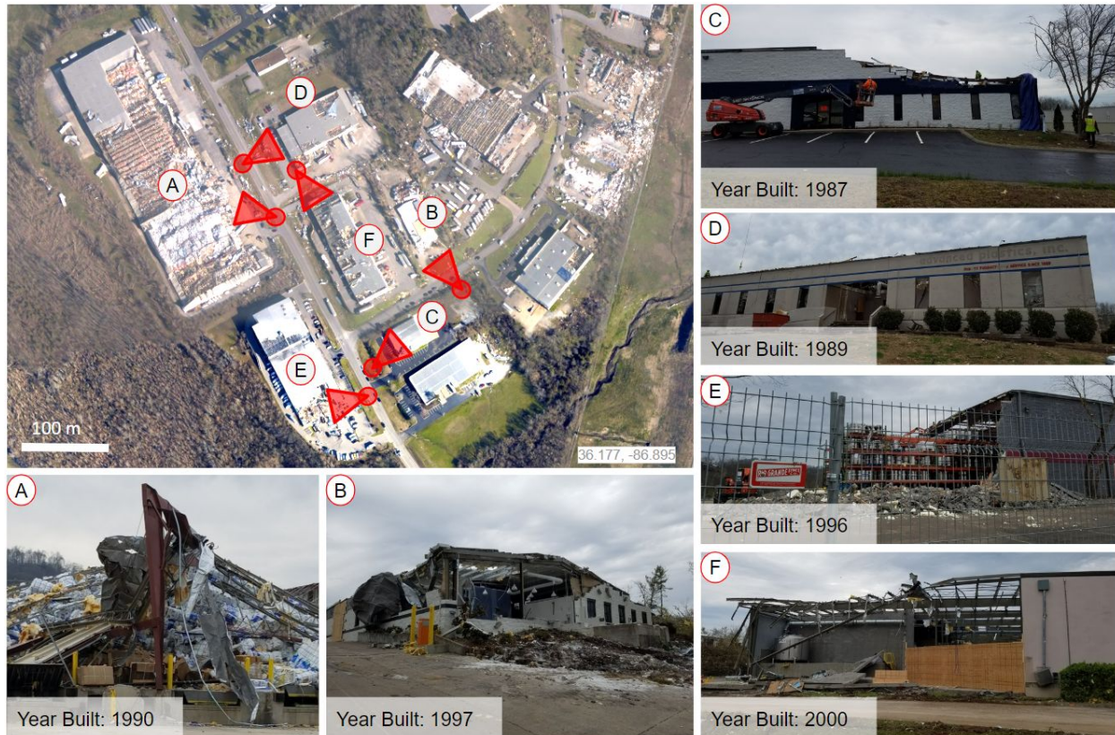
Figure 6.4.4. Cluster of damaged, large-volume industrial buildings west of the John C. Tune Airport sampled by FAST. Damage ranged from structural collapse of multiple bays (e.g., Building A) to moderate loss of metal roofing panels and insulation. Structural systems were steel-frame buildings with primarily CMU in-fill walls, steel roof joists or purlins, and corrugated metal deck.
