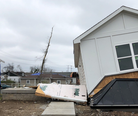
Figure 6.1.13. (left) Collapse of lower level in newly built “tall and skinny” home in North Nashville on 14th Ave.; (right) pictured is the 2nd floor with the left-hand 1st story wall laying flat. Single grouted blocks in the top course of the stem wall were still attached to the sill plate.
