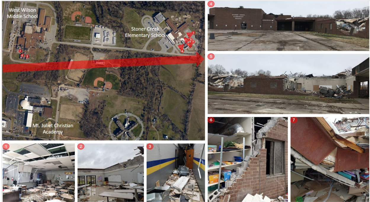
Figure 6.5.1. Overview of damage to West Wilson Middle School and Stoner Creek Elementary School in relation to the approximate tornado path (red arrow). Mt. Juliet Christian Academy sustained less severe damage but was not investigated by FAST.
