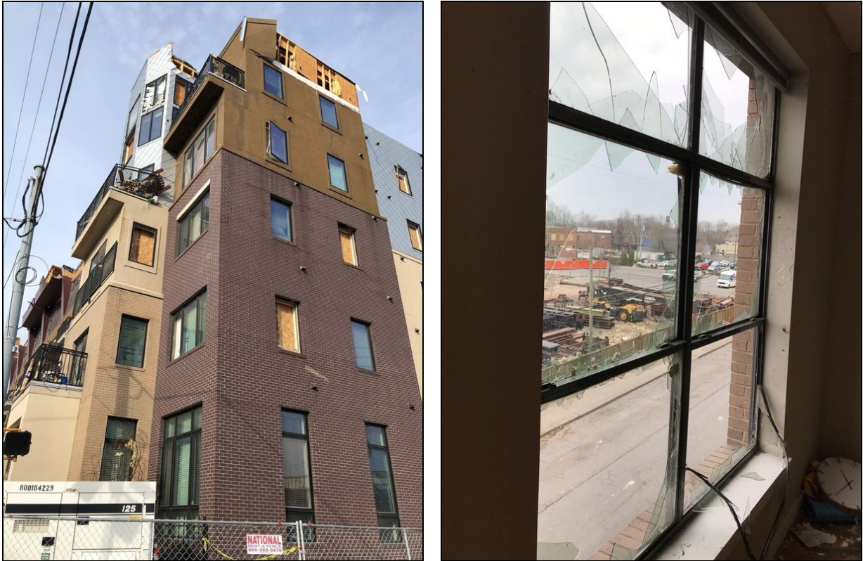
Figure 6.2.3. Typical residential structure in Germantown (Apartments >10 units). Damage primarily to windows and roofing/ top floor.
