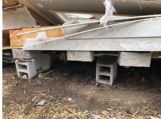
Figure 6.1.13. (left) Collapse of lower level in newly built “tall and skinny” home in North Nashville on 14th Ave.; (right) pictured is the 2nd floor with the left-hand 1st story wall laying flat. Single grouted blocks in the top course of the stem wall were still attached to the sill plate.
