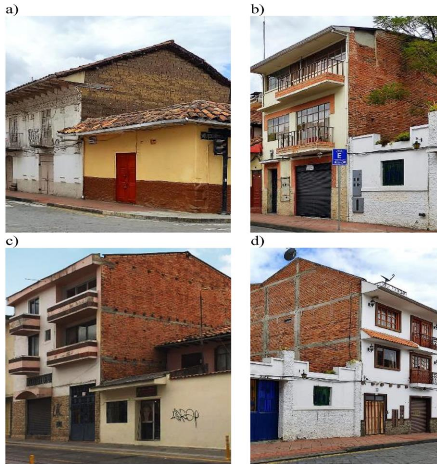
Figure 3.2. Masonry buildings typology: (a) unconfined adobe masonry, (b) unconfined brick masonry, (c) brick masonry with tie beams, (d) confined brick masonry. (Jiménez-Pacheco et al., 2022).
