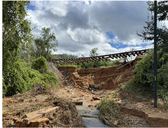
Figure 6.7. Undercutting of railway tracks in Asheville, NC (Source: Nate on X.com )
