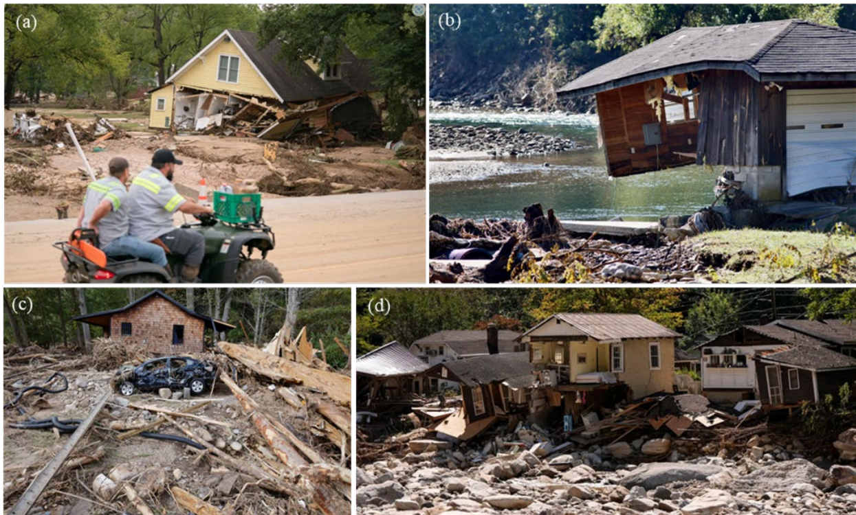
Figure 4.3.1. Outstanding examples of ravaged buildings across different regions in North Carolina: (a) Mill Creek in Old Fort, a timber residential house has been detached from foundation and carried several feet away, has sustained out-of-plane damage and debris can be seen around it (Source: Sean Rayford—Getty Images ), (b) house in Cruso at a close distance to the riverbank has been swept away due to severe scouring that compromised its structural integrity (Source: Reuters, Jonathan Drake ), (c) Barnardville, a house and other debris was found downstream hundreds of feet from its original location (Source: Reuters, Jonathan Drake ), (d) Chimney Rock Village, houses made of timber have been completely destroyed and displaced by strong currents (Source: Associated Press, Mike Stewart ).
