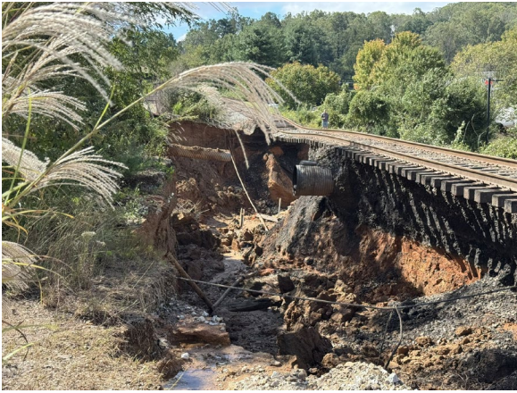
Figure 6.7. Undercutting of railway tracks in Asheville, NC (Source: Nate on X.com )
