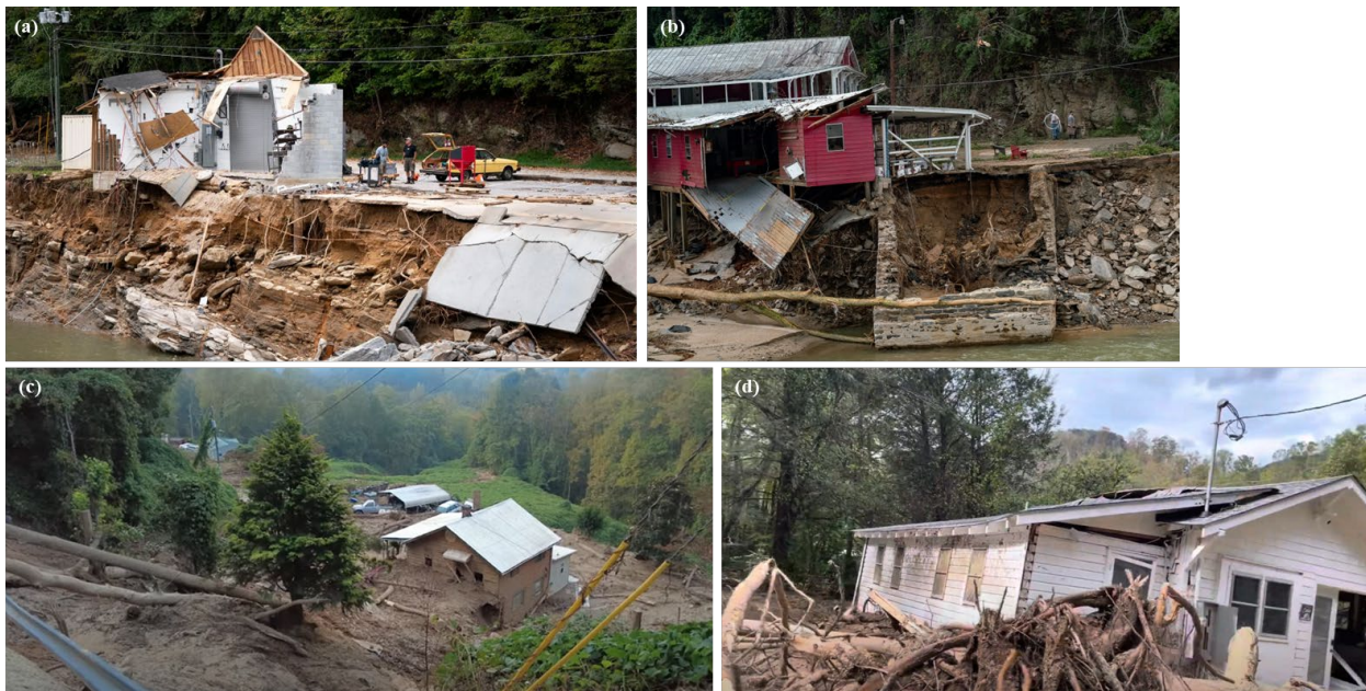
Figure 4.3.7. Four different locations in Bat Cave, North Carolina: (a) (Source: Sean Rayford/Getty Images ) and (b) (Source: New York Post , Ben Hendren ) are locations along the Rocky Broad River area that experienced unprecedented flood levels that resulted in extreme scouring/erosion that swept entire houses made of timber, (c) landslides also caused damages to houses like the one shown here (Source: video from Forbes Breaking News ) and (d) houses were also detached from foundations and were found stranded several feet away ( YouTube video by Blaine Chappell ).
