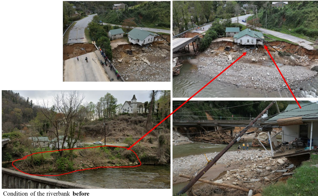
Figure 4.3.6. Severe scouring effects on the riverbanks of Rocky Broad River in Bat Cave, North Carolina. (Source: Google Street View (before) and starting from top left and going clockwise: New York Times , Christian Monterrosa , and the right two from Reuters , Marco Bello ).
