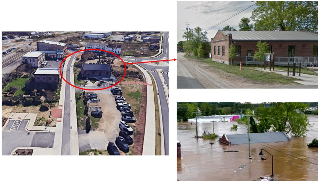
Figure 4.3.3. Flooded region before and after in the River Art District, Asheville, North Carolina (Source: Google Street View (before) and @nctradlines / Reuters (after)).
