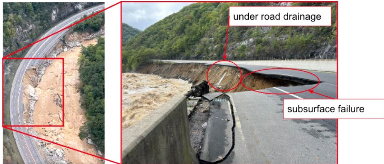
Figure 5.5. Damage to I-40 near the TN/NC border (photos from helicopter video posted to X , and photos posted to Threads ).
