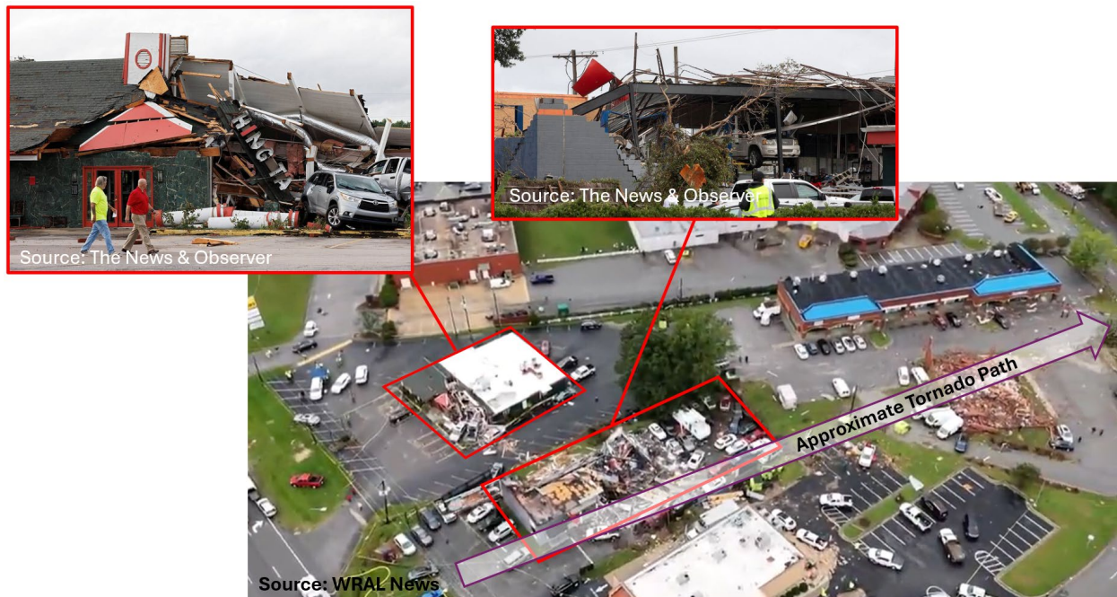
Figure 4.3.8. Several commercial structures were destroyed in downtown Rocky Mount, NC by an EF-3 tornado (Sources: inset photographs from Raleigh News & Observer , base aerial image from WRAL News ).
