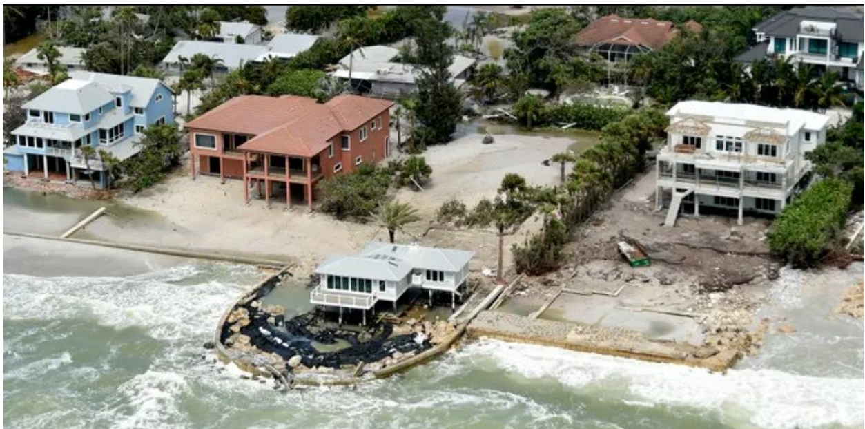
Figure 4.1.4. Beach erosion and wind-induced damage to the building on the right of the image in Longboat Key, FL (Source: Thomas Bender ).
