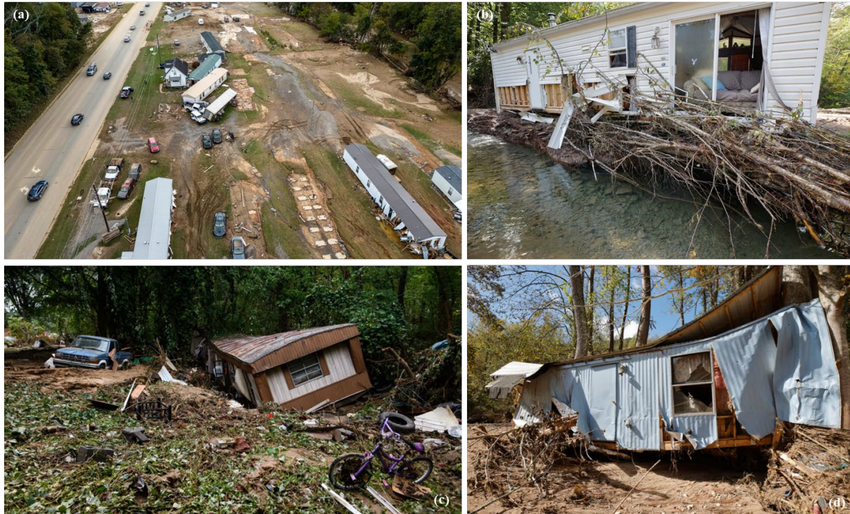
Figure 4.3.2. Examples of impacts to mobile homes in North Carolina: (a) in Swannanoa, mobile homes and vehicles displaced by flood waters, the footing structure for one of the mobile homes can be seen in the bottom right of the picture (Source: Associated Press Photo, Mike Stewart ), (b) mobile home in Cruso, swept away by surging creek (Source: Reuters, Jonathan Drake ), (c) in Old Fort, vehicle and mobile home pushed into tree line (Source: Getty Images, Melissa Sue Gerrits ), (d) in Barnardsville, a trailer home completely deformed and destroyed by the impacts of flooding (Source: Reuters, Jonathan Drake ).
