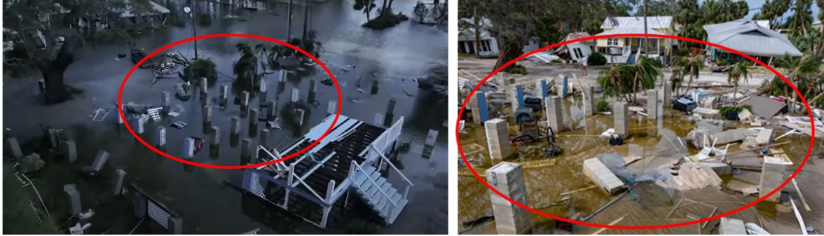
Figure 4.1.1. Elevated structures washed away by storm surge and wave loads in Cedar Key, FL (Source: Greg Lovett ).
