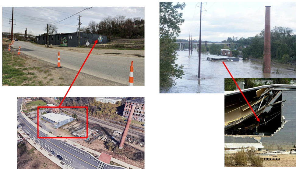
Figure 4.3.4. The images on the left focus on a specific building (building 99 - Second Gear and Sugar and Snow Gelato, Asheville, North Carolina) within the district, that was repurposed to host commercial stores. The water levels reaching close to the roof can be seen in the upper right image and out-of-plane failure for one of the walls is visible in the bottom right photo. (Source: Google Street View (pictures before) and Citizen Times, Jacob Biba and detail of damage from Glen Miska (pictures after)).
