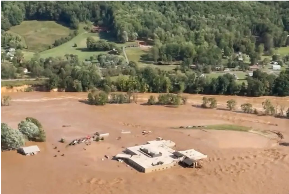
Figure 4.4.1. Unicoi County hospital impacted by flooding along the French Broad River in Erwin, TN (Source: Wade Payne/Associated Press ).
