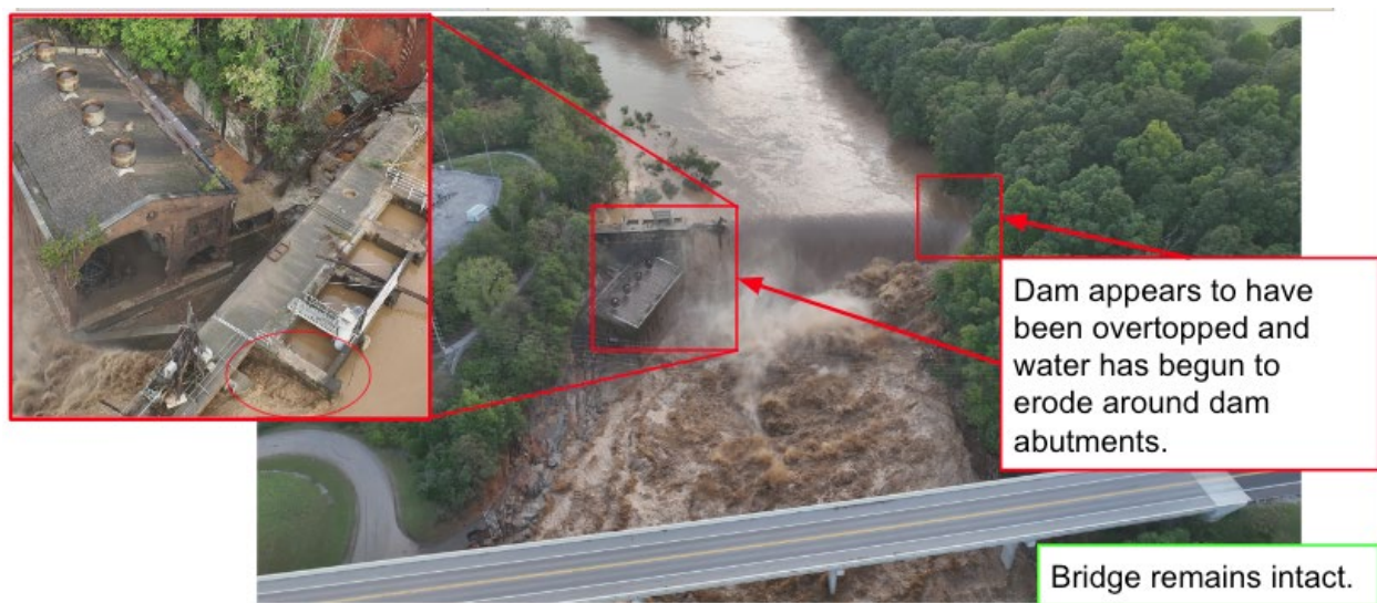
Figure 5.6. Overtopping of the Nolichucky Dam with erosion damage (Photos from Tom Satkowiak via X ).
