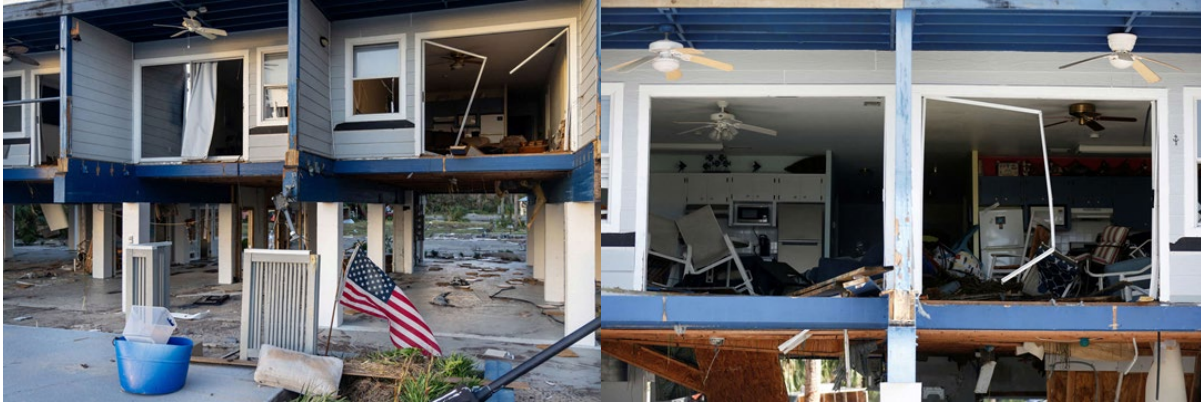
Figure 4.1.5. Damage to balconies, facades and other non-structural elements of elevated buildings in Steinhatchee, FL (Source: Kathleen Flynn, Reuters ).
