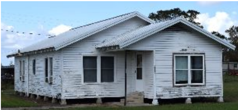
Figure 4.5. Typical older home (approximately 1940s construction) in communities along LA-14. Inset photo shows that such homes are elevated on concrete piers of various heights with no positive attachment (Credit: FAST-1).
