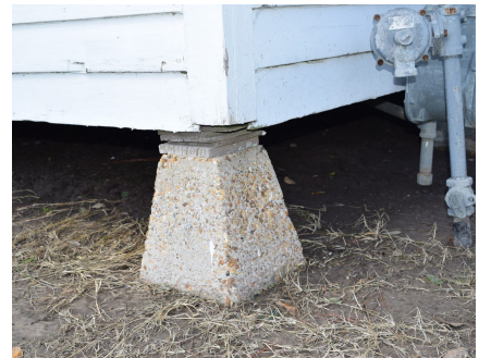
Figure 4.5. Typical older home (approximately 1940s construction) in communities along LA-14. Inset photo shows that such homes are elevated on concrete piers of various heights with no positive attachment (Credit: FAST-1).
