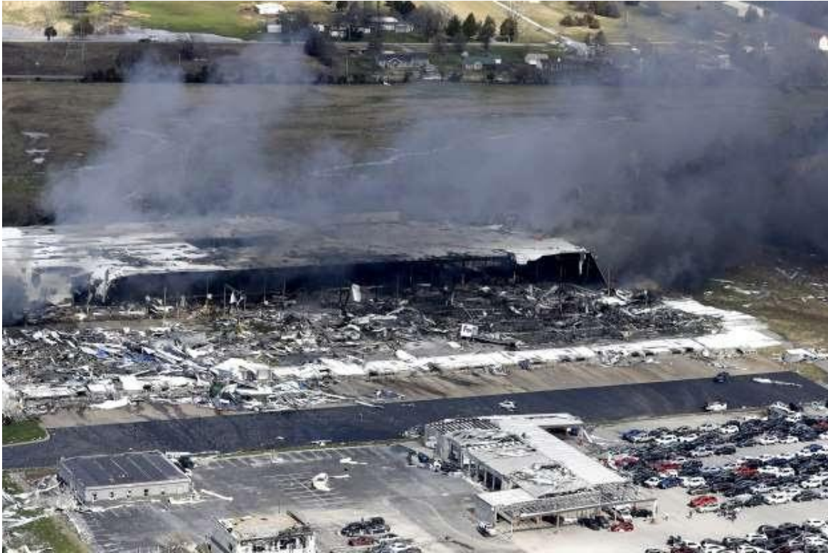
Figure 4.15. Precast tilt-up concrete building with approximately 50% of the building footprint collapsed. Photos indicated the facility caught on fire during/after the tornado. (Source: Mark Humphrey / AP Photos ). GPS: 36.187, -86.434.
