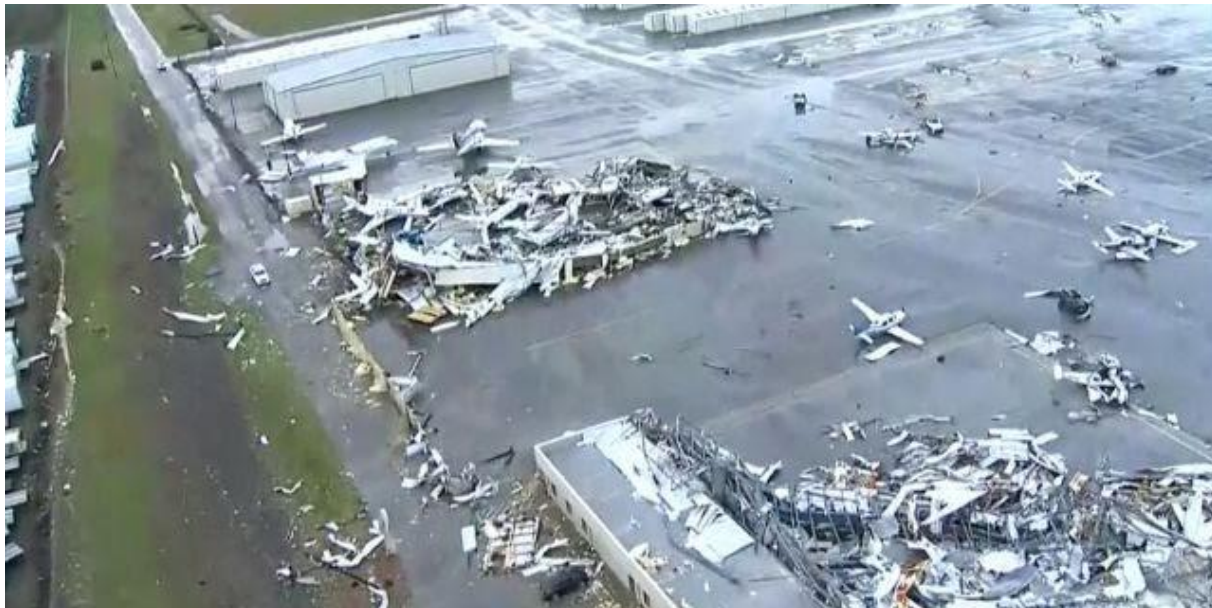
Figure 5.3. Damage to John C. Tune Airport, Nashville International's sister airport in West Nashville (Source: Fox News )
