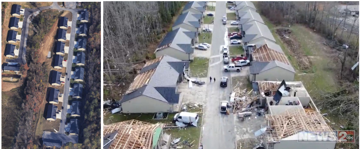
Figure 4.11. Damage to multiple duplex residential buildings near Broad St. (Cookeville, TN) (GPS: 36.170992 -85.537113): before and after the tornado (source: wkrn news ), looking North.
