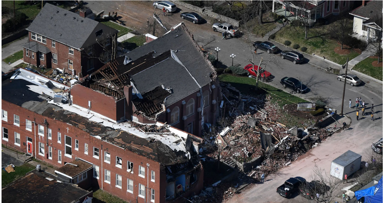
Figure 4.23. Heavy damage to the East End United Methodist Church at 1212 Holly in East Nashville (Source: George Walker IV / Tennessean.com).
