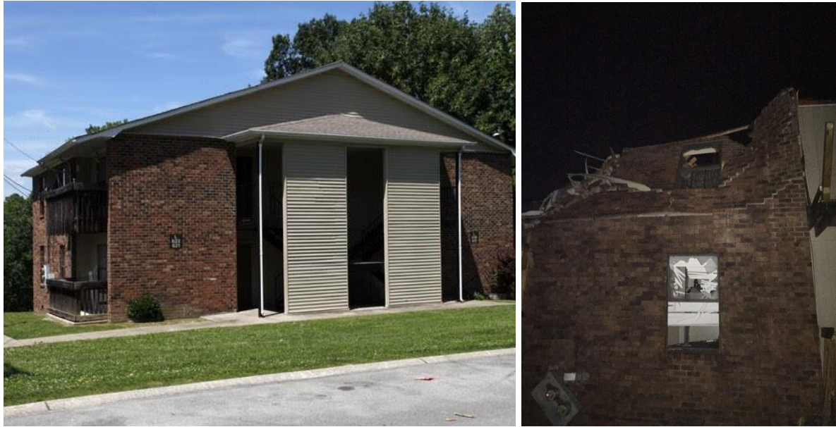
Figure 4.8. Margaret Robinson Apartments before and after the tornado (GPS 36.178388 -86.597882; source: tmj4 ).
