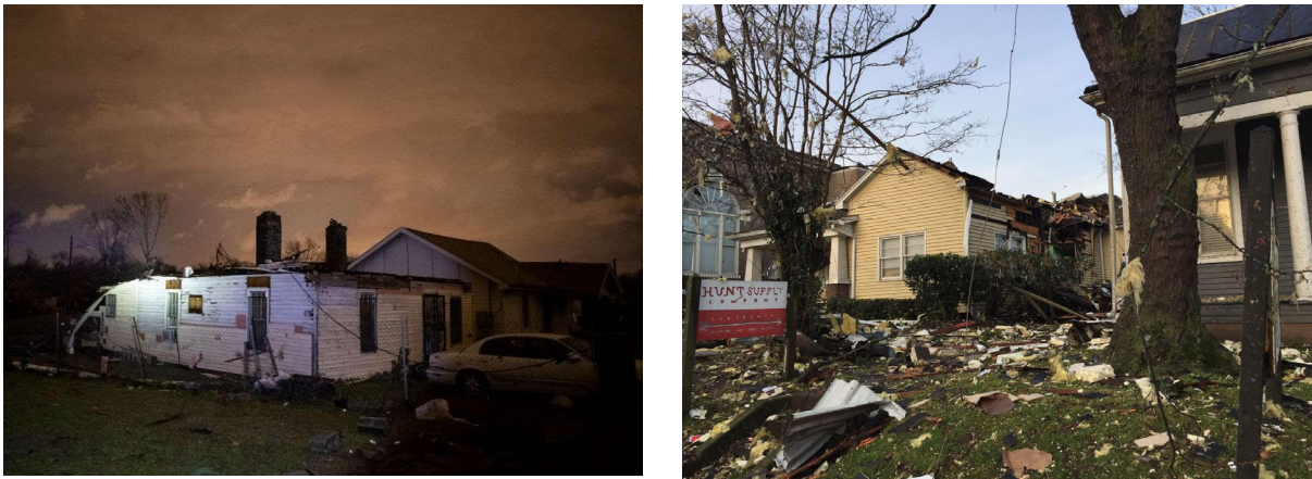
Figure 4.2. Roof structure damage to (left) a single-family house located in Underwood St. (Source: Brett Carlsen/Getty Images ); (right) roof damage to a single-family house located on Russell St. in East Nashville (GPS: 36.176342 -86.750374; Source: Ruth Ann Cox ).
