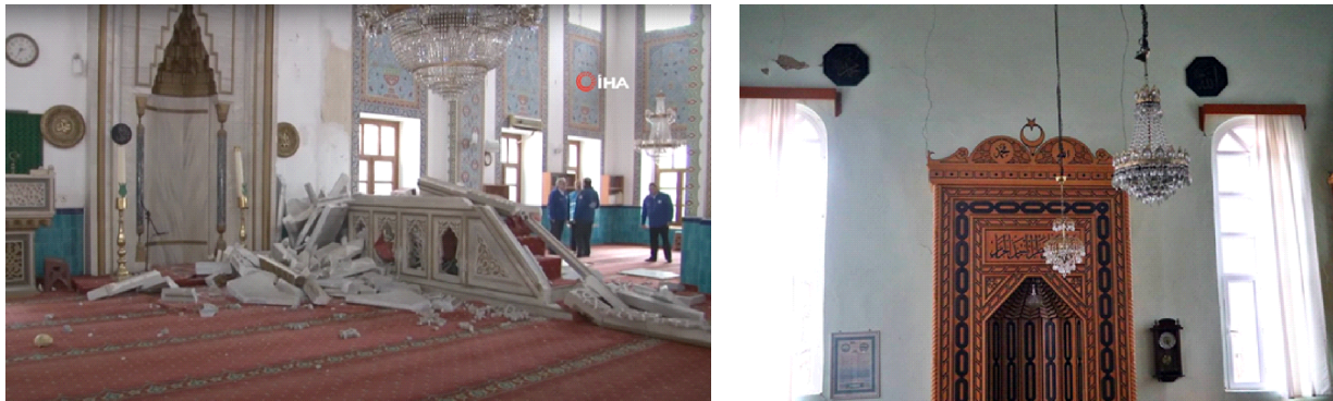
Figure 4.12. Damage to (a) Duzce Cedidiye mosque at 40.838°N, 31.163°E and (b) Saz village mosque in Kaynaşli, Duzce (Sources: (a) Anadolu Ajansi (2022), (b) KARAR.tv (2022)).
