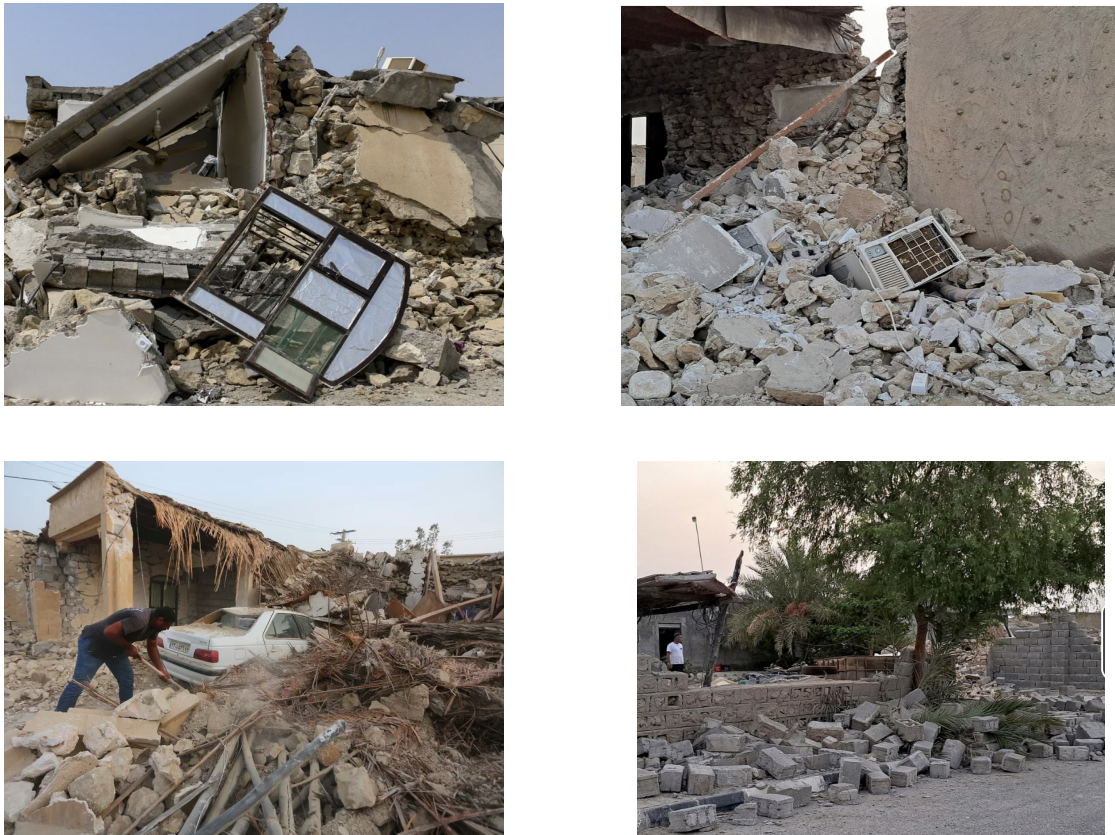
Figure 3. Collapsed masonry buildings in Sayeh Khosh village (AP, 2022; Reuters, 2022).
