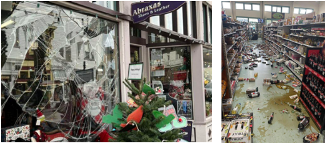
Figure 5. Shattered storefront windows and goods fallen off the shelves in a market in Ferndale (San Francisco Chronicle, 2021)
