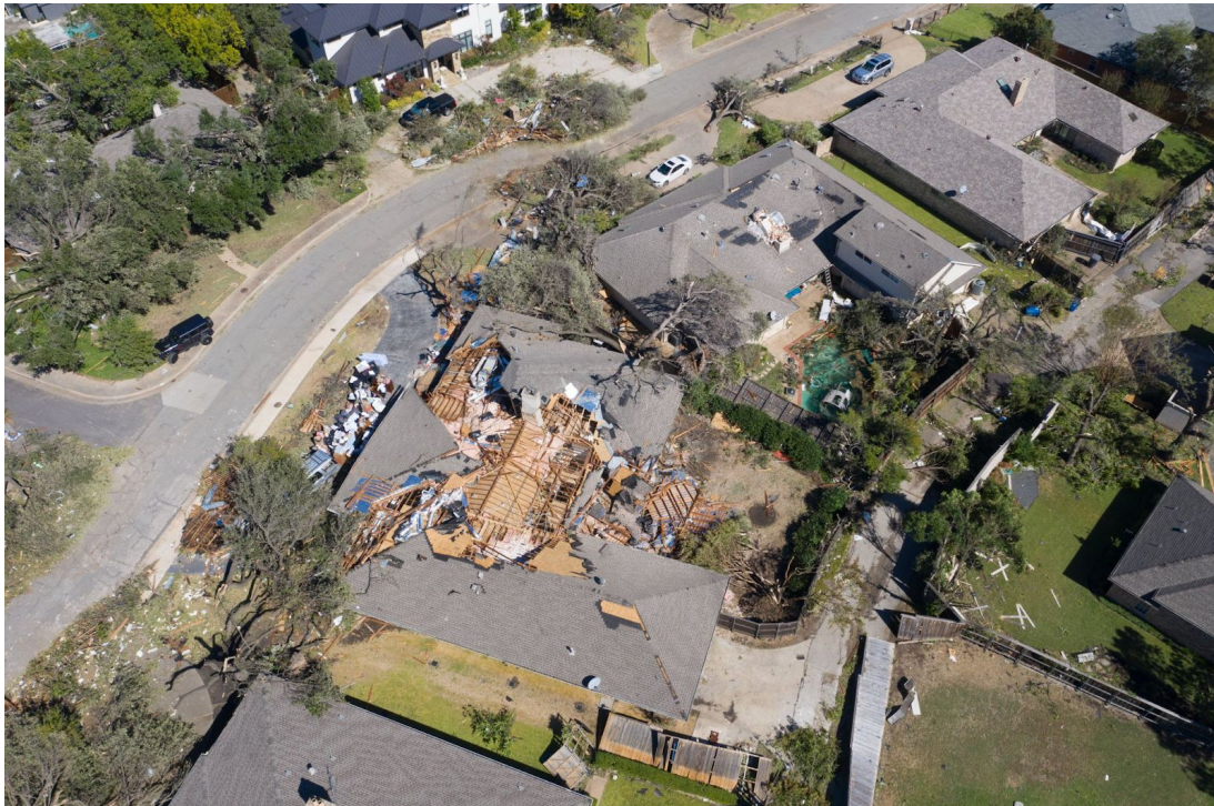
Figure 11. Isolated roof damage to a single-family home with limited impacts to adjacent homes (Source: Twitter via @Jberm236 ).
