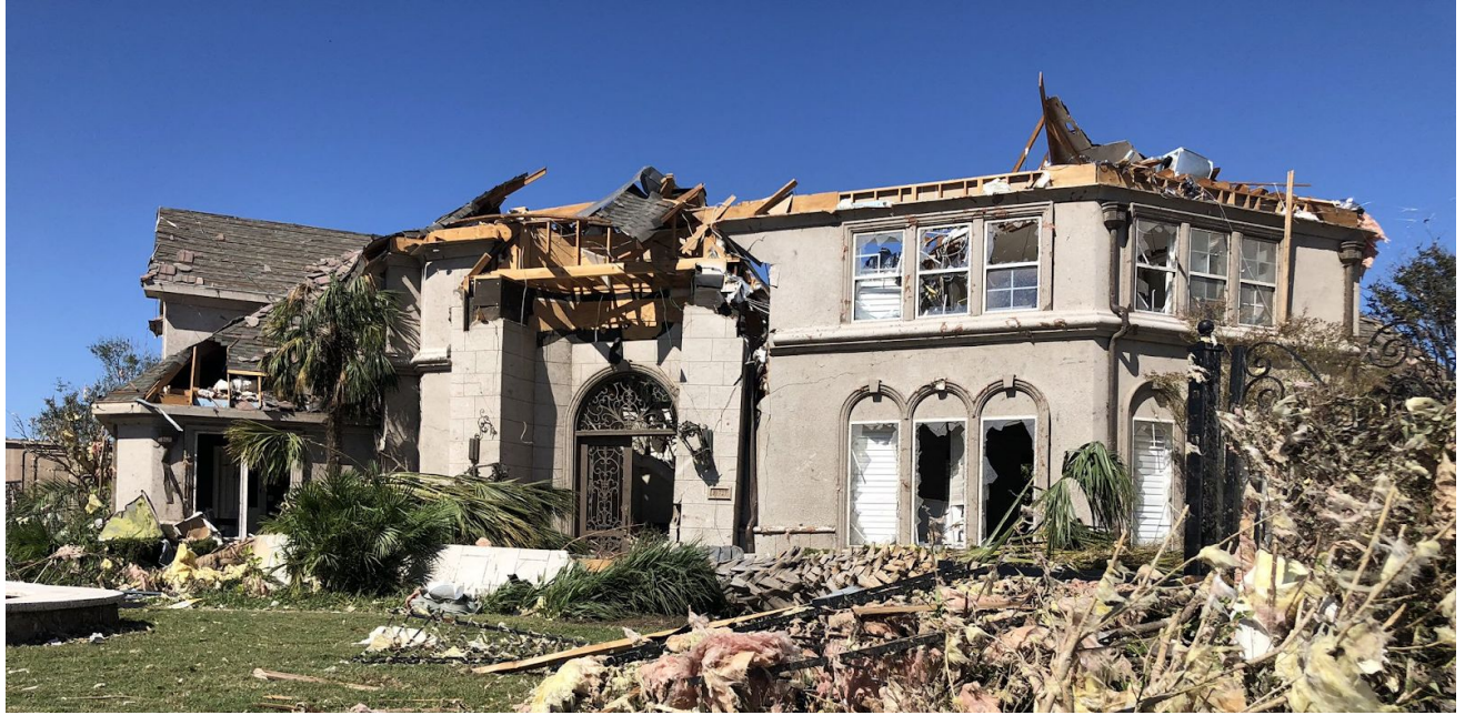
Figure 12. Damage to a single-family home in the Preston Hollows neighborhood (Source: CBS 11 ).
