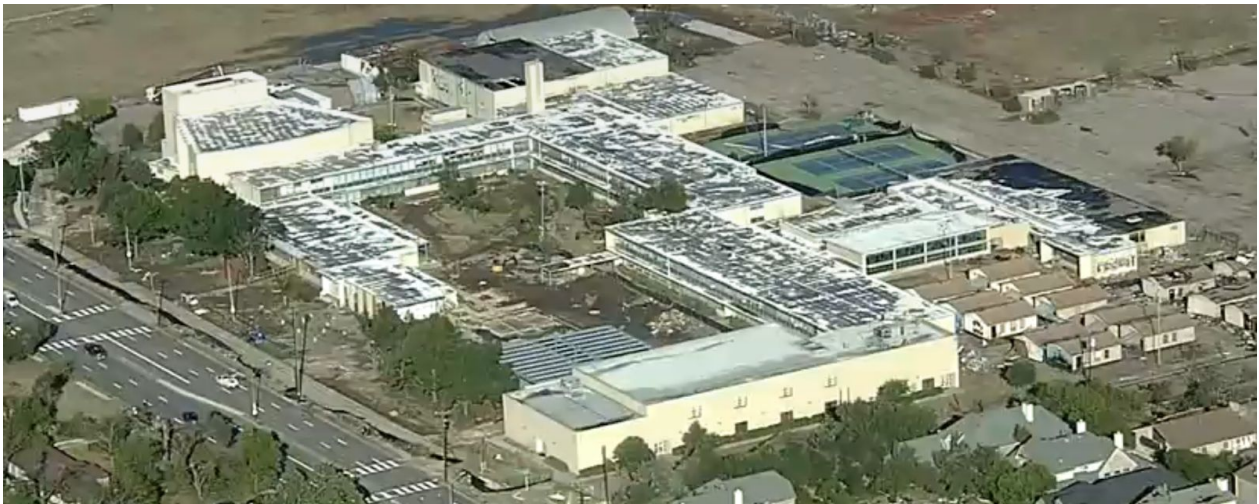
Figure 3. Thomas Jefferson High School with primarily envelope and cladding damage to the main facility (Source: Fox 7 Austin ).
