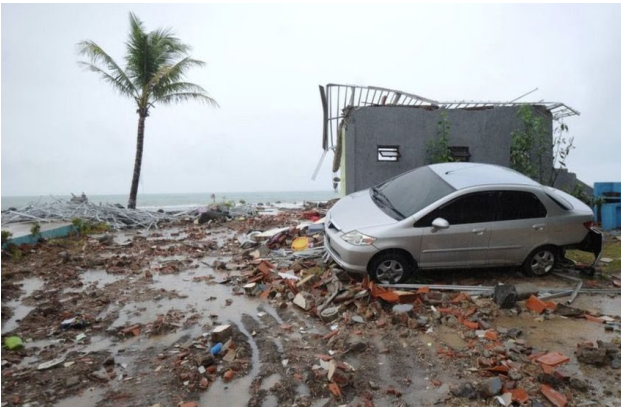
Figure 23: Floating debris, and particularly vehicles, appeared to enhance the hydrodynamic and impact loading on structures.
