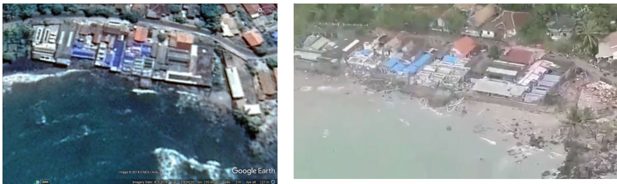
Figure 26: Google Earth (left) and aerial video (right) images of damage to coastal buildings on the South shore of Sumatra (5.82414S, 106.600E)
