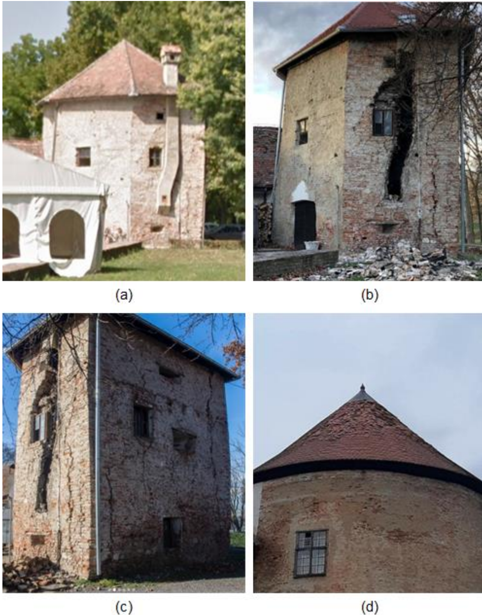
Figure 4.83. (a) Small tower connected to the Sisak fortress in 2011 (source: Google), (b, c) collapsed chimney in the small tower, and (d) damage to the tiles of the conical roof of one of the tower of the fortress (source: Instagram account starigradsisak and dvorcistarigardovi).
