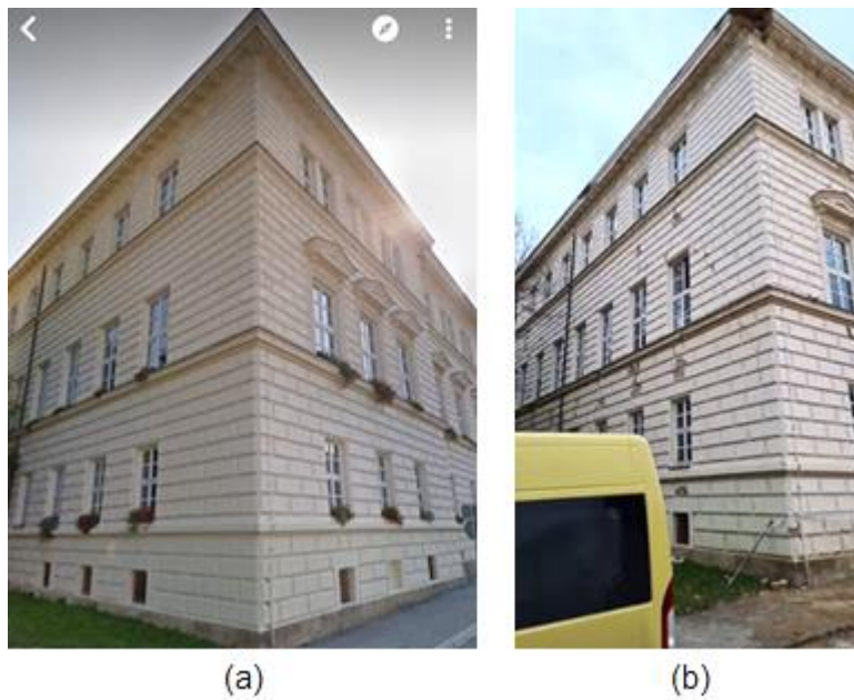
Figure 4.51. Transverse wall of Petrinja High School (a) before the earthquake (source: Google Street View) and (b) after the earthquake (source: Nenad Bijelić).
