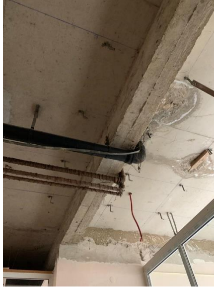
Figure 4.35. Exposed piping and fasteners for the hung ceiling (source: Damir Lazarević).
