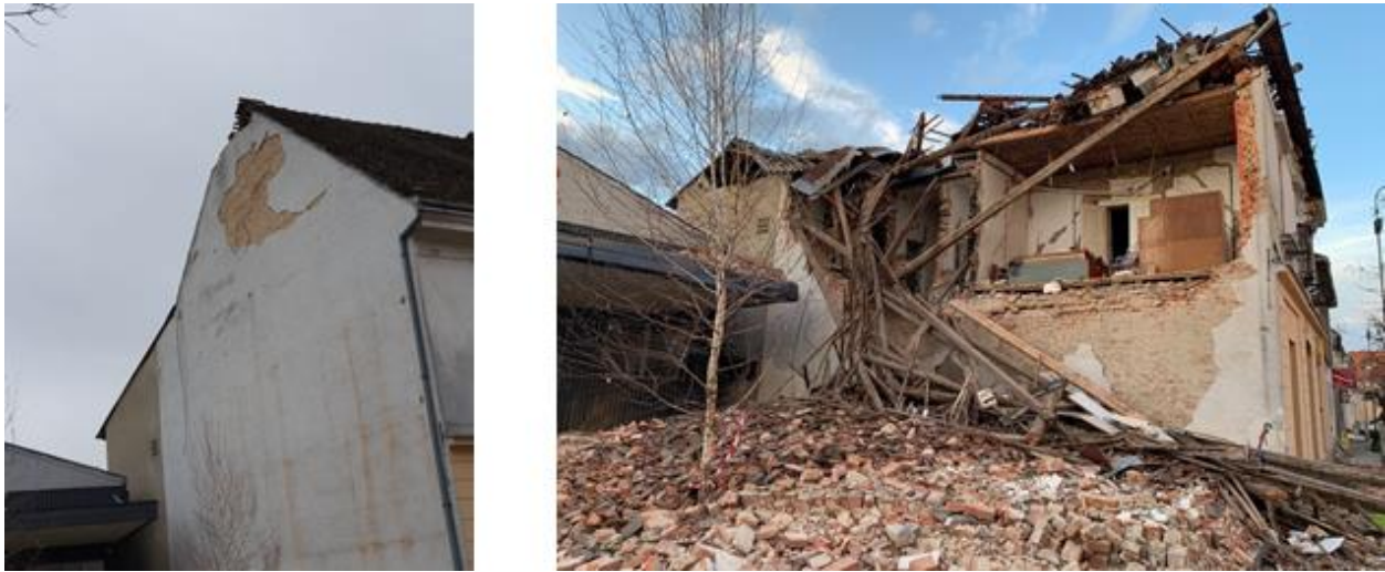
Figure 4.3. Typical wall and floor construction in older URM buildings, characterized by thick clay brick masonry walls, timber floors, and roofs. This building in Petrinja (adjacent to the KTC supermarket) was not significantly damaged in the December 28 M_w 5.2 earthquake but experienced gable wall and roof collapse in the December 29 M_w 6.4 earthquake (source: Joško Krolo).
