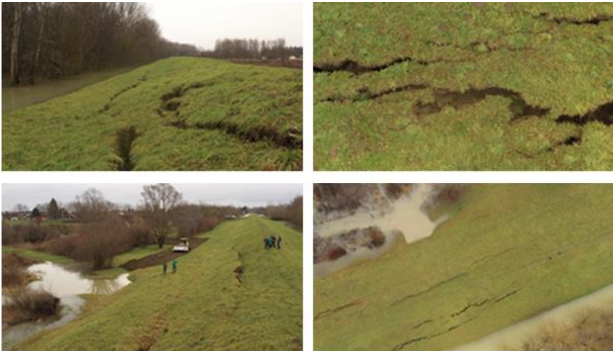
Figure 6.14. Embankment / levee failure by river Sava in Galdovo (source: Croatian Waters Archive).
