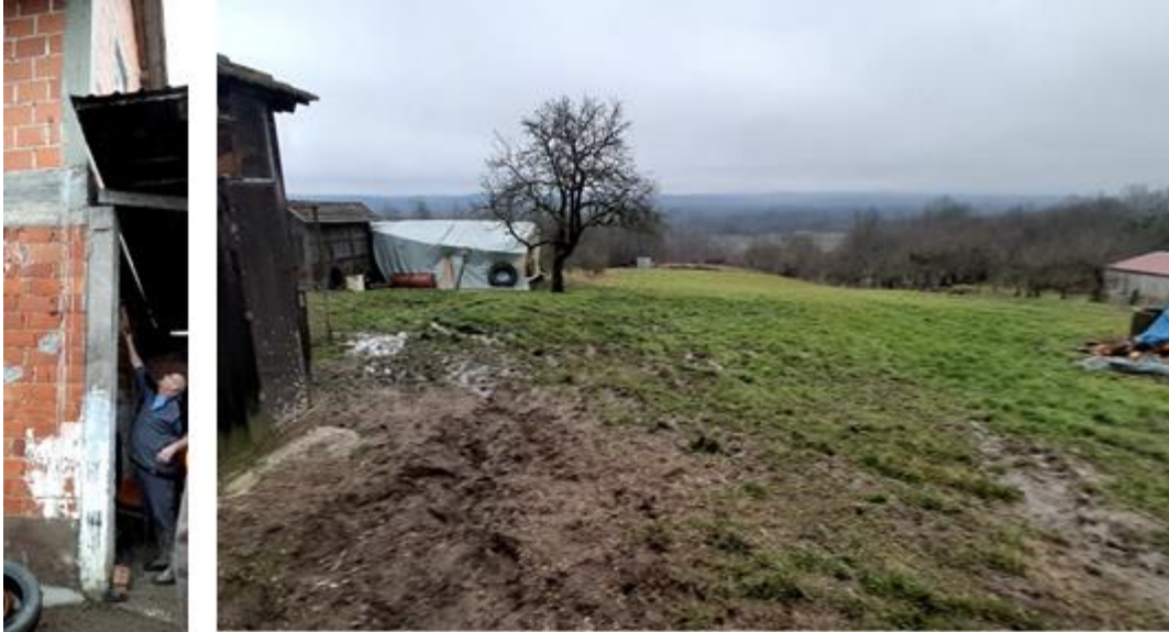
Figure 6.29. Neighboring the previously known landslide in Hadžar, is a small farm where various houses started moving down the slope, in different directions. The figure on the left shows a gap opening after the earthquake. The grass covered slope, usually firm even in rainy days, as rain would quickly run off, suddenly became wet and soft - maybe due to liquefaction in the shallow layer, which released water to the upper surface layer (45.3795,16.1199, source Sonja Zlatović).
