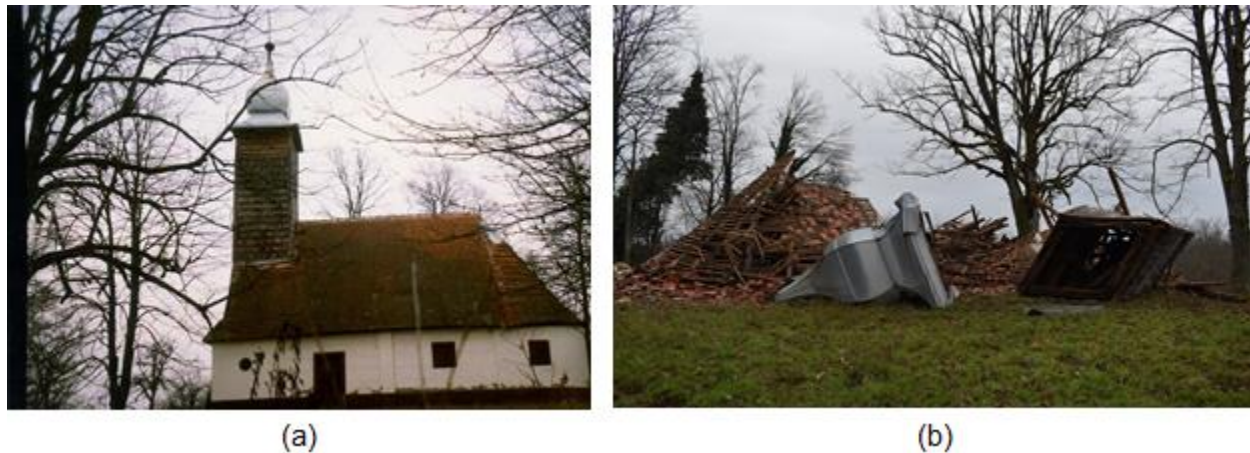
Figure 4.99. (a) Church in Majske Poljane (Hram Vaskrsenja Gospodnjeg) before the earthquake (source: Eparhija Gornjokarlovacka) and (b) Complete collapse of the Church (source: Eparhija Gornjokarlovacka).
