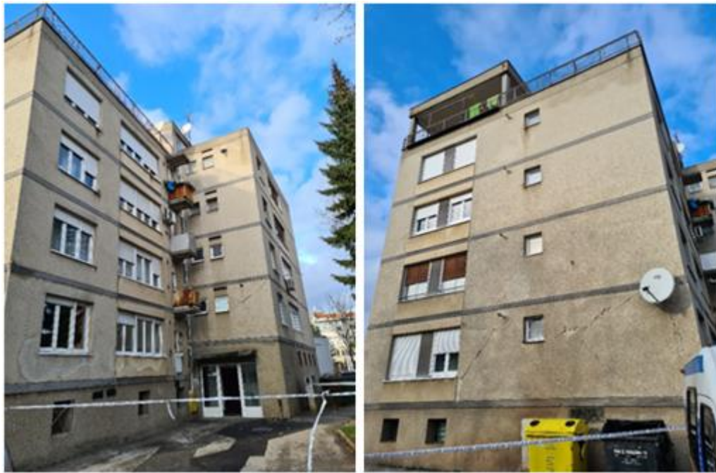
Figure 4.19. Damaged Building 3: exterior view and cracking pattern at the ground floor level (source: Nenad Bijelić).
