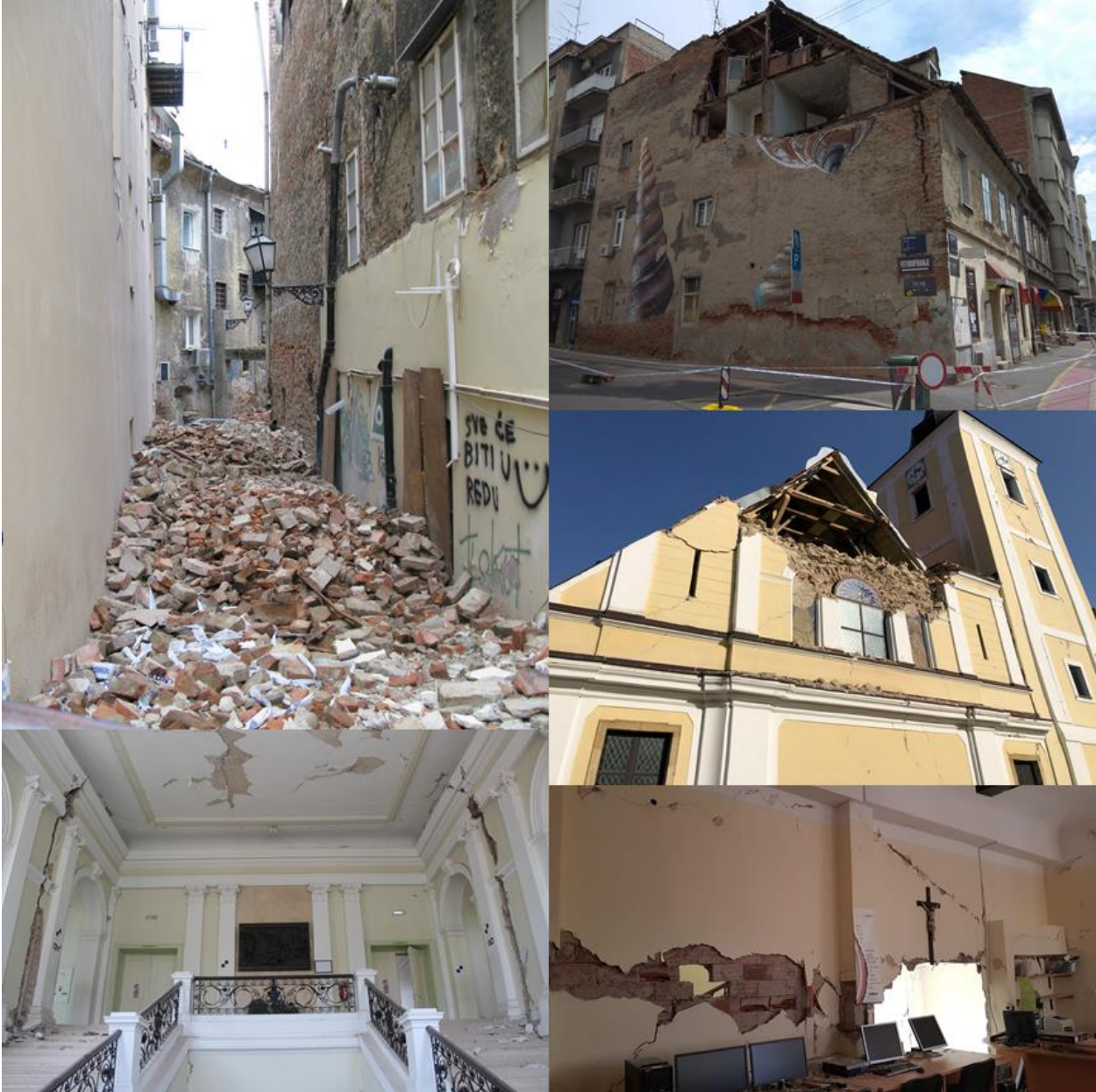
Figure 1.2. Photos of damage in Zagreb caused by the March 22, 2020 earthquake. (source: (1CroCEE 2021).
