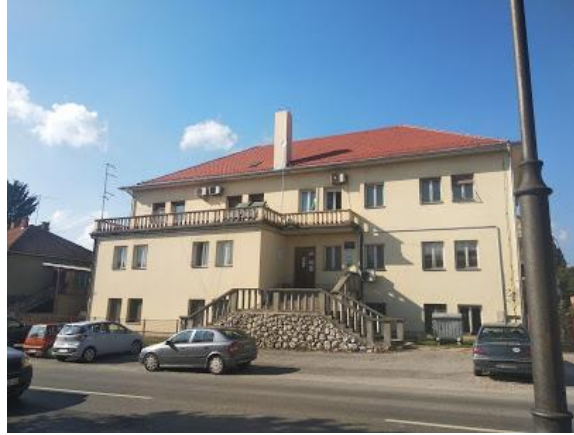
Figure 4.37. Outside view of the health center in Petrinja before the earthquake, showing its clay tile roof and stucco facade (source: Google Earth).
