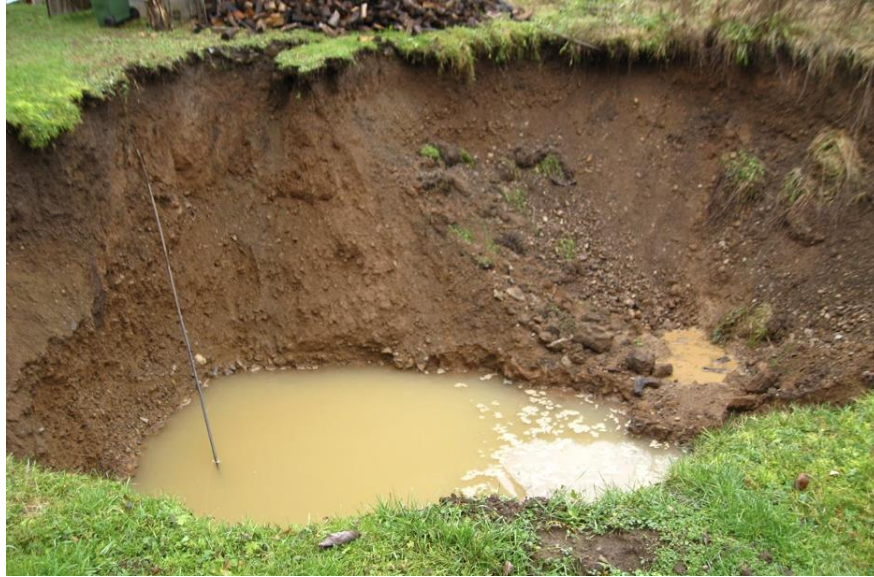
Figure 6.26. Sinkhole in Mečenčani (45.2829,16.4298, source Sonja Zlatović).
