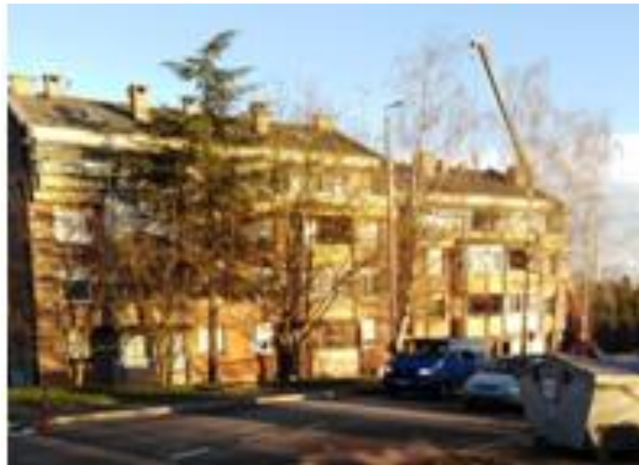
Figure 4.24. Removal of the chimneys from the roof of an RC building, "Brzaj" settlement in Sisak (source: Maja Freiberger).
