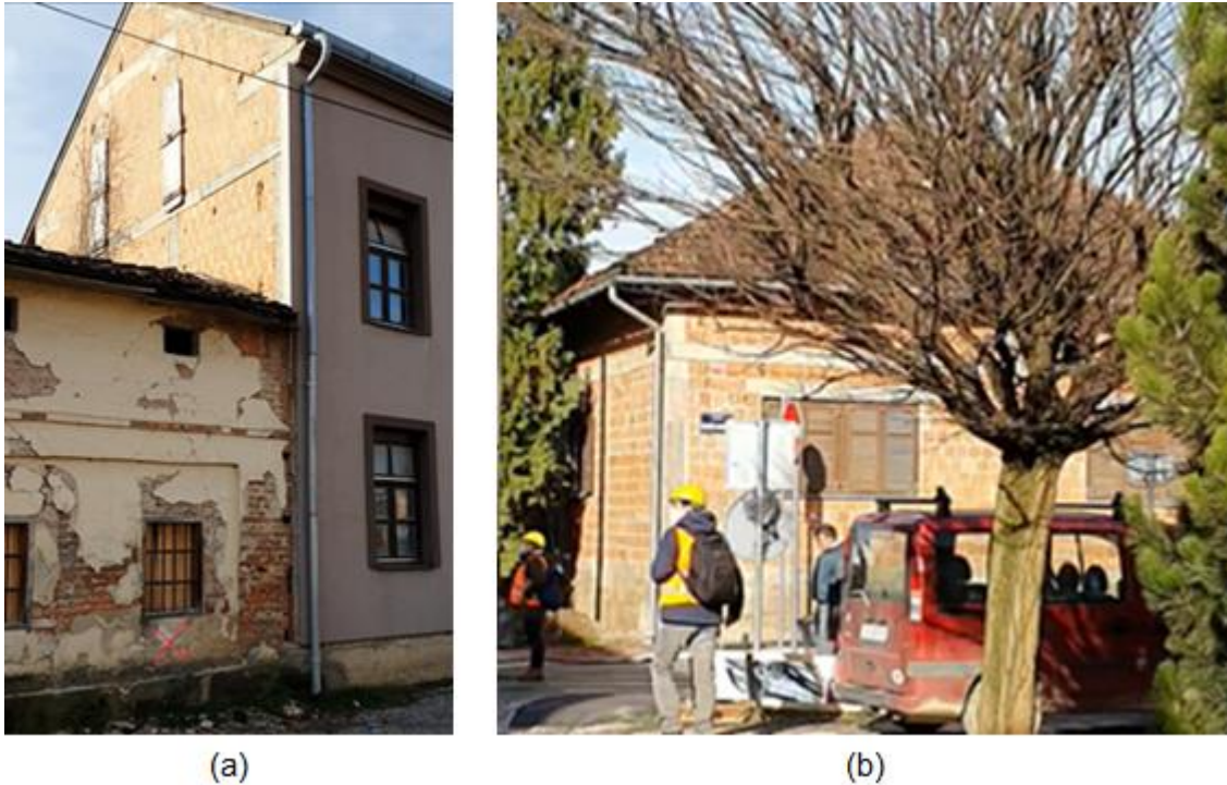
Figure 4.10. Examples of good performance of confined masonry buildings in Petrinja: (a) a two-story confined masonry building remained undamaged while an adjacent older URM building experienced severe damage; and (b) an undamaged single-story confined masonry building (source: Marko Bartolac).
