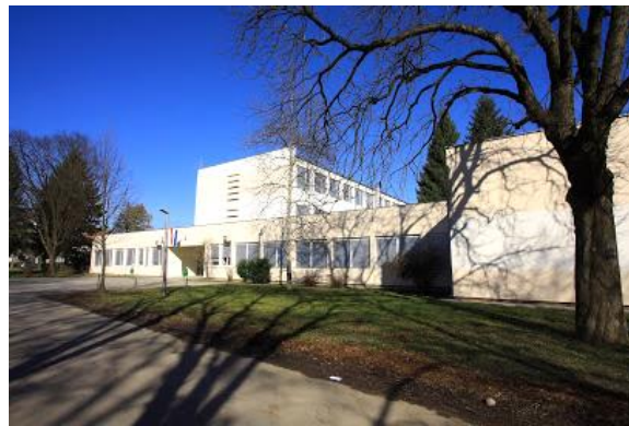
Figure 4.66. Faculty of Education before the earthquake (source: Google Earth).
