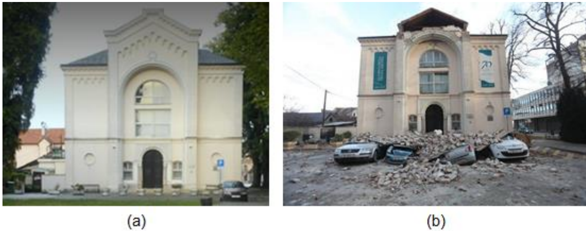
Figure 4.61. Fran Lhotka Music School (a) before the earthquake (source: Google Maps) and (b) after the earthquake (source: Facebook page - Glazbena škola Frana Lhotke, Sisak).
