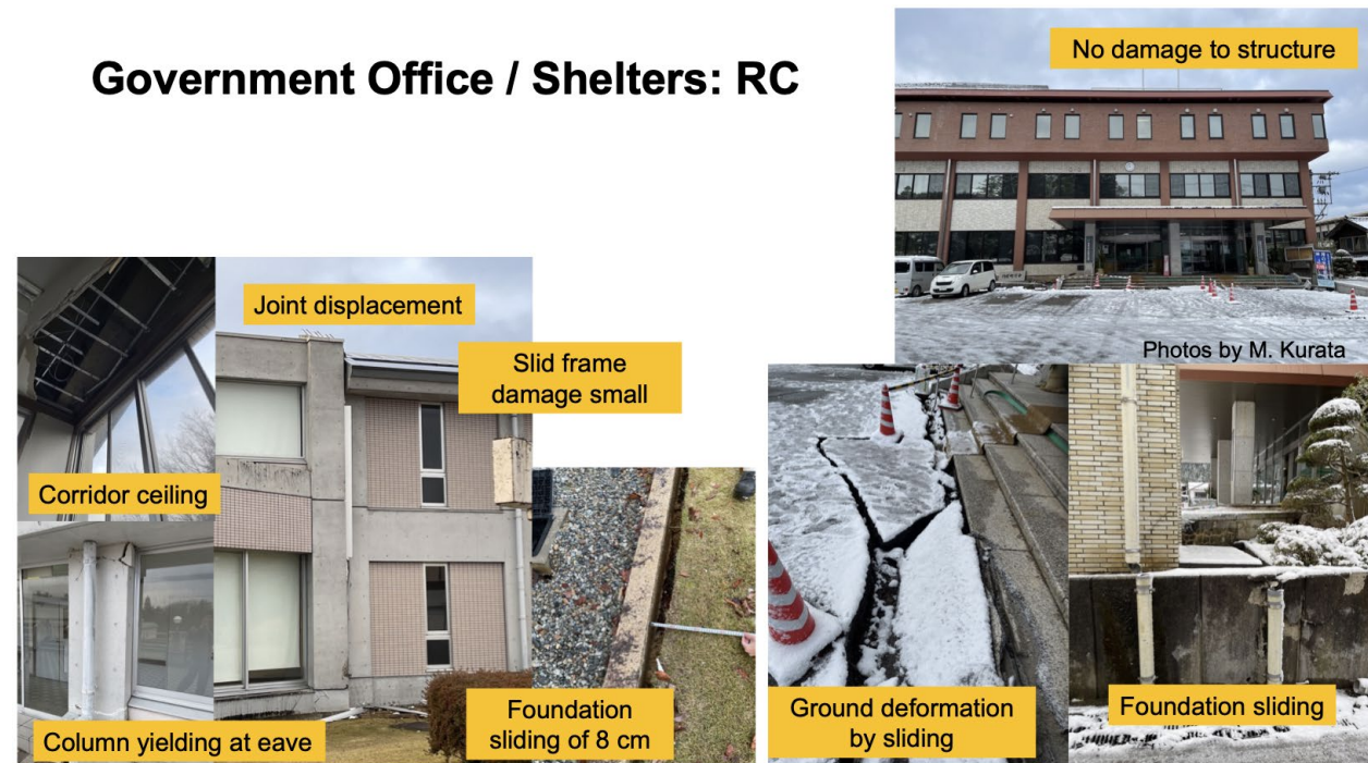
Figure 4.10. Government building and welfare facility (Credit: M. Kurata).
