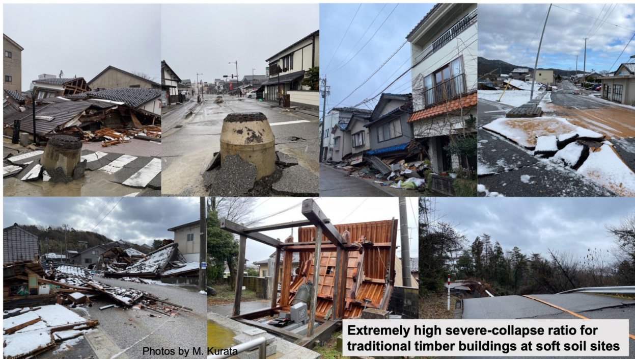
Figure 4.3. Traditional building damage at the affected sites (Credit: Kurata and Yamada).
