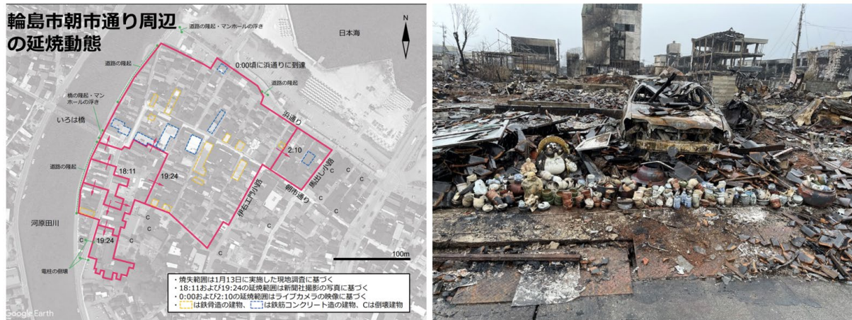
(a) Earthquake-triggered fire in Wajima city
