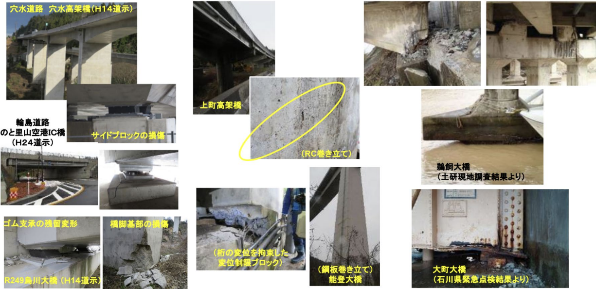
(a) New code conforming bridges (b) Seismically-retrofitted bridges (c) Unretrofitted bridges
