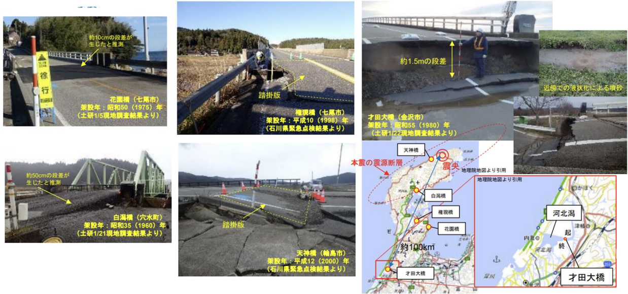
(a) Emergency restoration (b) Step slabs effective (c) Large step by liquefaction
