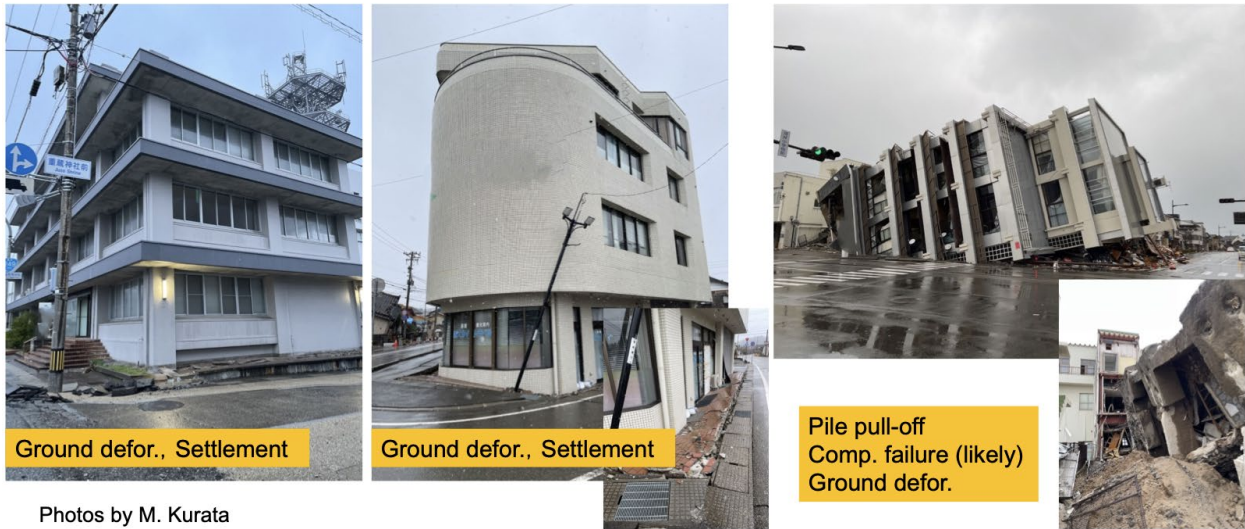
Figure 4.5. Damage to low-mid-rise RC buildings (Credit: M. Kurata).
