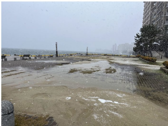
(a) Sand boiling and cracks in the ground
