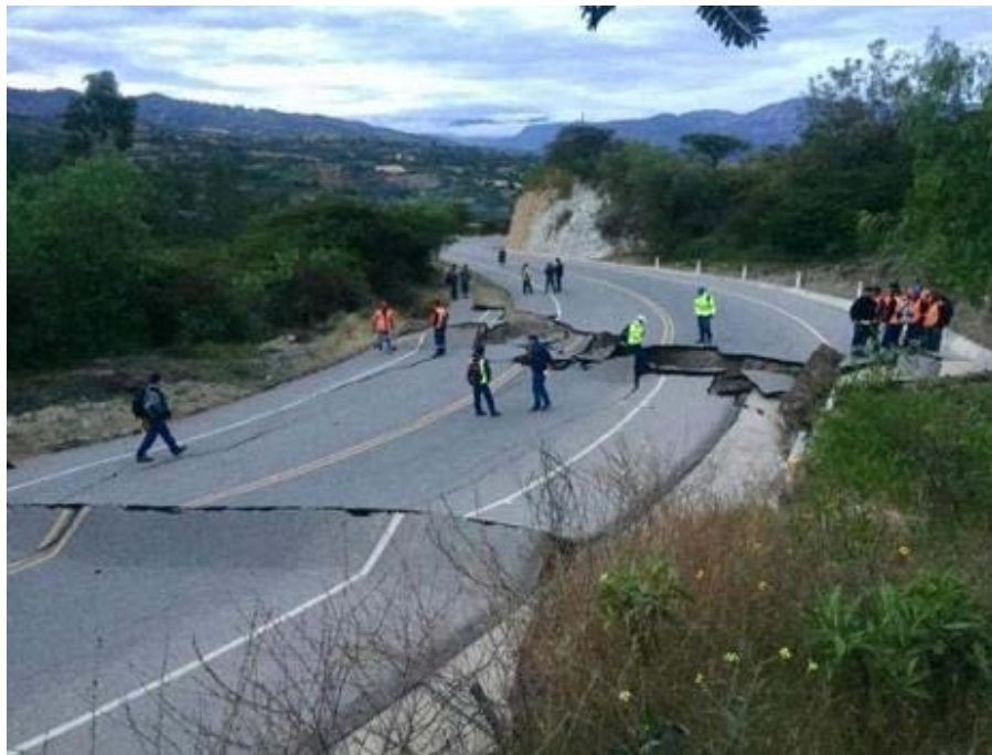
Figure 9.3. Cajabamba-Cajamarca road, close to Huañiamba (COEN, 2019).
