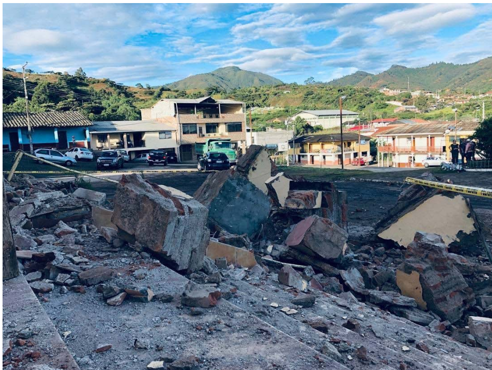
Figure 9.55. Bell tower of a church collapsed in Loja, Ecuador, at 490 km away from the epicenter (Trujillo, 2019).
