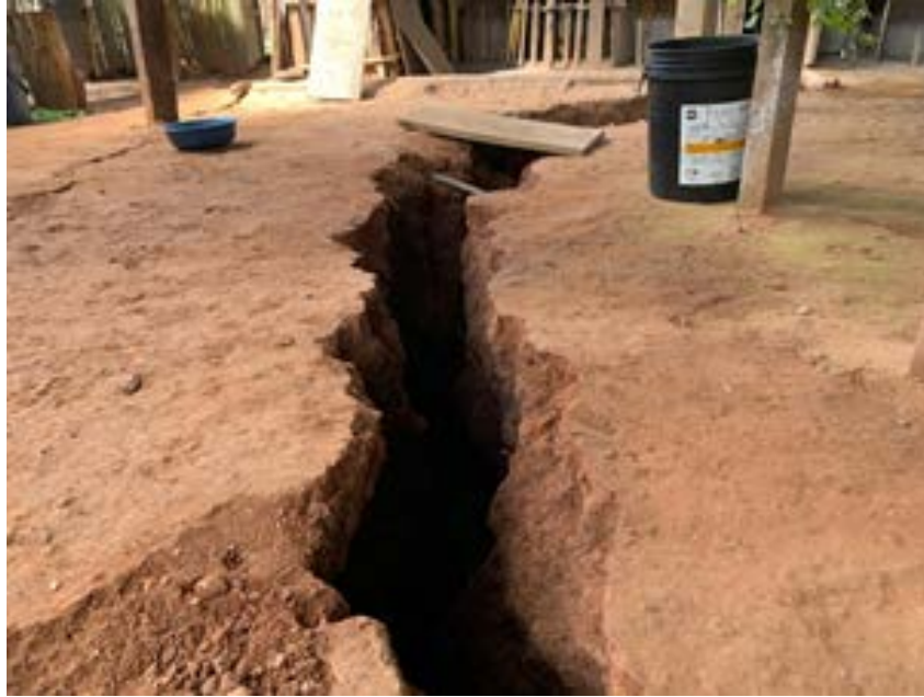
Figure 9.42. Apparent lateral spreading damage at the ground floor inside of a building at the 2 de Mayo village, Yurimaguas (Reategui and Mora, 2019).
