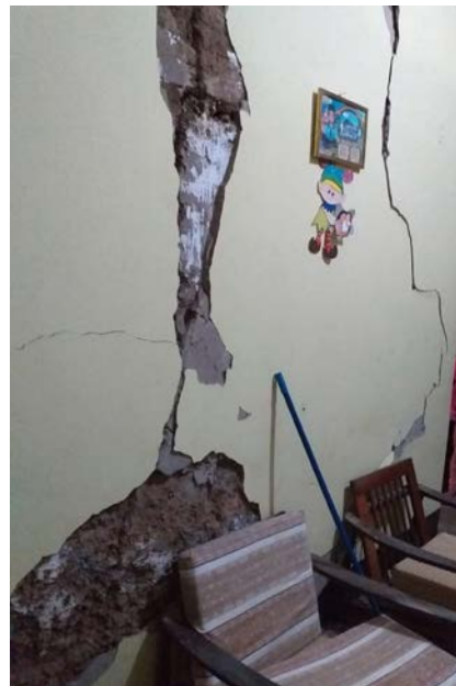
Figure 9.78. Plaster spalling and wall cracking in Lagunas, Loreto (Source: Rotafono [2]).
