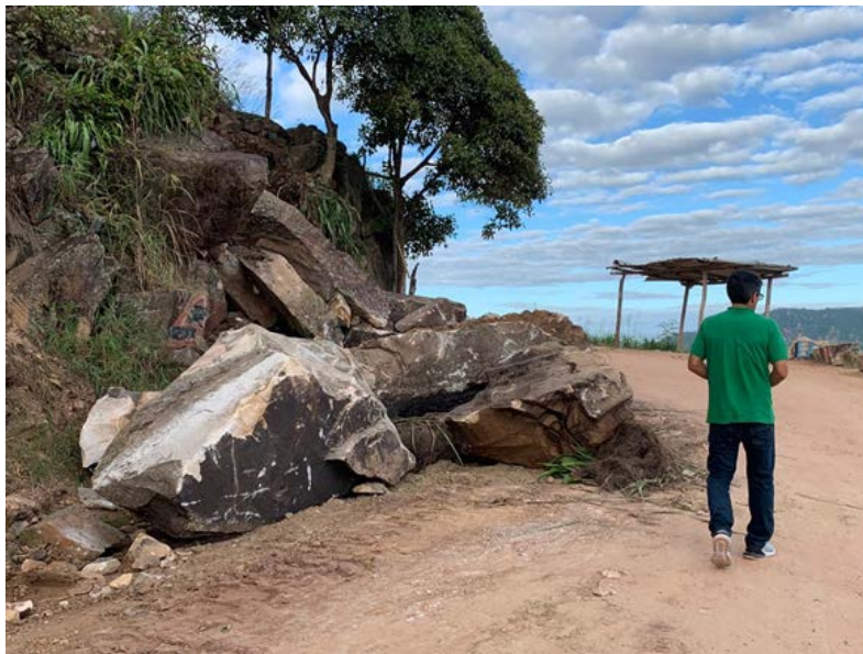
Figure 9.39. Rockfall at 2 de Mayo village (located at 1.5 hours from Tarapoto, Sauce district) (Reategui and Mora, 2019).
