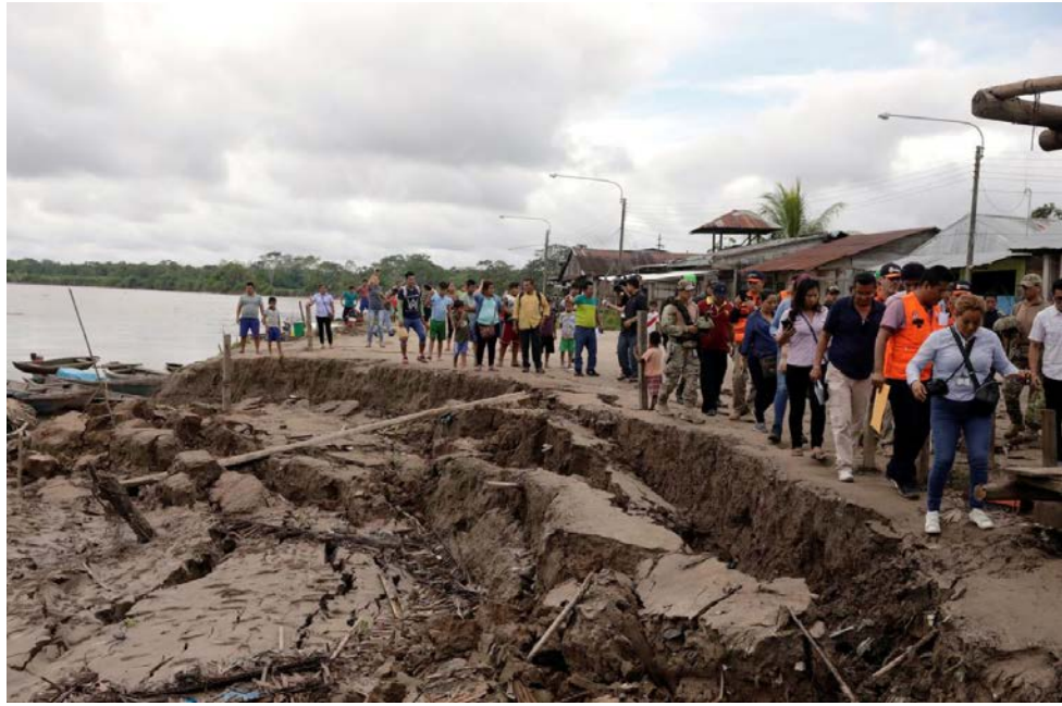
Figure 9.12. Lateral spreading along the Huallaga river at the Santa Gema near Yurimaguas in the Amazon region of Peru, (Jourdan et al. 2019).
