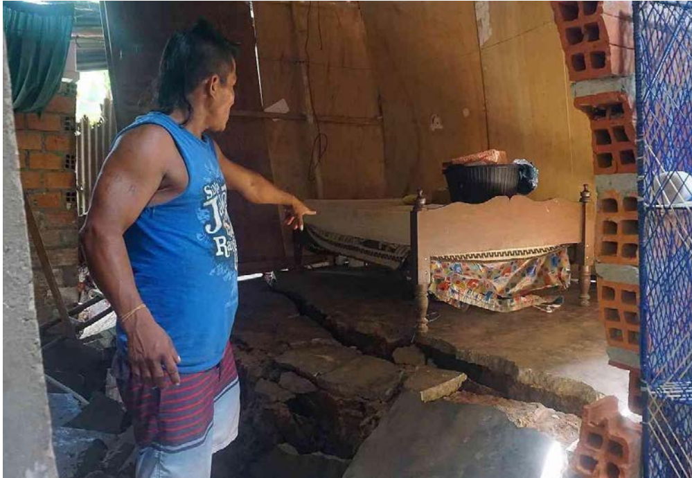
Figure 9.1. Ground failure inside family house in Alto Amazonas, Loreto (Source: AFP [3]).
