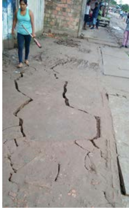
Figure 9.38. Huallaga pier at Lagunas with apparent lateral spreading effects (Source: @govanniacate via Twitter).
