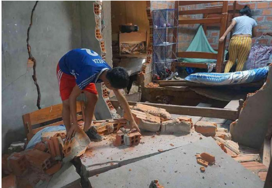
Figure 9.49. Out-of-plane failure of an interior hollow-clay brick masonry wall in Alto Amazonas, Loreto (Source: AFP [3]).
