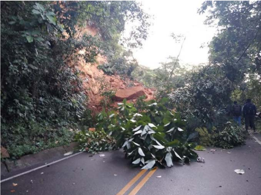
Figure 9.35. Yurimaguas-Tarapoto road, hill landslides (Source: @govanniacate via Twitter).
