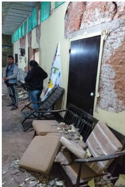
Figure 9.78. Plaster spalling and wall cracking in Lagunas, Loreto (Source: Rotafono [2]).
