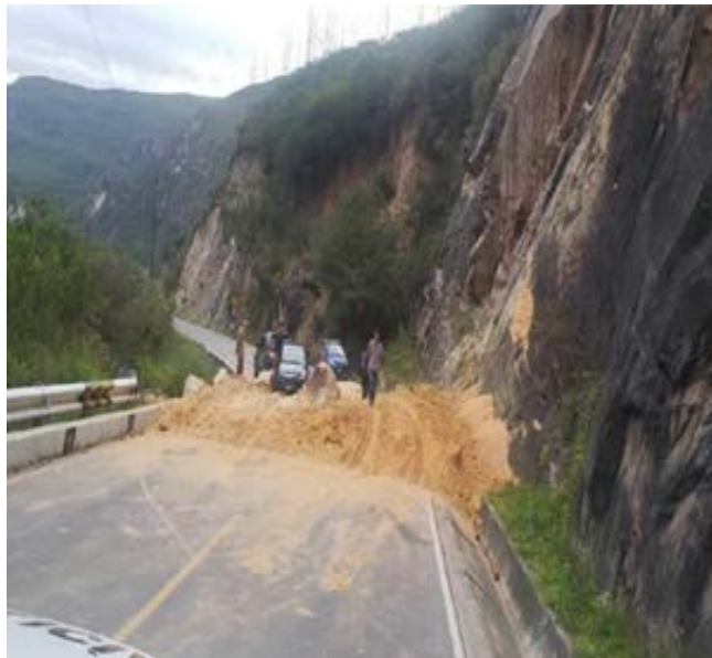
Figure 9.37. Landslides at the Leymebamba-Chachapoyas road, Ubillon sector, km 272+00, Amazonas (COEN, 2019).
