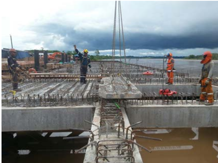
Figure 9.76. Port of Yurimaguas during construction (Source: Postensa SAC. Dr. Luis Bozzo).
