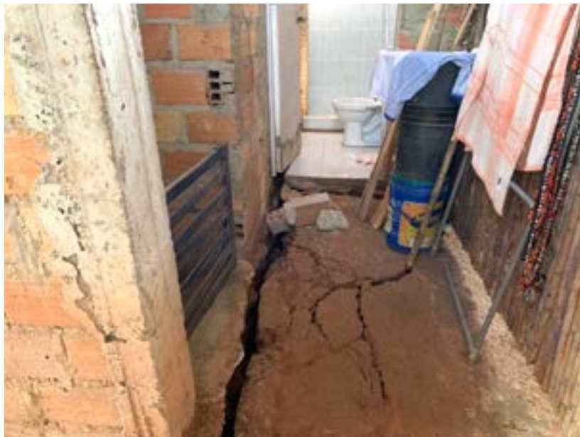
Figure 9.43. Apparent lateral spreading damage in buildings at the 2 de Mayo village, Yurimaguas (Reategui and Mora, 2019).
