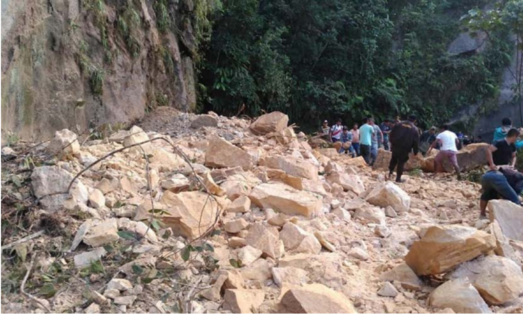
Figure 9.34. Yurimaguas-Tarapoto road, hill landslides (Source: @govanniacate via Twitter).
