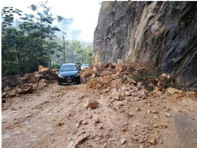
Figure 9.33. Yurimaguas-Tarapoto road, hill landslides (Source: @govanniacate via Twitter).
