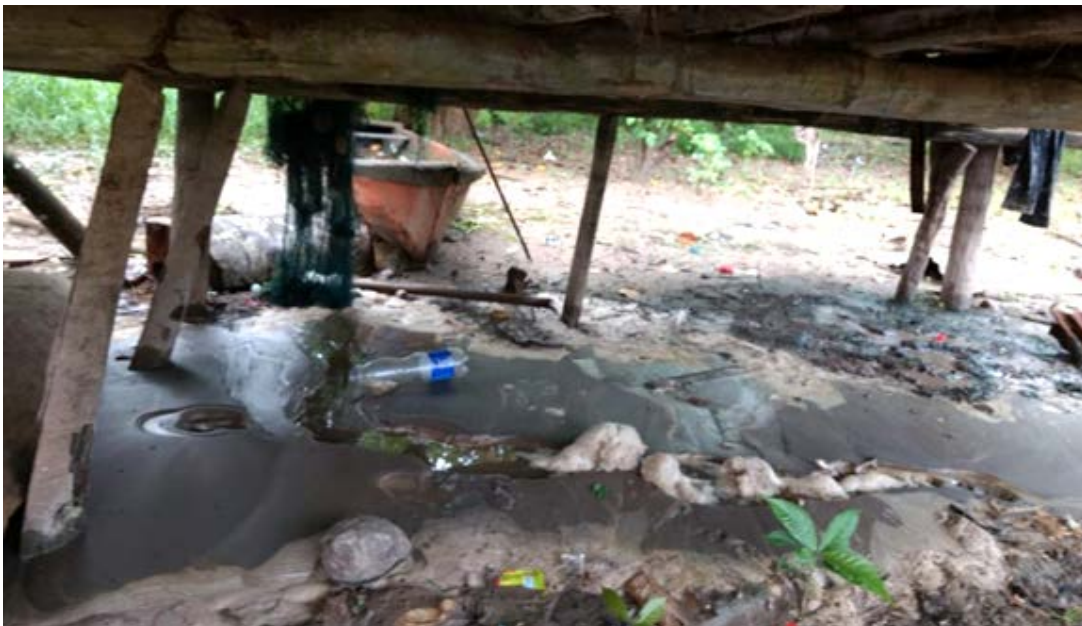
Figure 9.19. Liquefaction ejecta under a house built on wooden piles in district of Lagunas in Alto Amazonas, 145 km away from epicenter, Loreto Region. (Source: Perú 21).
