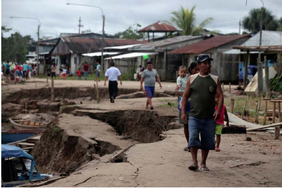
Figure 9.14. Lateral spreading along the Huallaga river at the Santa Gema near Yurimaguas in the Amazon region of Peru, (Jourdan et al. 2019).
