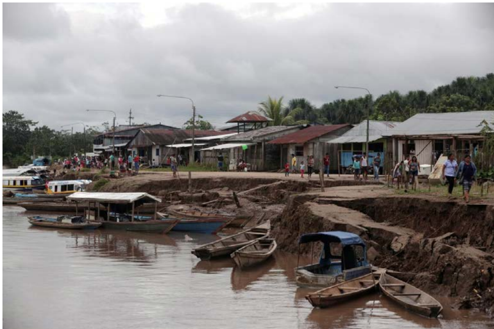
Figure 9.13. Lateral spreading along the Huallaga river at the Santa Gema near Yurimaguas in the Amazon region of Peru, (Jourdan et al. 2019).
