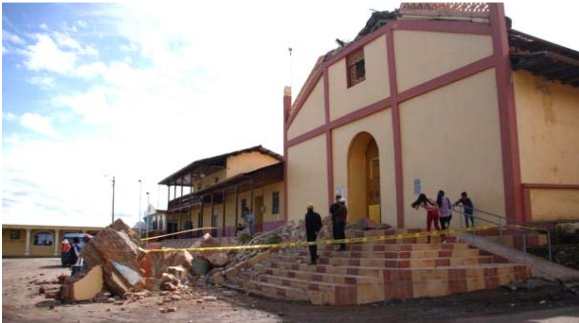
Figure 9.55. Bell tower of a church collapsed in Loja, Ecuador, at 490 km away from the epicenter (Trujillo, 2019).
