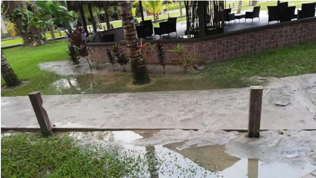
Figure 9.24. Liquefaction ejecta in El Sauce Resort, Tarapoto (Source: Rotafono [2]).
