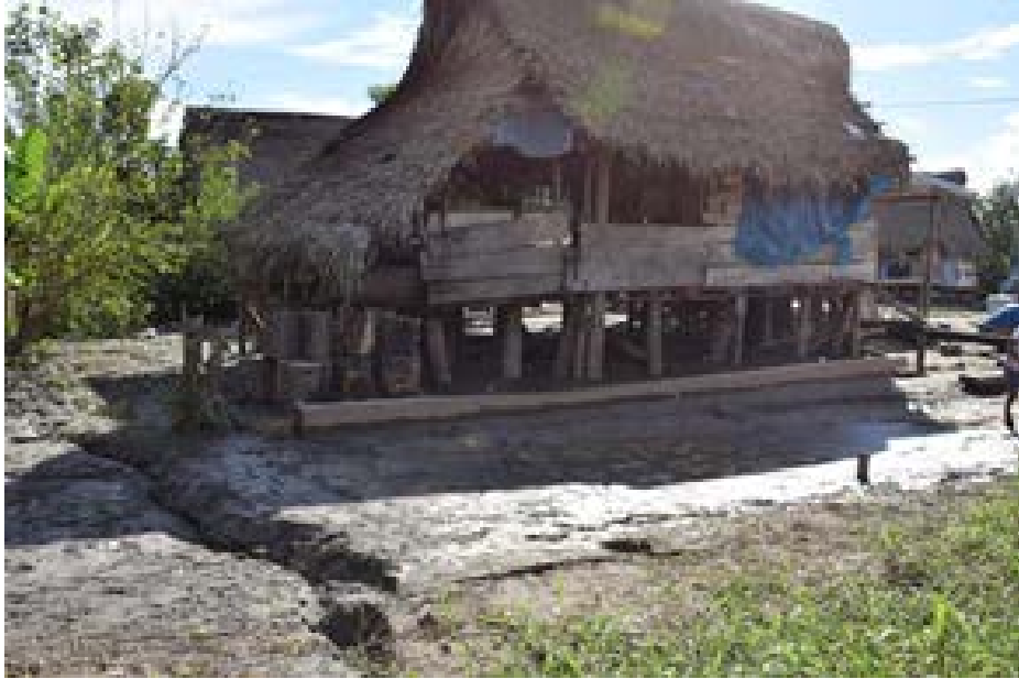
Figure 9.30. Seismically-induced ground damage due to liquefaction and lateral spreading at El Sauce District (Source: Ministerio de Vivienda del Perú - Photo by Miguel Estrada).
