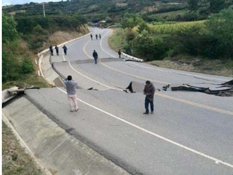
Figure 9.2. Cajabamba-Cajamarca road, close to Huañiamba (COEN, 2019).
