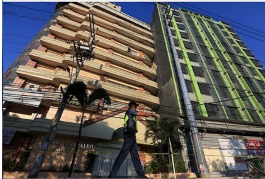
Figure 6. Tilted 10 story school building in Manila
