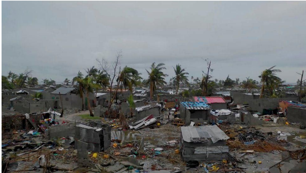
Figure 5: Damage to non-engineered housing units consisting of adobe/timber walls and sheet metal roofing (Photo Credit: Reuters)
