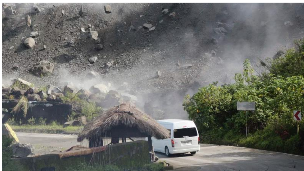
Figure 4. Earthquake rockslides resulting in road blockages (NPR, 2022).
