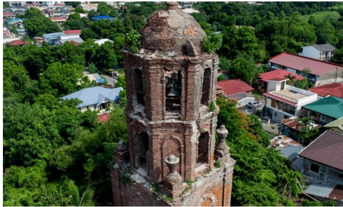
Figure 7. Damage to the Bell Tower in Bantay, Ilocos Sur (Twitter, 2022b; Dawn, 2022).
