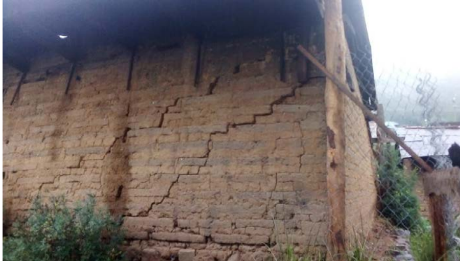
Figure 7.4. Severe diagonal tension cracking in a wall of an adobe house, Oaxaca (Its going down, 2020).
