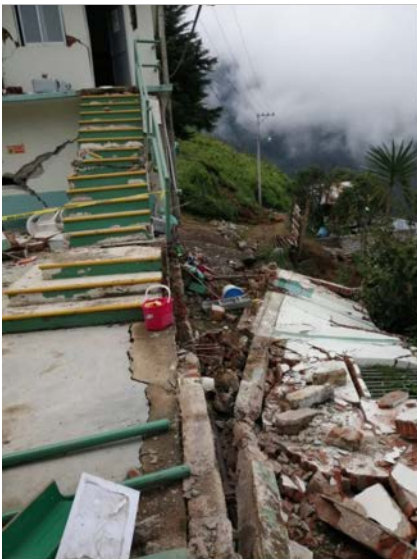
Figure 7.18. Failure of unreinforced masonry wall of the medical unit located at Santa Catarina Xanaguía in the San Juan Ozolotepec municipality, Oaxaca (Twitter, 2020I).
