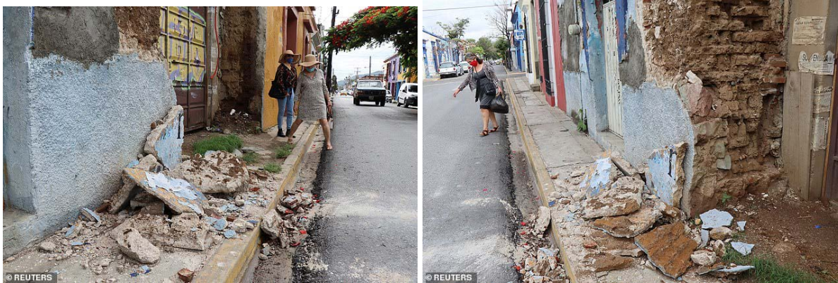
Figure 7.15. Failure of masonry walls and spalling of plaster in Oaxaca (Distinct Today, 2020).
