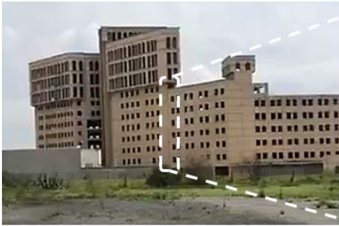
Figure 8.4. Damage produced by pounding at Hotel Miled located in the Metepec municipality, Mexico State (QuieroTV, 2020).
