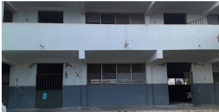
Figure 4.18. Short column effect due to partial height infill walls in Sinai National School in Miragoane (Source: Gefthe Devilmé, GeoHazards International)
