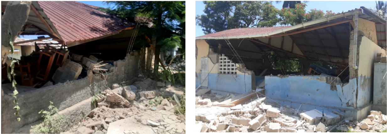
Figure 4.20. Public secondary school collapsed in Petit Trou de Nippes (Source: Twitter ).
