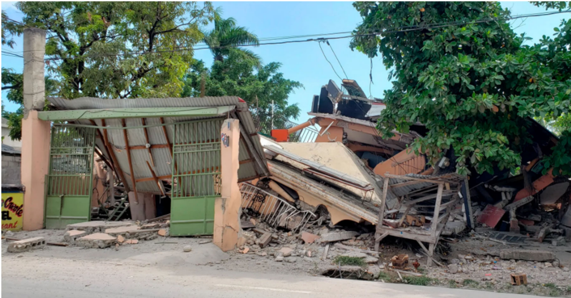
Figure 4.10. Cayimite Hotel collapsed in Les Cayes, Haiti, Aug. 14, 2021 (Source: US today ).
