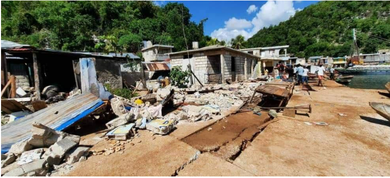
Damaged houses in the commune of Pestel, Corail Arrondissement, Grand'Anse Department (Source: Twitter )
