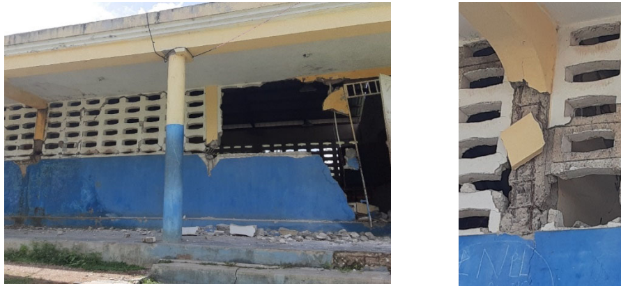
Figure 4.18. Short column effect due to partial height infill walls in Sinai National School in Miragoane (Source: Gefthe Devilmé, GeoHazards International)
