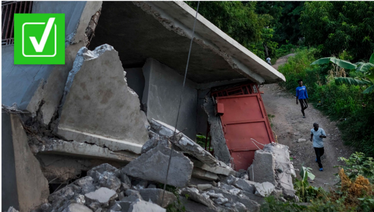
Collapsed building in Saint-Louis-du-Sud (Credit: AP )
