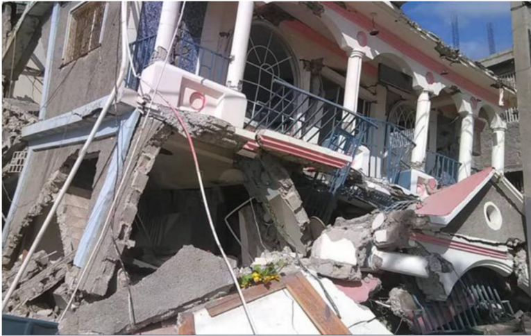
Collapsed hotel in Les Cayes (Source: Twitter )
