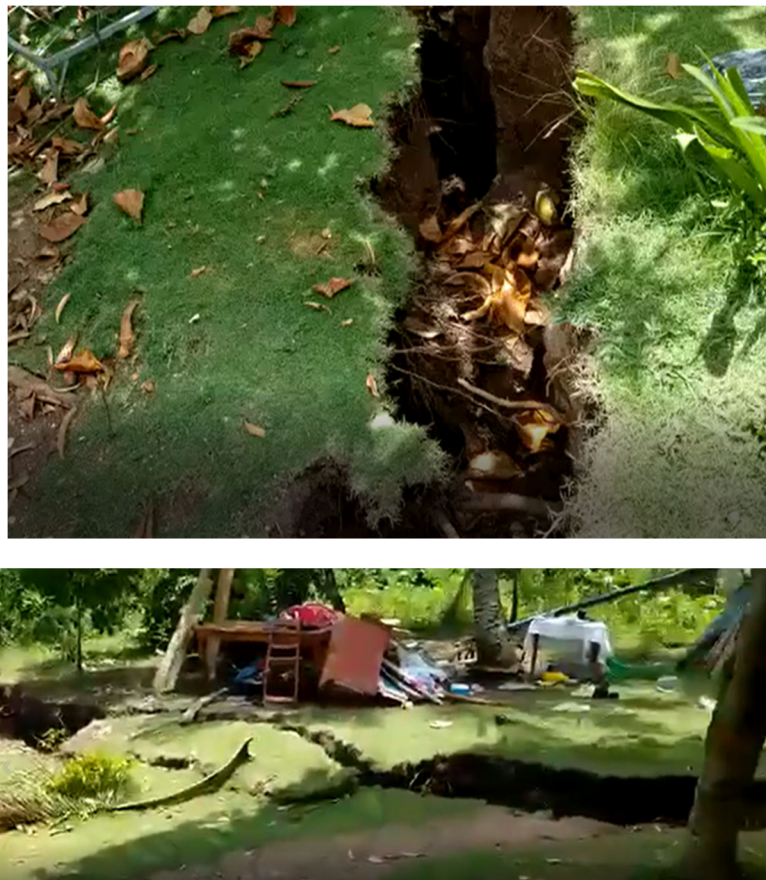
Figure 6.2. Stills from an amateur video showing the apparent top of a landslide in L'Asile (Source: Michael Wilson, direct communication).
