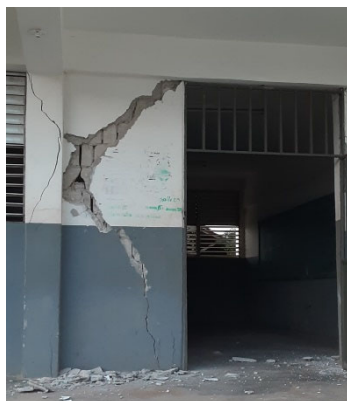
Figure 4.19. Infill wall damage and short column shear cracks at Boisrond Tonnerre school, Anse-a-Veau, Nippes Department (Source: Gefthe Devilmé, GeoHazards International)
