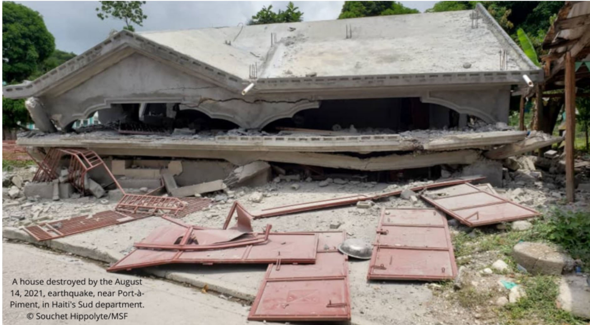
Figure 4.5. Pancake collapse of a weakly-confined masonry house destroyed in Port-à-Piment in the Sud Department (Source: Twitter ).
