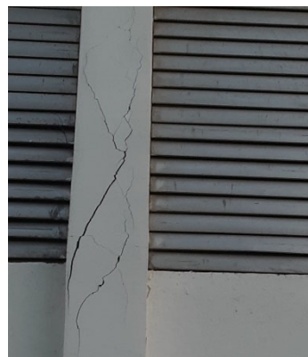
Figure 4.19. Infill wall damage and short column shear cracks at Boisrond Tonnerre school, Anse-a-Veau, Nippes Department (Source: Gefthe Devilmé, GeoHazards International)
