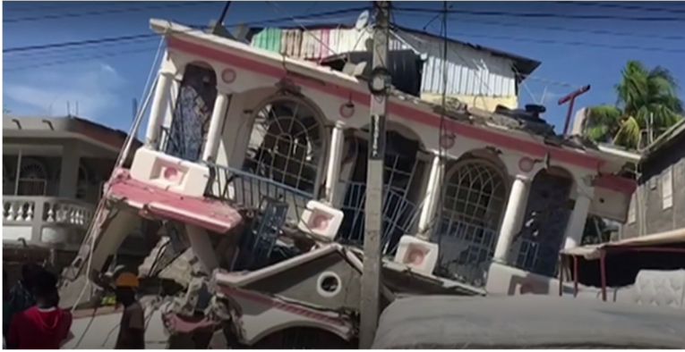
Collapsed hotel in Les Cayes front view (Source: Still photo of footage by Ralph Tedy Erol/AP, Source: NY Times )
