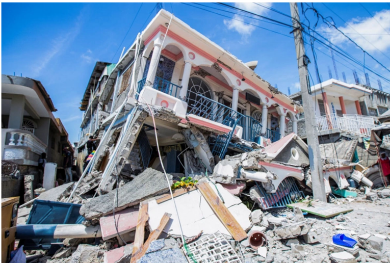
Collapsed Hotel Les Cayes (Source: Ralph Tedy Erol/AP, Source: Aljazeera )
