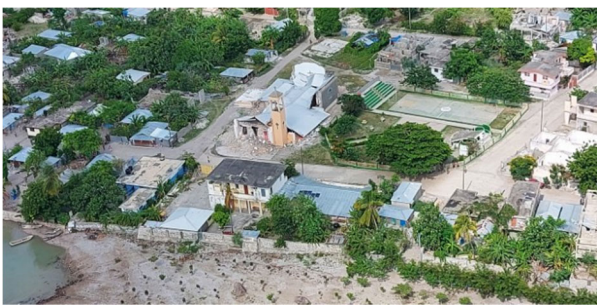
Collapse of the church of Saint Anne in Chardonnières, Sud Department (Source: USA Today )
