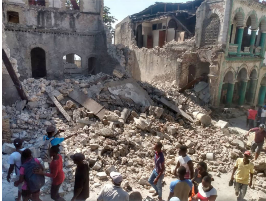
Figure 4.23. Collapse of stone masonry historical buildings, downtown Jeremie (Source: CNN ).
