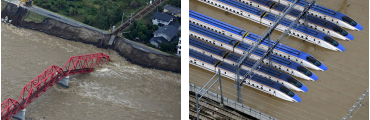
Figure 10: Damage to a railway bridge and high-speed trains (Source: Forbes, 2019).
