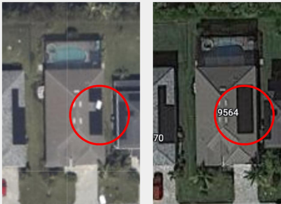
Figure CS5.2. Evidence of roof solar panel damage by comparing (left) a damaged panel visible in the post-storm NOAA imagery, and (right) pre-event imagery showing the undamaged panel.
