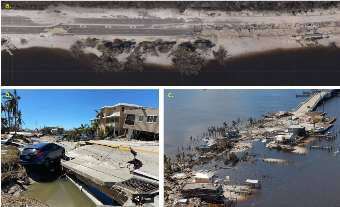
Figure 5.3. Observed damage coastal roadways, including (a) the McGregor Blvd in Fort Myers (source: NOAA Hurricane Ian Imagery), and (b), (c) the Pine Island Rd (Source: ABC news (2022) and Levy (2022) respectively).
