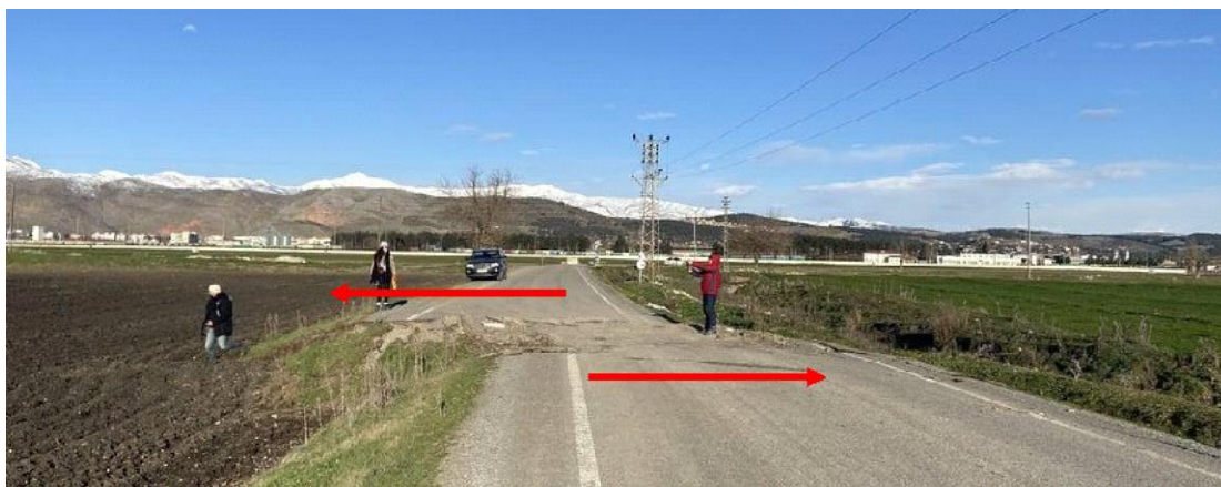
Figure 2.8. Fault slip of 3.0 to 3.5 m at the Anatolian plate from the February 6, 2023 earthquake sequence (adapted from reddit post by u/kebabG 2023a , last accessed 2-20-2023).
