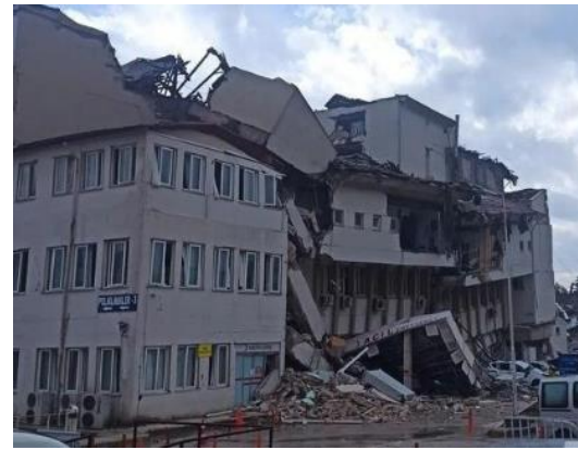
View of the northeast side of the collapsed facility (Source: Twitter ).
