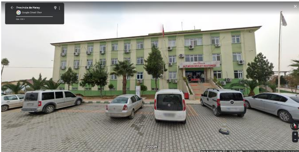
Figure 4.61. Pre-earthquake view of Altinozu State Hospital, Hatay province, 36.1120N 36.2437E (Source: Google Street View ).
