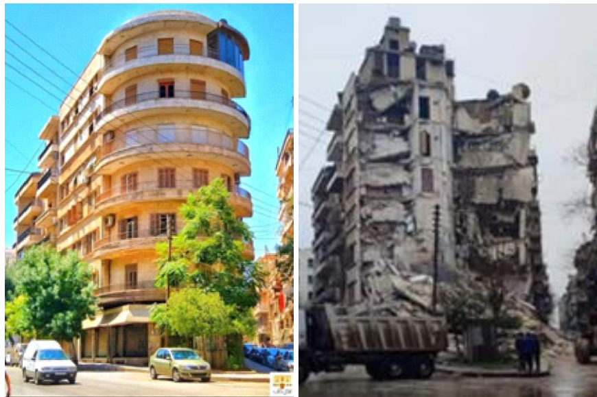
Figure 3.2. An Aleppo City mid-rise non-engineered building before and after the earthquakes, (Source: Salah Haj Ismail personal Archive).
