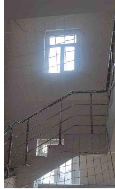
(a) Diagonal tension cracks of building exterior wall. (b) Crack parallel to stair run direction.
