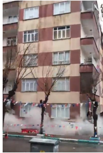
(a) Building prior to collapse. (b) Collapse of weak/soft story prior to gravity collapse.
