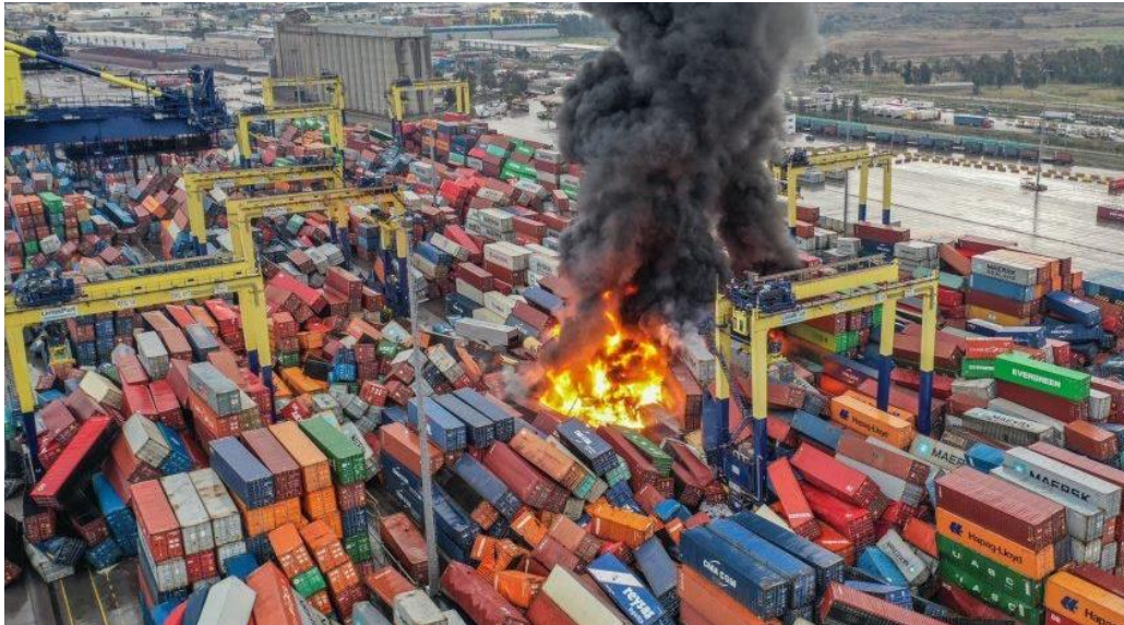
Figure 1.6. While gantry cranes appear unaffected by the earthquake, primary and secondary effects from fire after the earthquake compounded losses and downtime at the Iskenderun Port (Source: Odessa Journal ).
