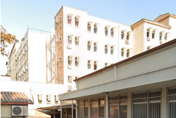
(a) Before the earthquake sequence (Source: Google Street View ).
