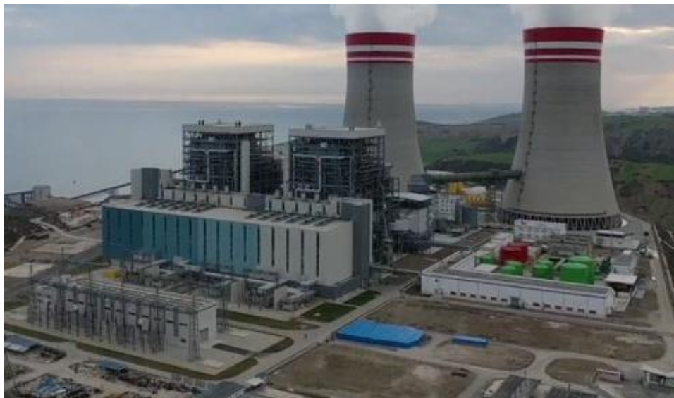
Figure 5.10. Undamaged Hunutlu thermal power plant in the Adana province (Source: Twitter ).
