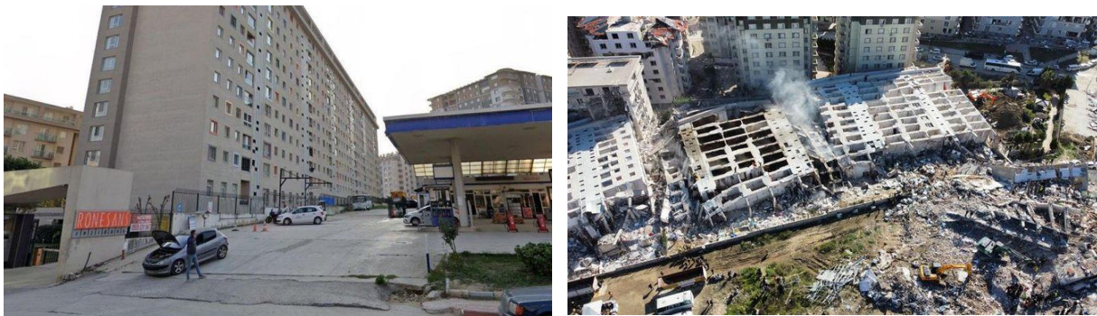
Figure 4.17. Potential sidesway collapse of the Rönesans residence, Hatay (Source: AFP via Middle East Eye ).
