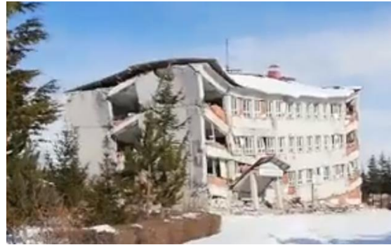
(b) Collapse after the earthquake sequence.
