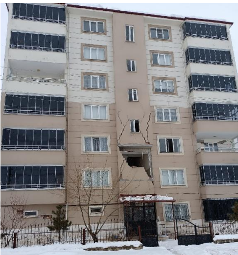
(a) Exterior walls.
