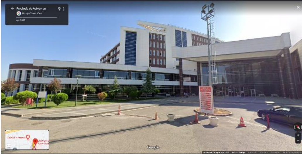
Figure 4.60. Pre-earthquake image of Adiyaman Training and Research Hospital, Adiyaman province, 37.7675N 38.3228E (Source: Google Street View ).
