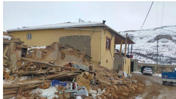
(b) Collapsed house.
