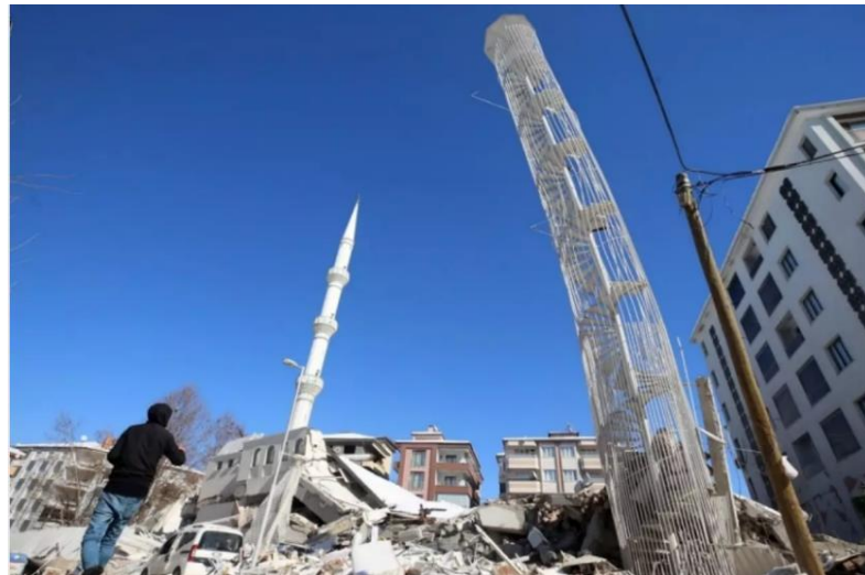
Figure 4.80. A 5-story RC building collapsed, but the steel stair stood alone, Malatya, Türkiye (Source: TRHaber 2023).
