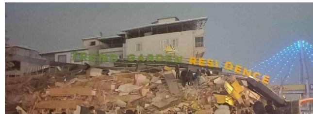
Figure 4.38. Before and after photographs of Trend Garden Residence showing the building collapse in Malatya, the pancake collapse of all stories suggests major structural problems. (38.347N 38.283E) (Source: NY Times ).
