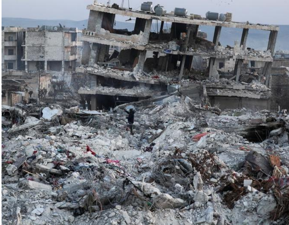
Figure 4.30. Collapsed building (foreground) and a partially collapsed RC building (background) in Jandires, Northern Syria (Source: Reuters ).
