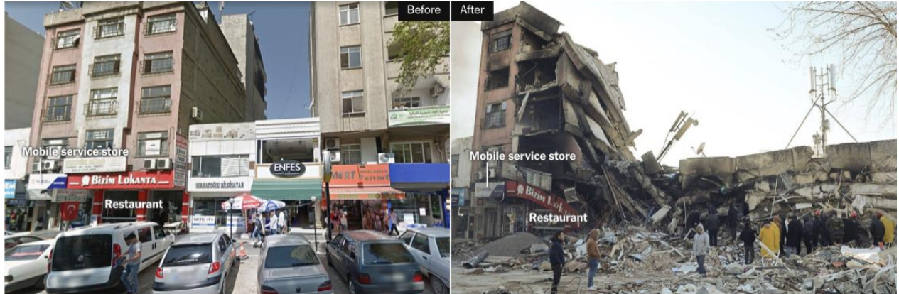
Figure 4.6. Collapse of buildings due to weak/soft story & pounding. The short 2-story building located between two mid-rise buildings, without adequate seismic separation, likely led to pounding between the roof slab of the 2-story building and the mid-height of the adjacent buildings. This has resulted in partial collapse of the building on the left and total collapse of the building on the right along with collapse of the 2-story (Source: New York Times 2023).
