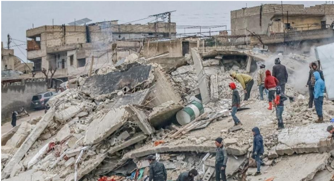
Figure 4.35. Collapsed concrete building near Idlib, Northern Syria. Notice the poor reinforcement of the columns (Source: AFP ).
