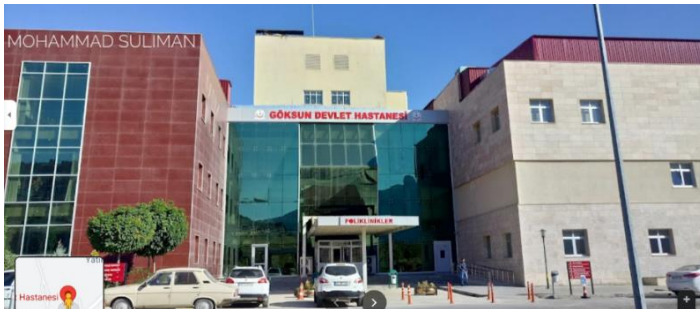
(a) Pre-earthquake ( Google Street View ).
