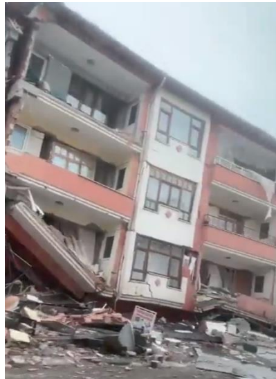
Figure 4.10. Soft-story collapse of residential buildings in different cities (Sources: The Insider Paper via Twitter & AlertaNews24 via Twitter ).
