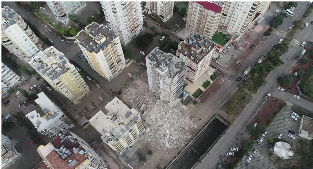
(c) Aerial View of collapsed building (Source: NTV 2023 ).
