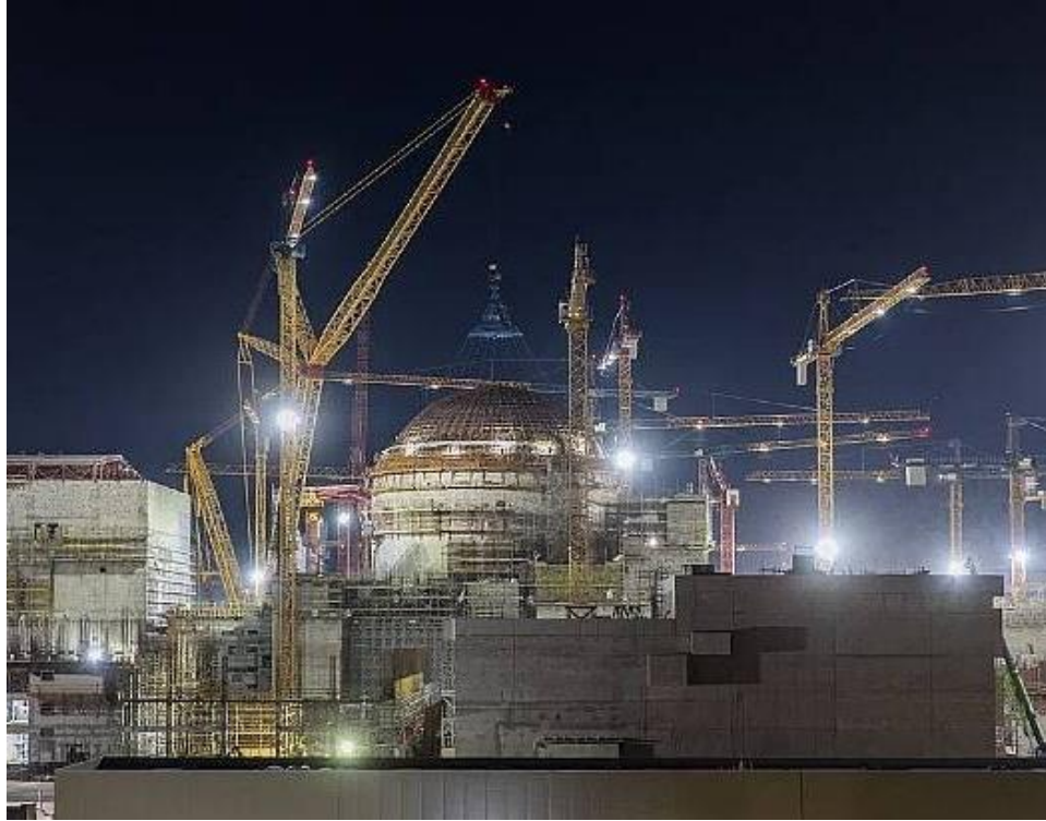
Figure 5.11. Undamaged Akkuyu nuclear power plant (Source: World Nuclear News ).
