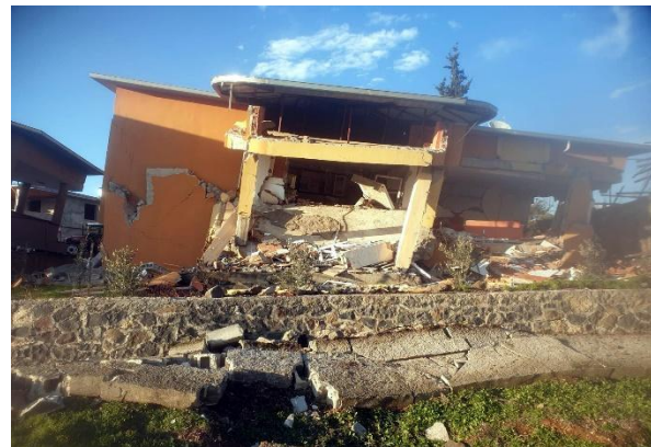
Figure 4.13. First story collapse of single-family RC residential buildings in Tevekkelli possibly due to weak and soft-story failures (Source: Veryansin TV 2023 ).
