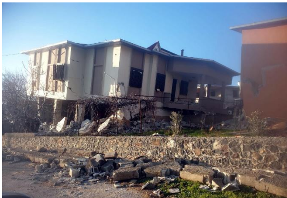
Figure 4.13. First story collapse of single-family RC residential buildings in Tevekkelli possibly due to weak and soft-story failures (Source: Veryansin TV 2023 ).
