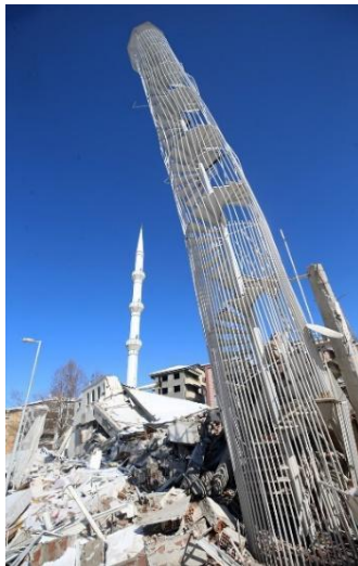
Figure 4.80. A 5-story RC building collapsed, but the steel stair stood alone, Malatya, Türkiye (Source: TRHaber 2023).
