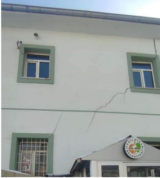
(a) Diagonal tension cracks of building exterior wall. (b) Crack parallel to stair run direction.
