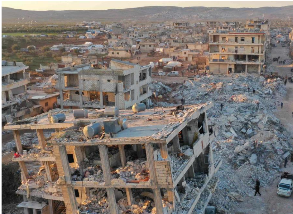
Figure 4.31. Collapsed buildings in Harem, Reef Idlib, Northern Syria (Source: wsiu.org 2023).
