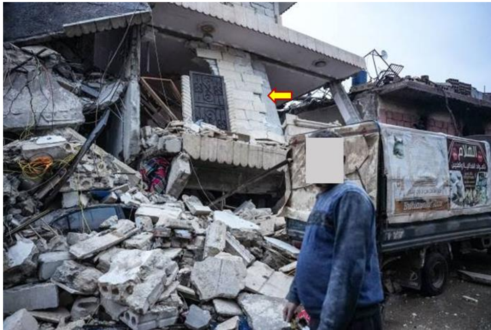
Figure 4.22. Collapse of a multi-family low-rise unreinforced masonry building in Aleppo (Source: Getty Images ).
