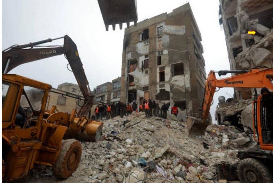
Figure 4.24. Ruins of a collapsed building with severely damaged RC columns (shown with arrows) in the adjacent building, Hama (Source: LOUAI BESHARA/AFP, Getty Images ).
