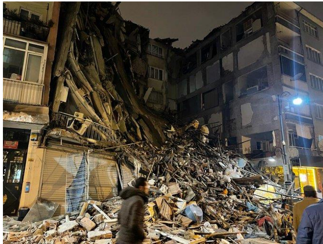
Figure 4.5. Ruins of a collapsed building showing no seismic gap between adjacent buildings, Malatya (Source: Darkwebhaber via Twitter ).
