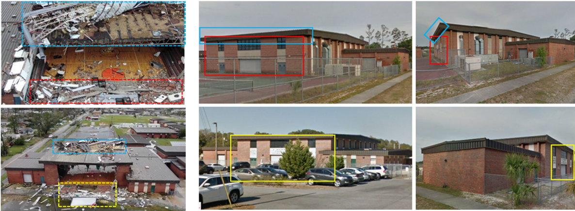
(a) After hurricane Michael
