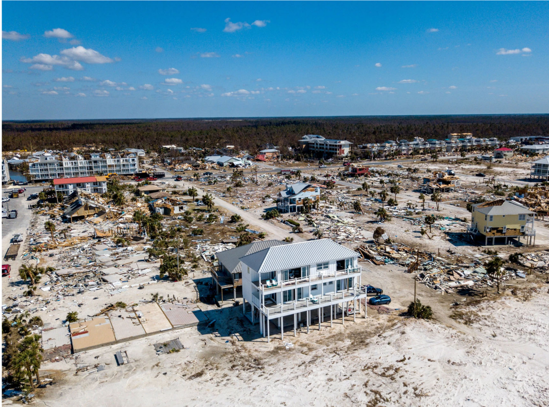
Figure 16: Widespread devastation to wood-framed single and multi-family residences in Mexico Beach as noted by the bare slabs with few survivors in the areas with highest inundation, including the concrete “Sand Palace” (Source: New York Times)
