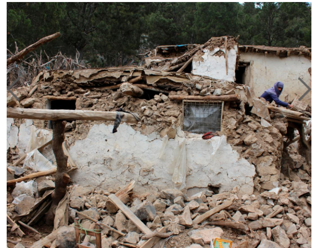
Figure 5. Collapsed masonry and earthen homes in Paktika & Khost provinces (Popalzai et al., 2022; Noroozi, 2022).
