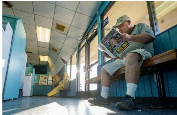
Figure 14. (a) The Daily Independent Newspaper office ceiling damaged during the M 6.4 event (Jessica Watson, AP); (b) Suspended ceiling partial failure at a laundromat in Ridgecrest after the M 6.4 event (Photo by Terry Pierson, The Press-Enterprise/SCNG)
