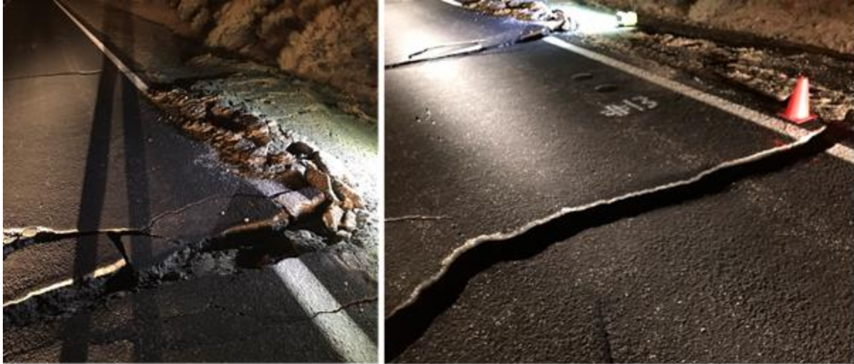
Figure 49. SR 178 near PM (post mile mark) 8.5 Caltrans crews making repairs to patch road before open to traffic 57 (picture taken 12:53am 07/06/2019)
