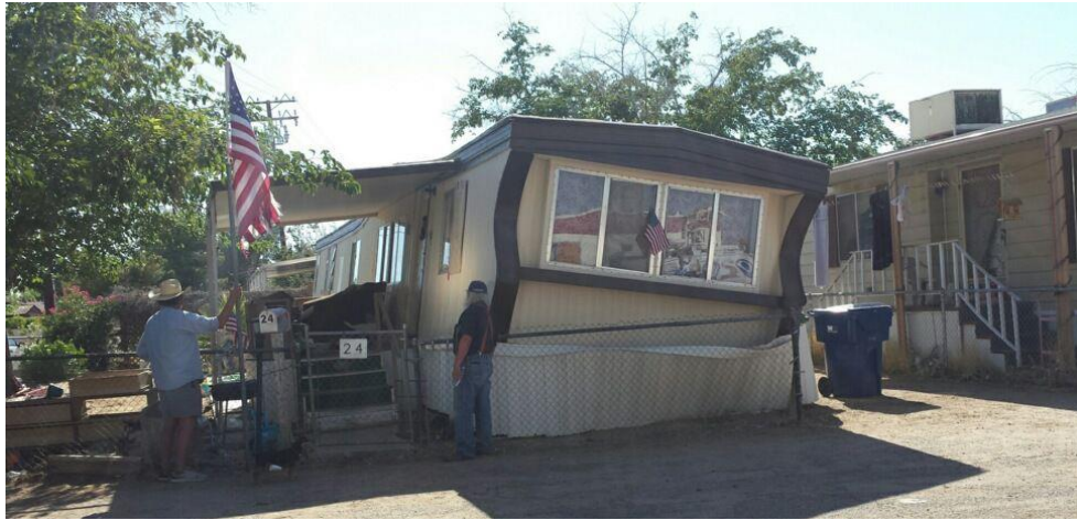
Damaged mobile home in Ridgecrest, CA during the M 6.4 earthquake. Photo by Darla A. Baker / The Californian .
