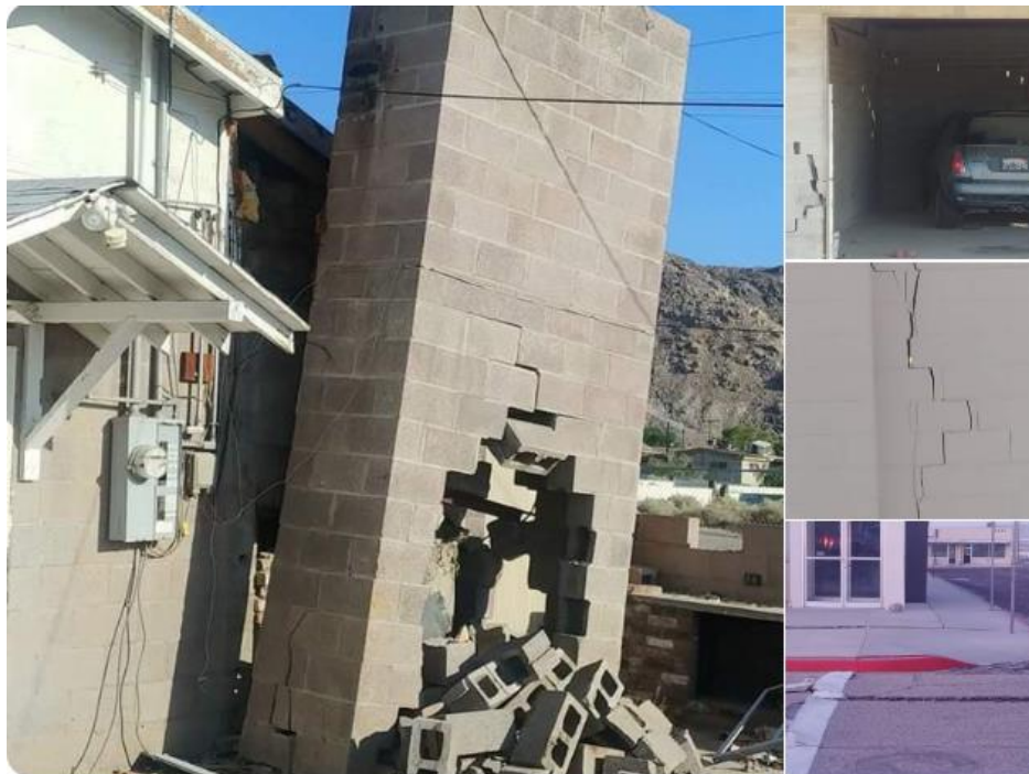
Figure 20. Damage to a masonry house in Trona after the M 7.1 earthquake (Source: Eytan Wallace via Twitter)
