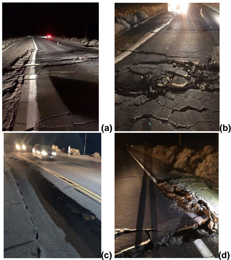
Figure 33. (a) Several cracks on the SR 178 WS between Trona and Ridgecrest after the M 7.1 event. The road was closed for repairs; (b) Details of the cracks 26 ; (c) Other picture of the cracks 27 ; (d) Rockfall cleared on SR 178 between Trona and Ridgecrest but route still closed for temporary repair 28
