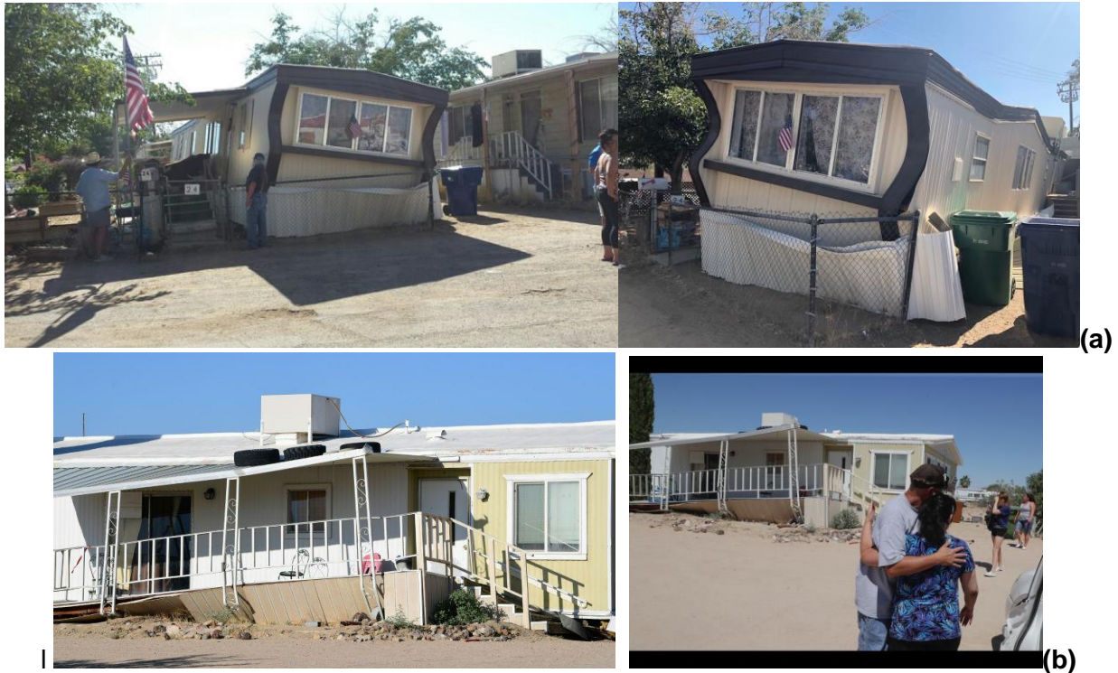
Figure 26. Damage to mobile homes in Ridgecrest area due to the M 6.4 event (a) Source: Bakersfield News, 2019; (b) Source: Yahoo News, 2019
