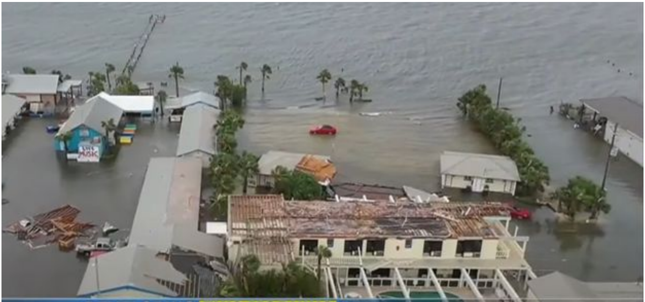
Figure 3.5. Structural roof damage at the Paradise Inn hotel in Pensacola, FL (Source: CBS This Morning www.youtube.com )
