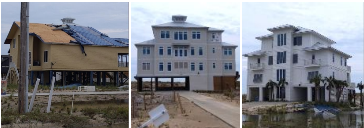
Figure 4.4. Typical damage observed in Gulf Shores: (a) significant loss of roof cover; (b) no loss of roof cover, but minor loss of cladding; (c) no observed damage.
