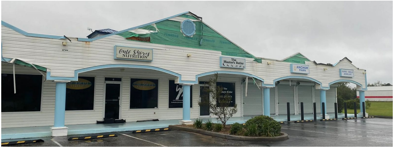
Figure 3.2. Loss of siding on strip mall in Gulf Shores, AL (Source: https://globalnews.ca/ )
