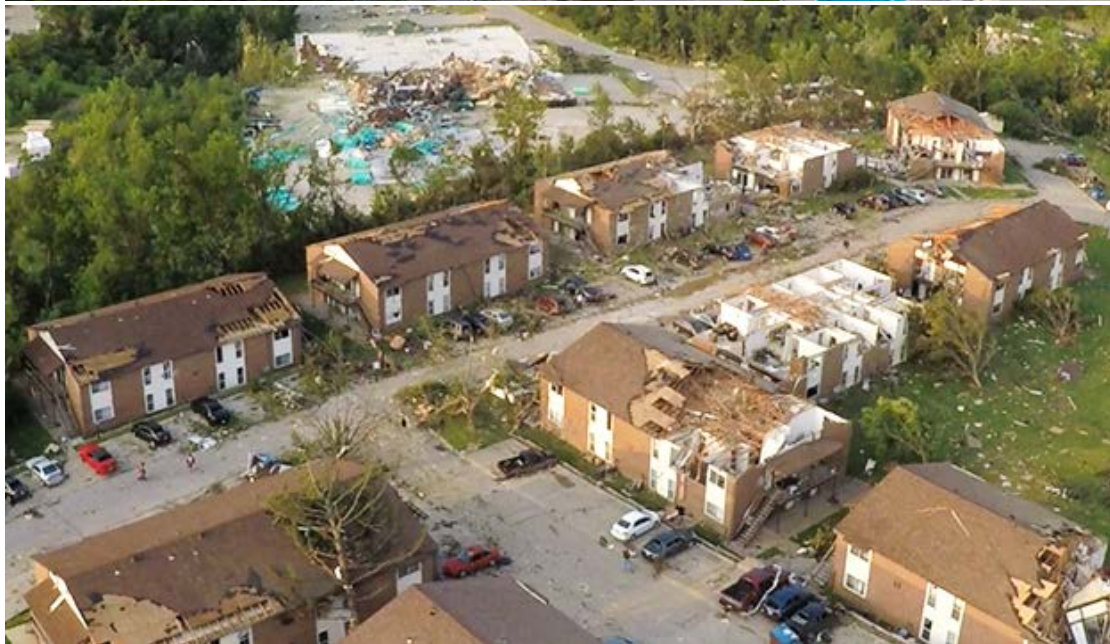
Fig. 1 Drone photos of the Hawthorne Park Apartment Complex.
