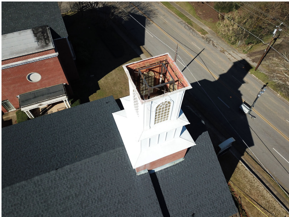
Figure 5. (a) Damaged roof structure on main campus building MC1 campus and (b) loss of steeple on main campus building MC2 at the First Baptist Church Wetumpka campus. It is clear the steeple lacked structural connections because the remaining structure is lightly damaged.
