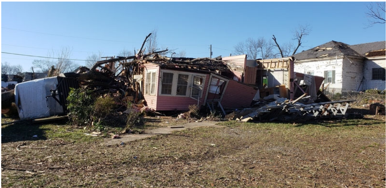
Figure 14. Partially collapsed single family home in Wetumpka, AL.
