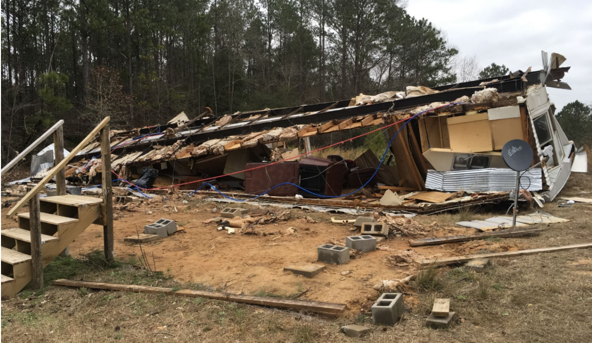
Figure 22. Single-wide mobile home rolled over due to tornado, injuring 2 people. (Source: https://www.weather.gov/bmx/event_01192019booth )
