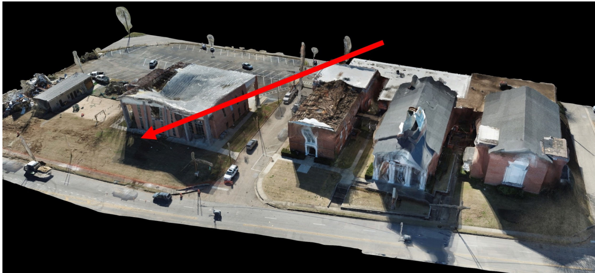
Figure 4. Pre-tornado birds-eye view of the FBC campus with individual buildings annotated (top); post-tornado birds-eye view of the FBC campus based on preliminary processing of UAV photos using Structure-from-Motion techniques. Approximate direction and location of tornado path centerline is indicated by the red arrow.
