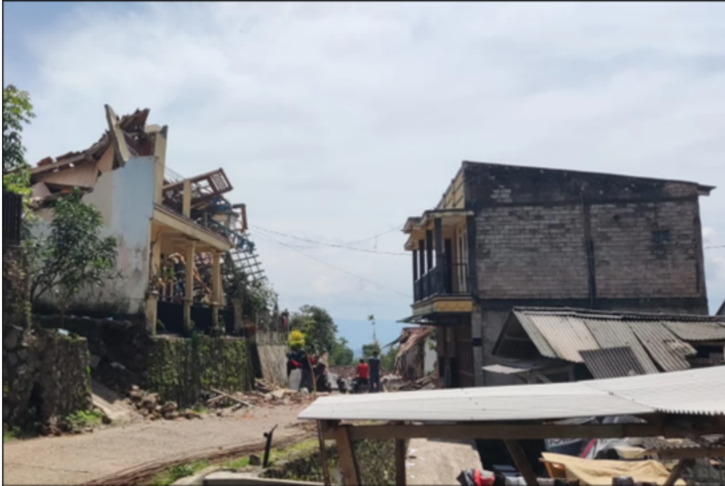
Figure 4.4 – A collapsed building next to a survived building (Project Hope, 2022).
