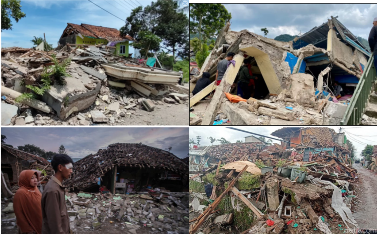
Figure 4.2 – Pancake collapses (Project Hope, 2022; BBC, 2022a; tirto.id, 2022; Fadhillah, 2022).
