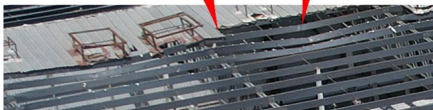
Figure 4.3.1. Damage to Multiplaza las Palmas; (top) before Hurricane Otis (Source: Google Street View); (middle and bottom) after Hurricane Otis (Source: FAST)
