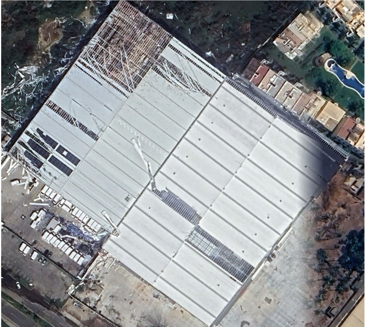
Figure 4.3.5. Bimbo Distribution Center, including Warehouse 1 on the left and Warehouse 2 on the right (Source: Google Earth).
