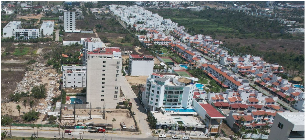
Figure 4.1.14. Overall view of buildings inland from Clusters 13 and 15 (Source: FAST).
