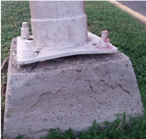
Figure 4.4.2. Brittle damage of public lightning poles, including rotation of foundation and out-of-plane base plate bending (Source: FAST).
