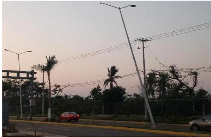
Figure 4.4.2. Brittle damage of public lightning poles, including rotation of foundation and out-of-plane base plate bending (Source: FAST).
