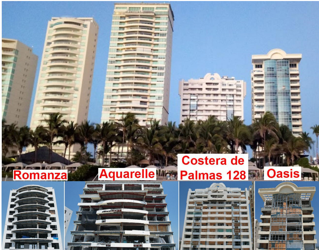
Figure 4.1.7. Cluster 13 SW elevation seaward views; (top) before Hurricane Otis (Source: Google Street View); (bottom) after Hurricane Otis (Source: FAST).
