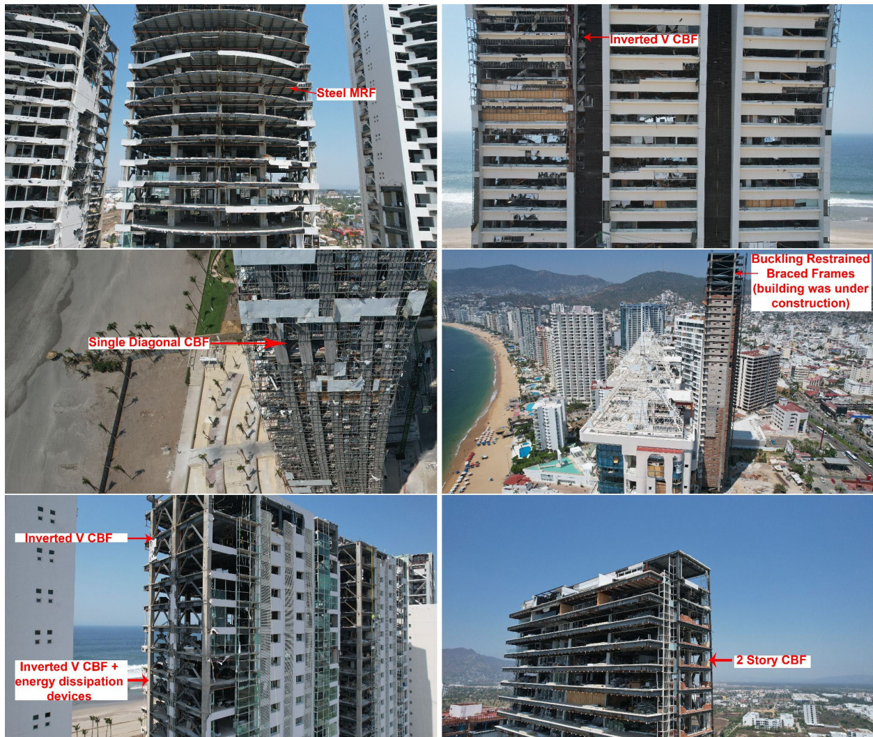
Figure 4.1.2. Examples of LFRS with Composite Columns in Acapulco (Source: FAST).
