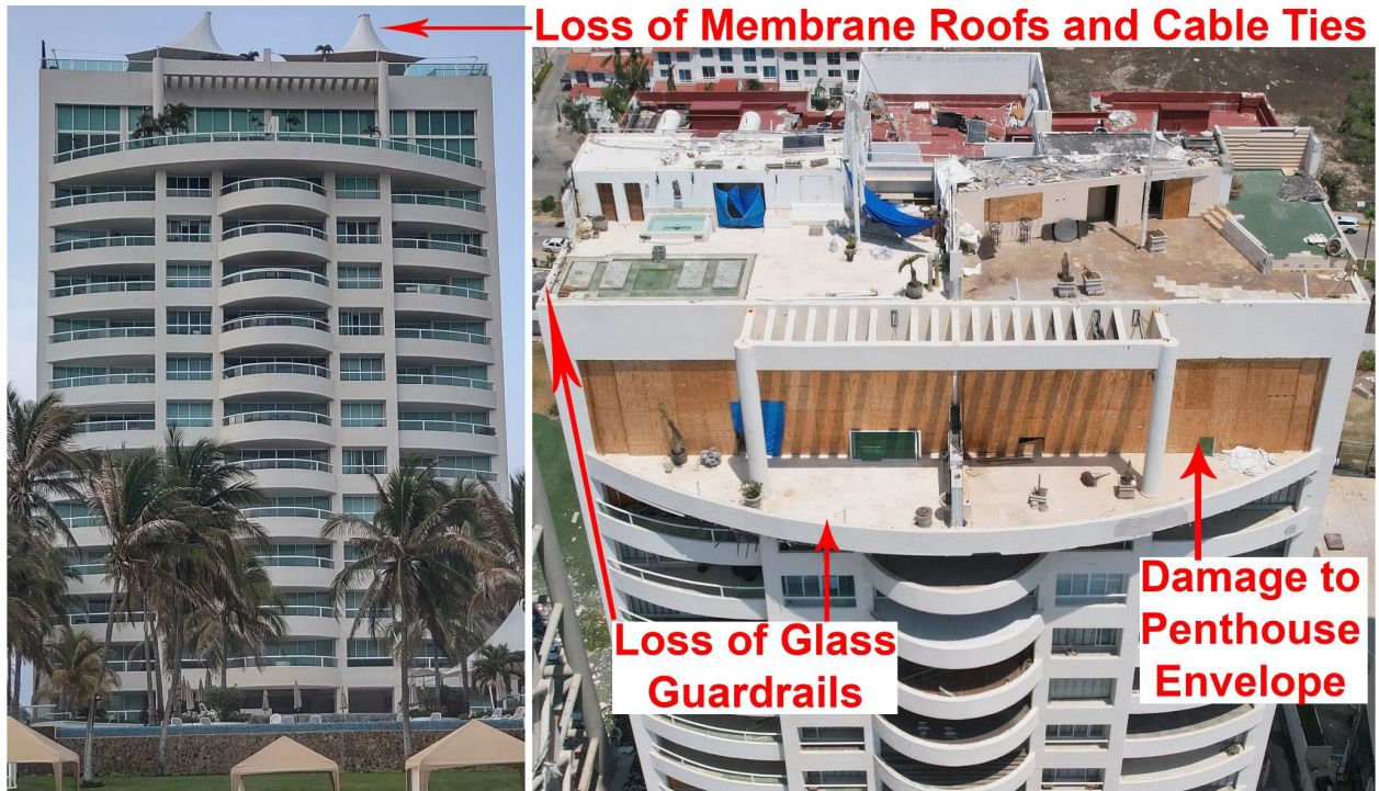
Figure 4.1.13. Torre Playa Diamante (Cluster 13) damage to penthouse and appendages, view of the SW, beachfront, elevation; (left) before Hurricane Otis (Source: Google Street View); after Hurricane Otis (Source: FAST).
