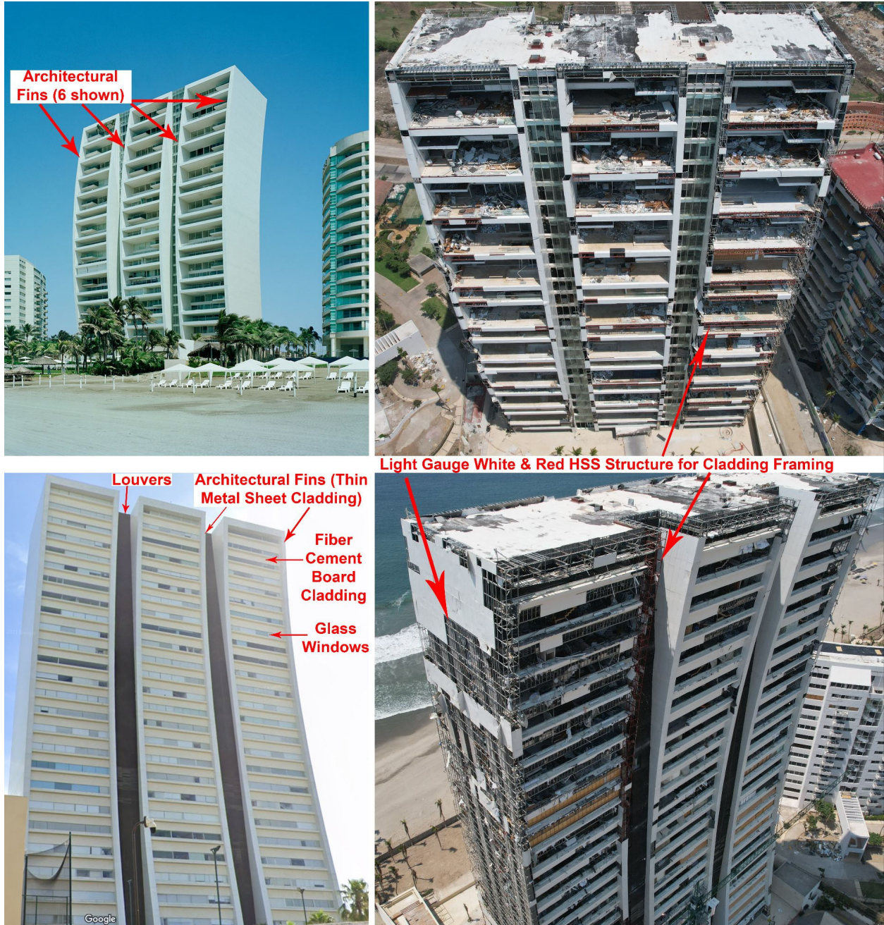
Figure 4.1.8. Marena (Cluster 15) seaward and landward elevations views; (top, left) before Hurricane Otis view of the seaward SW elevation (Source: Google Street View); (bottom, left) before Hurricane Otis view of the landward NE elevation (Source: Google Street View); (top, right) after Hurricane Otis view of the seaward SW elevation (Source: FAST); (bottom, right) after Hurricane Otis view of the landward NE elevation (Source: FAST).
