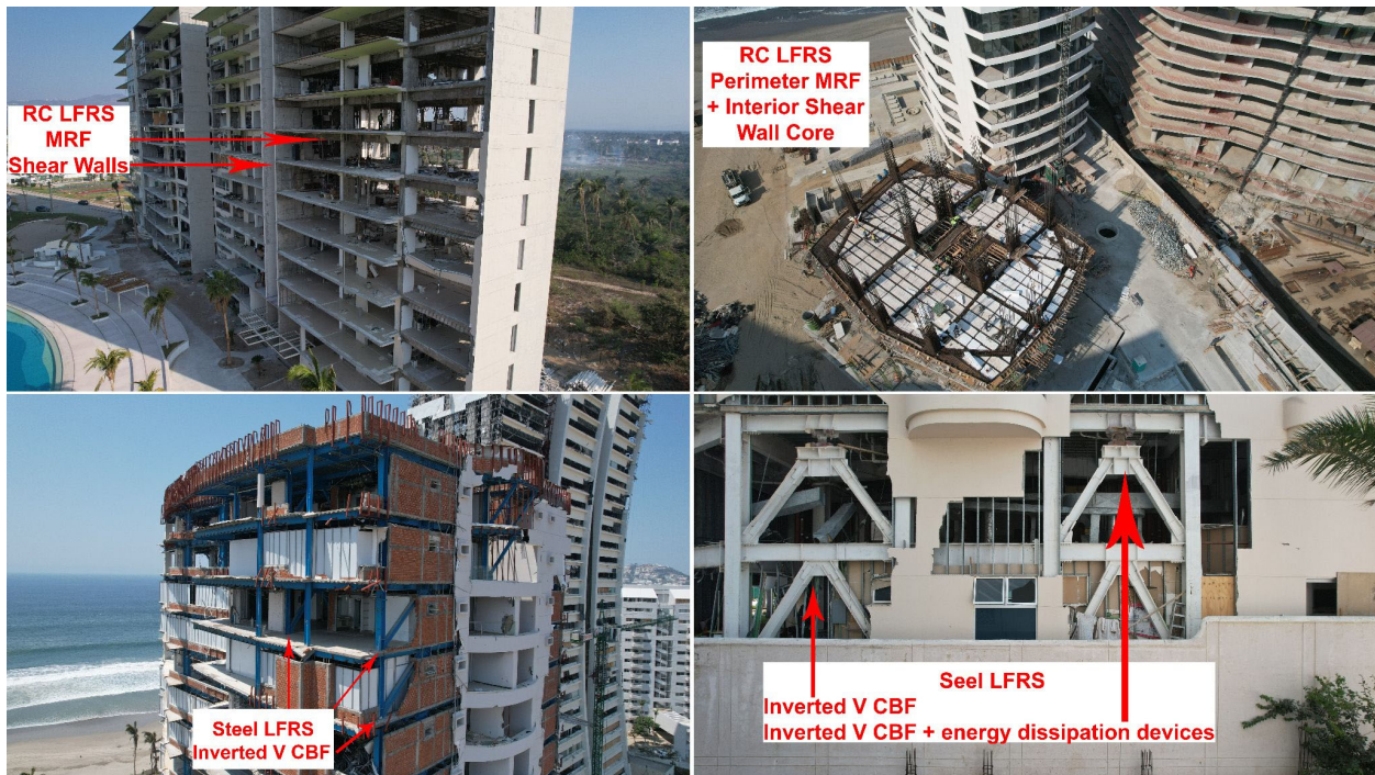
Figure 4.1.1. Examples of Reinforced Concrete (RC) and Structural Steel LFRS in Acapulco (Source: FAST).
