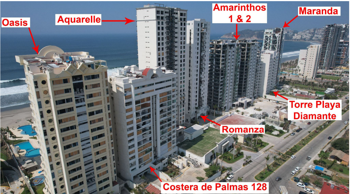
Figure 4.1.5. Cluster 13 NE elevation landward views; (top) before Hurricane Otis (Source: Google Street View) & (bottom) post Hurricane Otis (Source: FAST).
