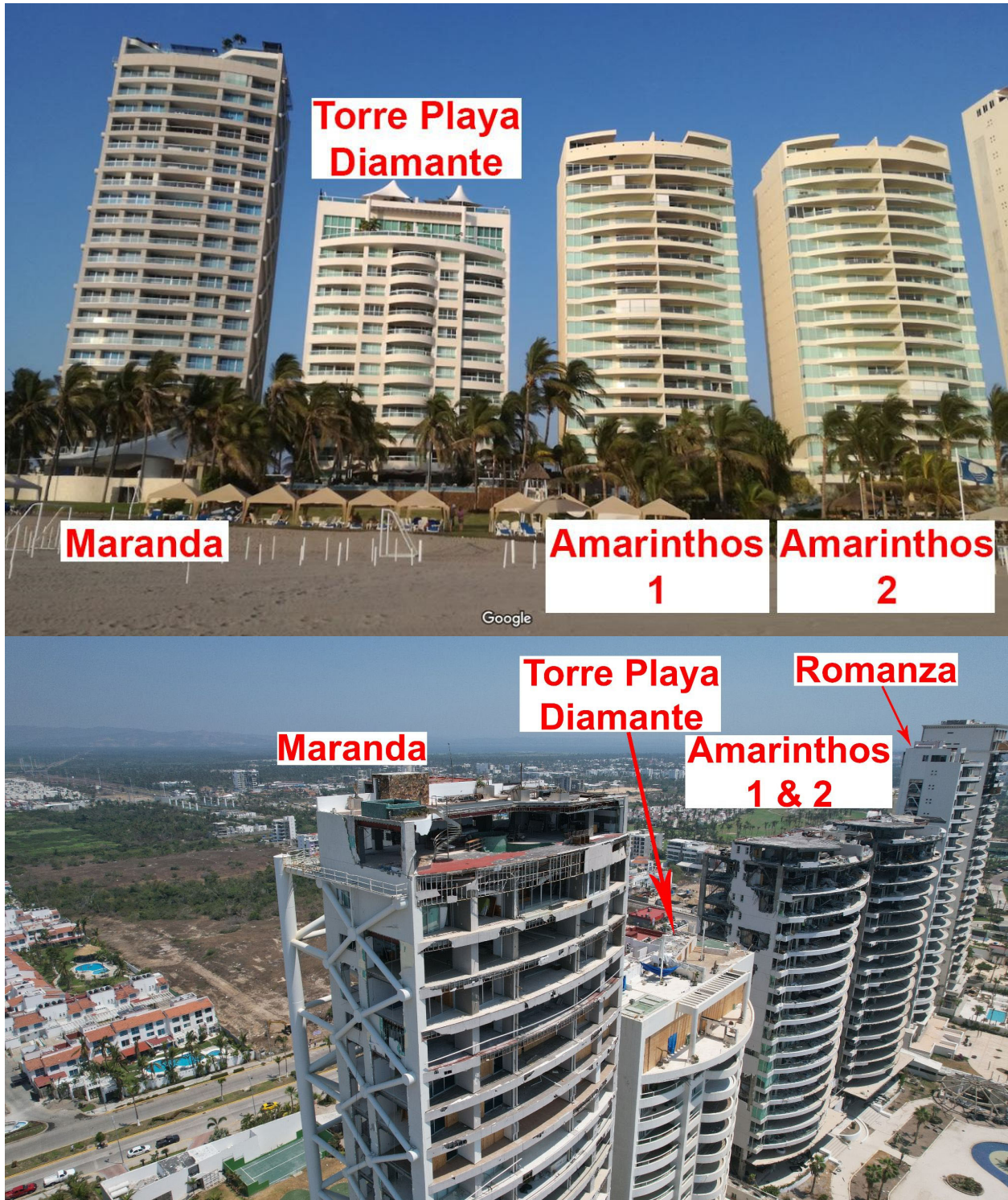
Figure 4.1.6. Cluster 13 SW elevation seaward views; (top) before (Source: Google Street View); (bottom) after Hurricane Otis (Source: FAST).
